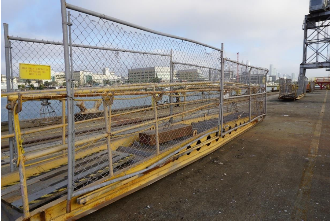
30 Ft. Gangway (Wharf 3)
