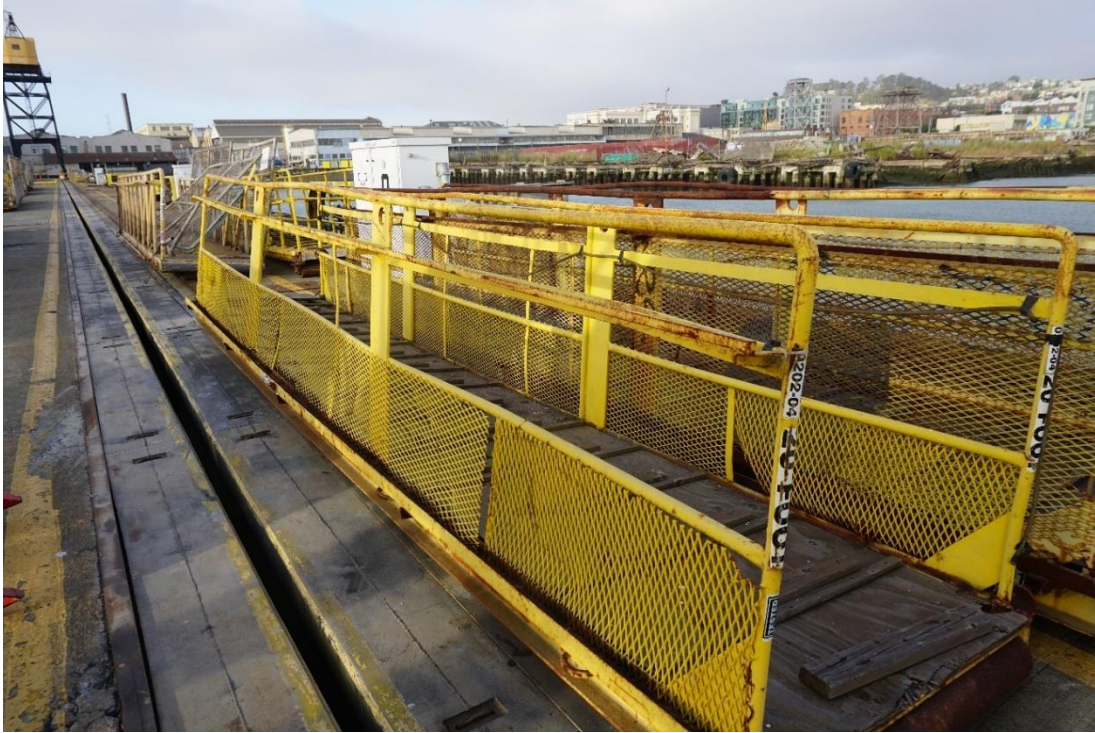
20 Ft. Gangway (Wharf 3)
