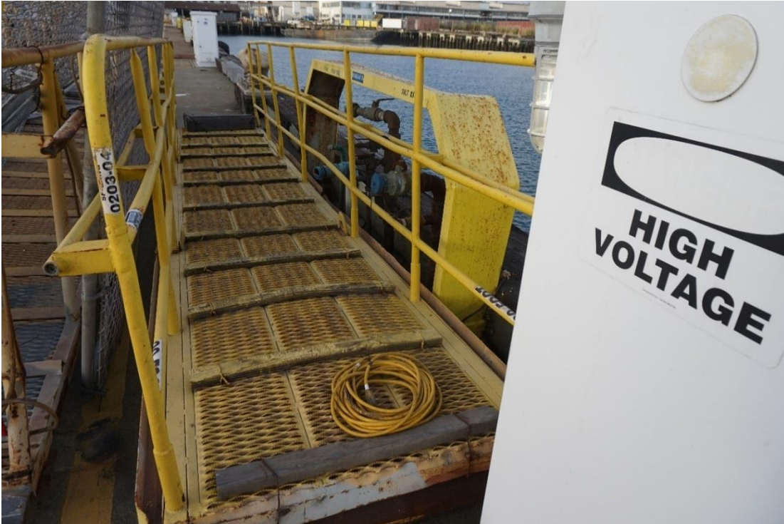
20 Ft. Gangway (Wharf 3)
