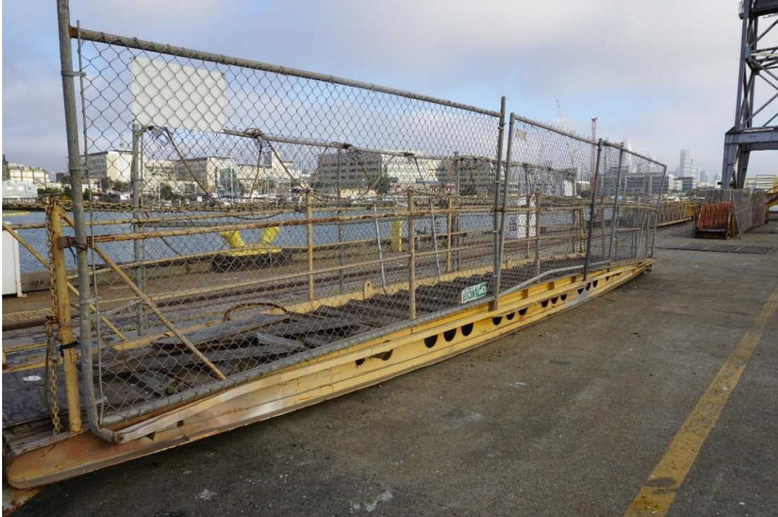
35 Ft. Gangway (Wharf 3)
