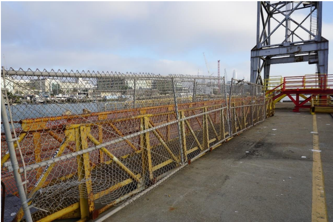
50 Ft. Gangway (Wharf 3)
