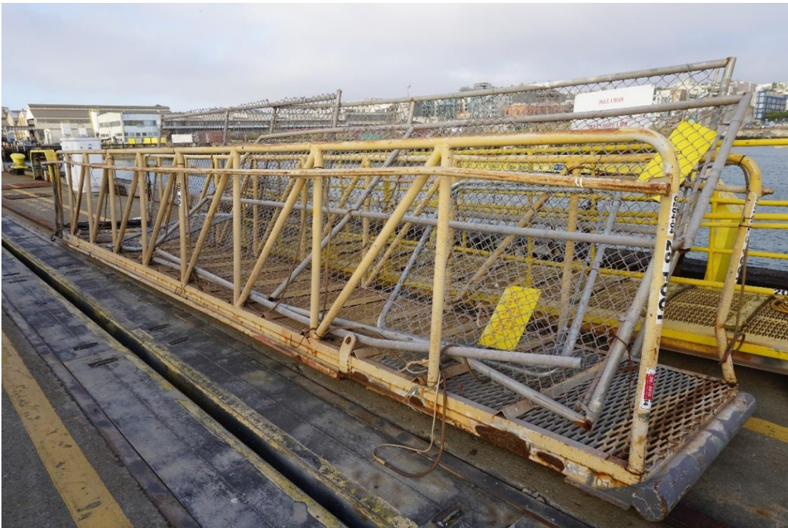
28 Ft. Gangway (Wharf 3)
