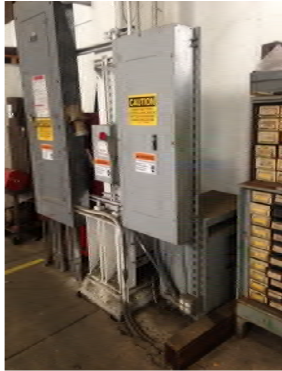
Figure 23. Interior panel boards & dry type transformer
