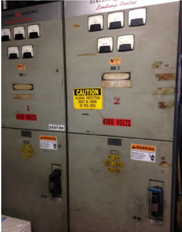
Figure 28. 4160V switchboard
