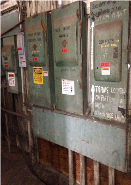
Figure 30. 400A 480V power distribution system
