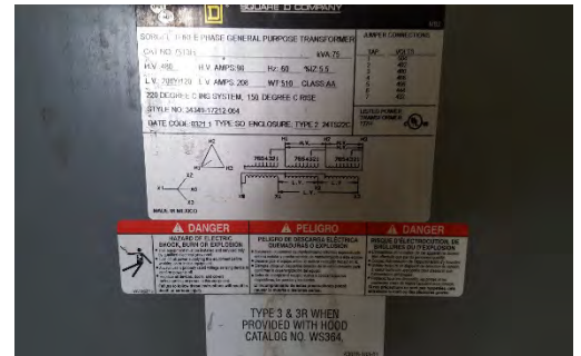
Figure 45. 75 KVA transformer
