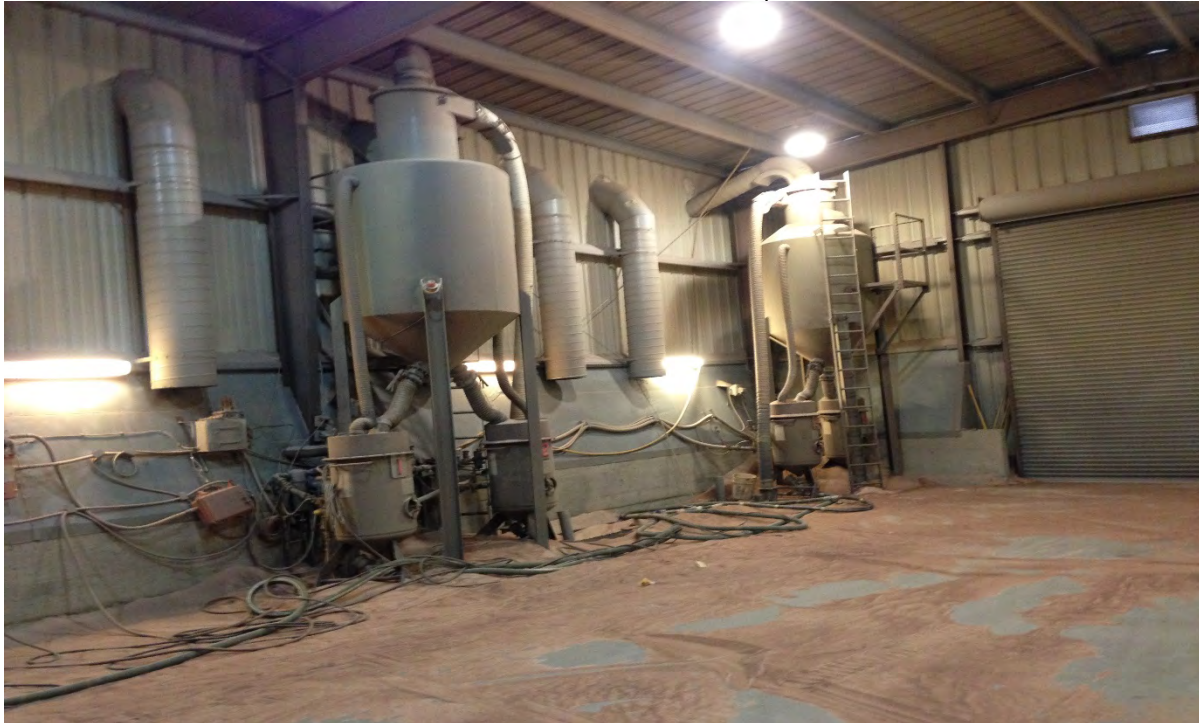
Figure 46. Interior of building 251
