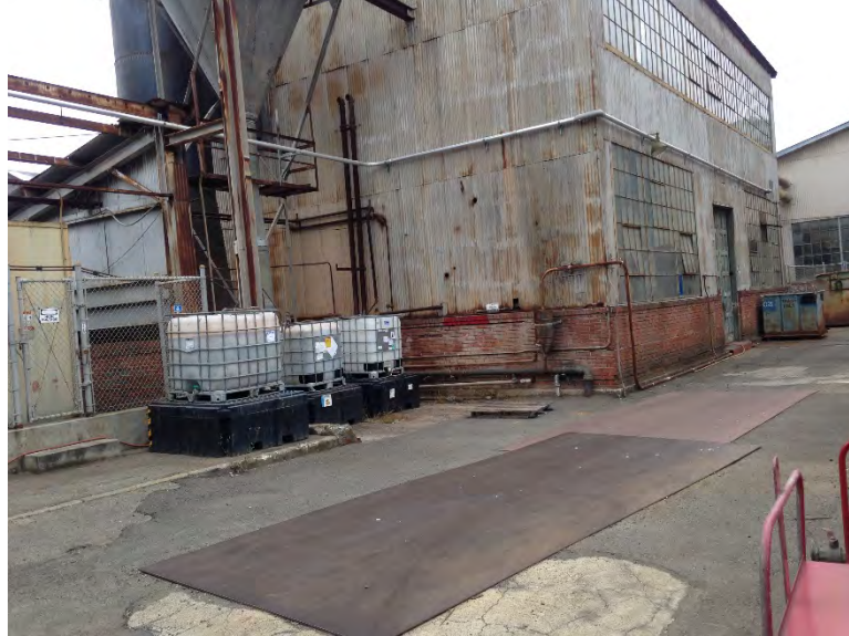
Figure 6. exterior of Substation #11
