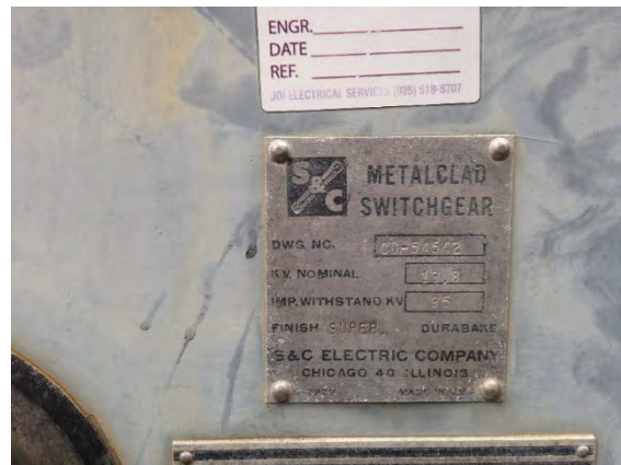
Figure 8. switchgear nameplate
