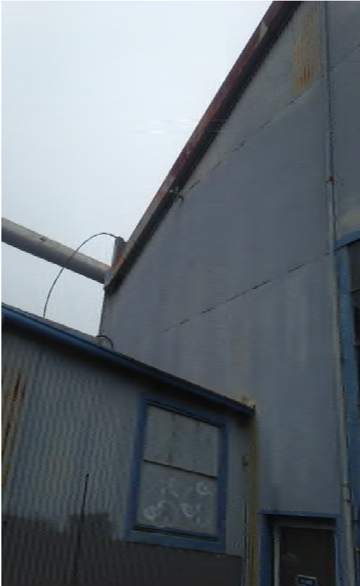
Figure 26. Overhead PG&E cut line
