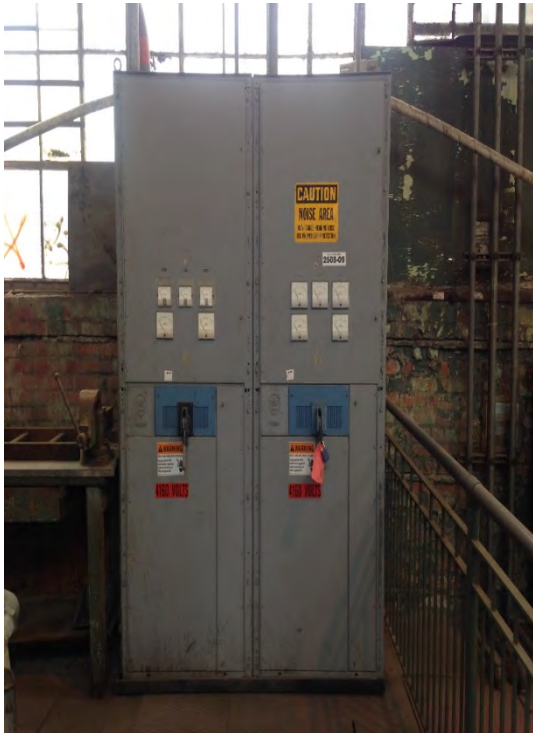
Figure 10. 4160V switchboard
