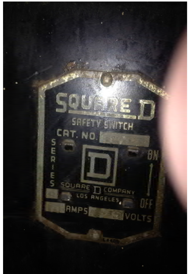
Figure 39. Power and lighting panel
