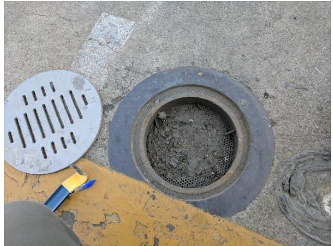
Figure 9. Wharf-side Drain Inlet with Screen
