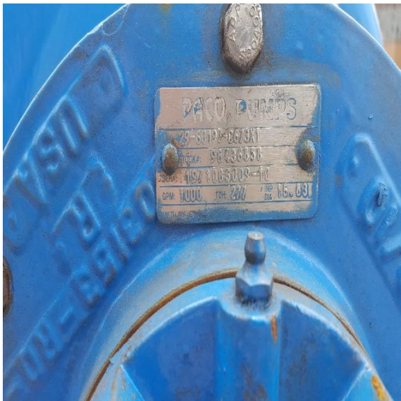
Figure 31. 75 HP Fresh Water Booster Pump Nameplate (2 Pictures)
