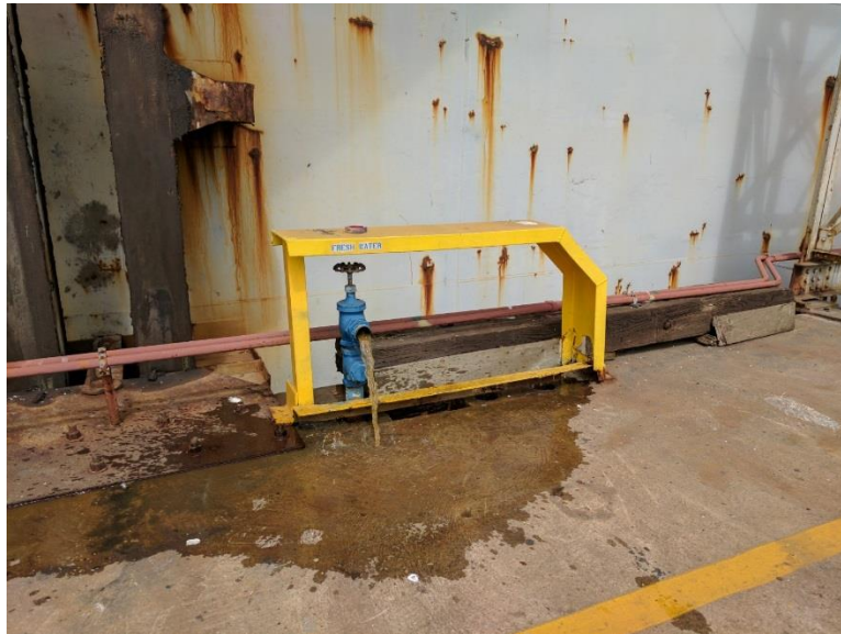
Figure 25. Opened Fresh Water Riser Pier 4
