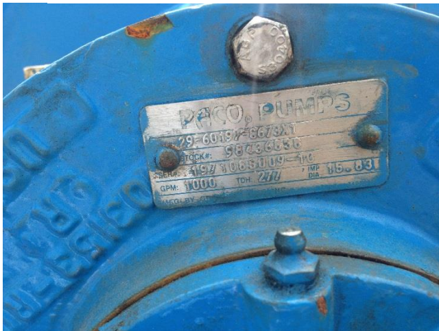
Figure 32. 250 HP Pier 3 Salt Water Pump (P3SWP) Nameplates (2 Pictures)
