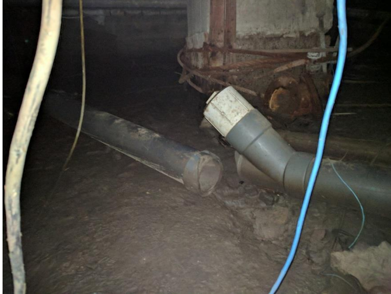
Figure 18. Storm Drain Outfall Bldg 111
