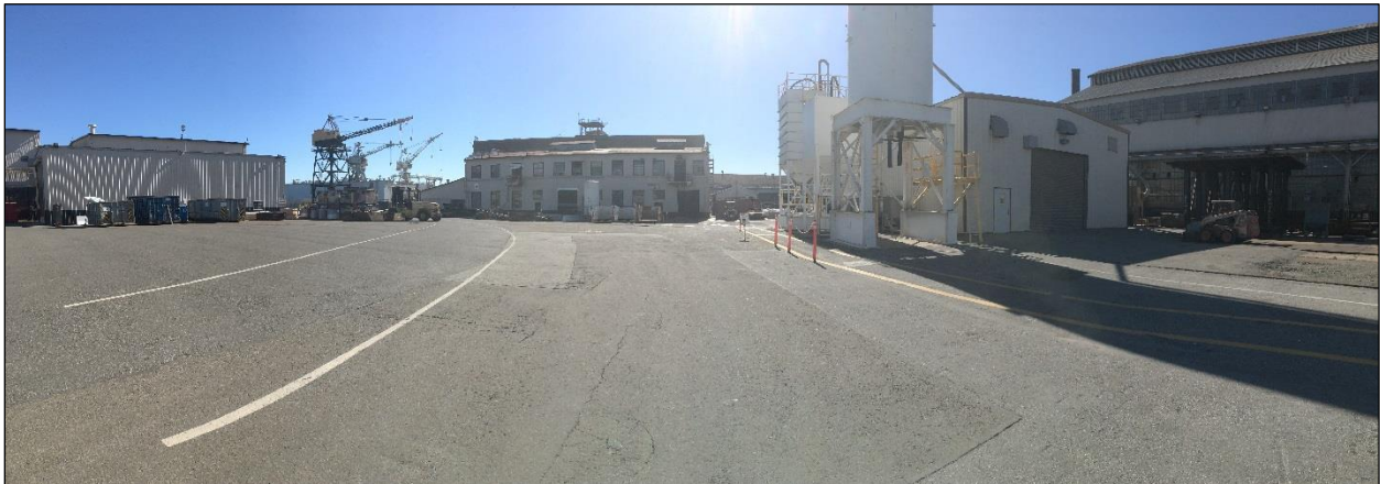
Figure 1. Pier 68-70 viewed from Admin Offices
