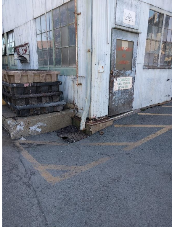
Figure 11. Disconnected Roof Downspout w/ Plugged Inlet Figure 12. Disconnected Roof Downspout
