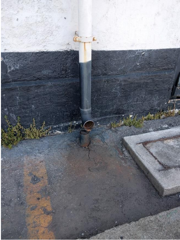
Figure 11. Disconnected Roof Downspout w/ Plugged Inlet Figure 12. Disconnected Roof Downspout
