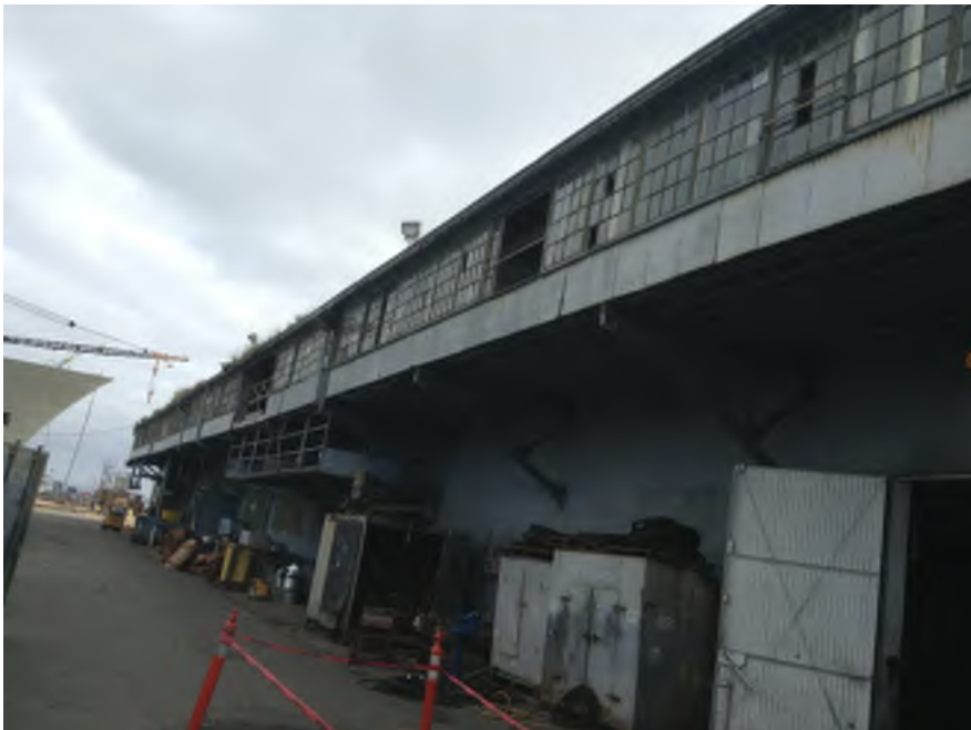
Fig. 2 – Building 109 viewed from northwest corner.
