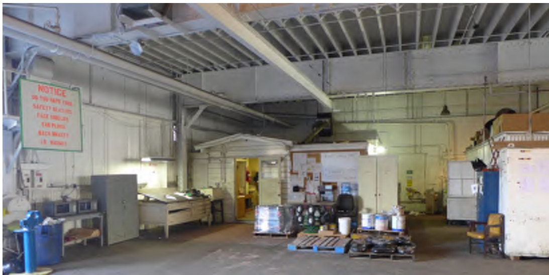
Figure 16 - Building 109, Interior of plate shop, facing east.
