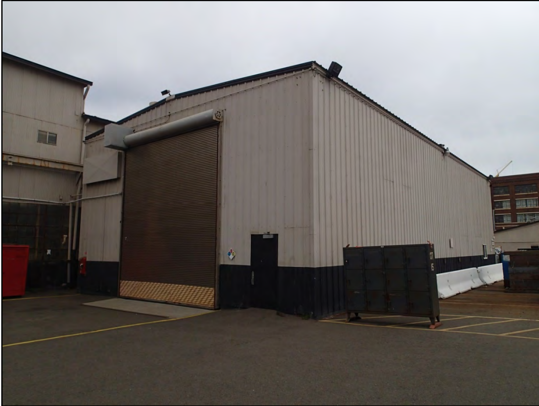
Figure 250-2 - Overall southwest view of Building 250.
