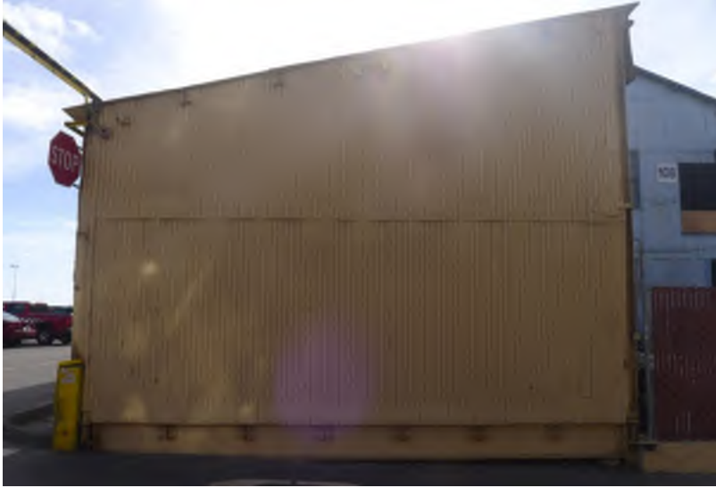
Figure 3 - Building 120: West Elevation
