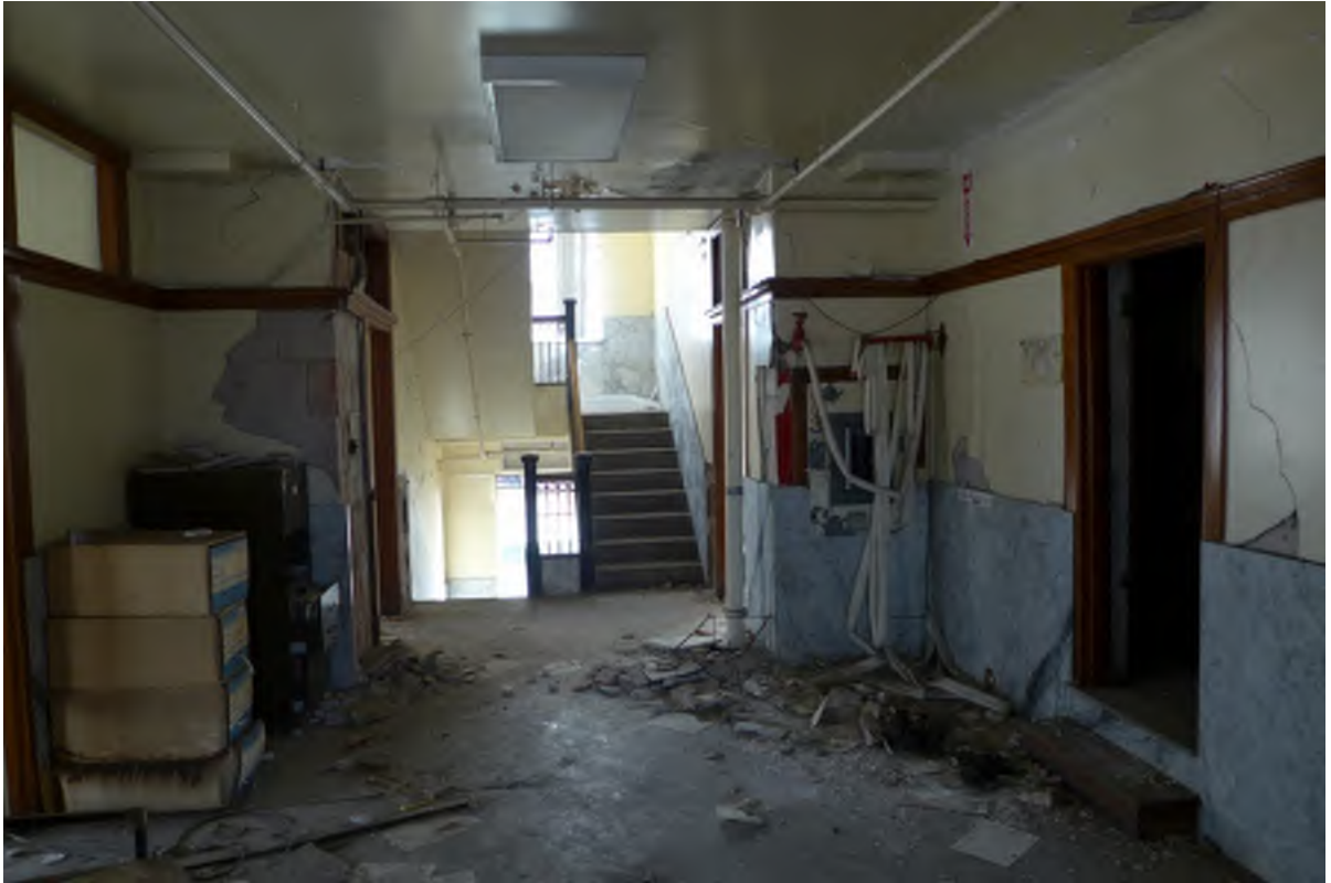
Figure 20 - Building 111, mezzanine facing west
