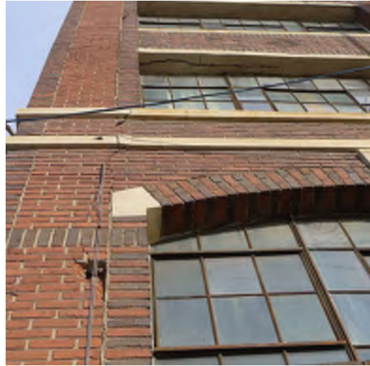
Figure 9 – Cracking, south elevation
