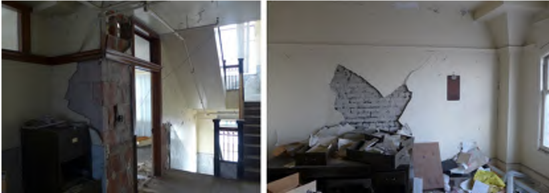
Figure 27 - Building 111, mezzanine lobby and office walls
