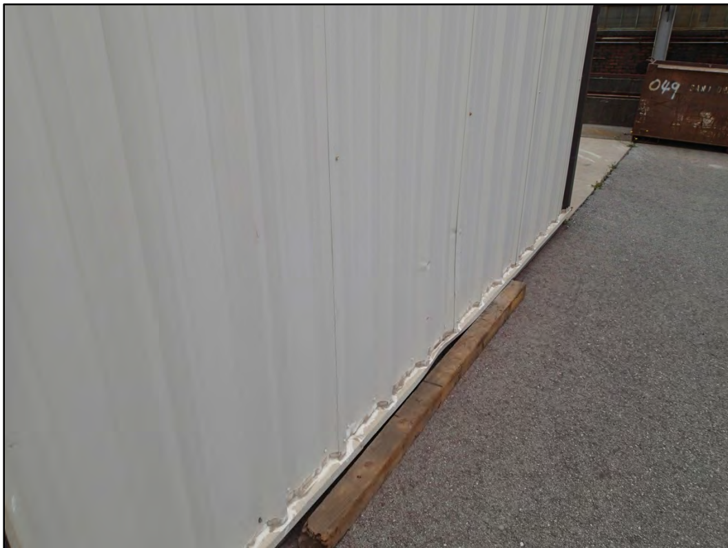
Figure 251-3 – View of the typical condition of the corrugated metal panels at Building 251.
