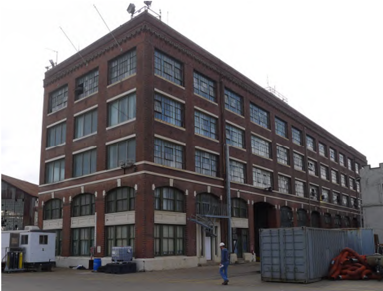
Figure 1 - Building 111, view from the northwest
