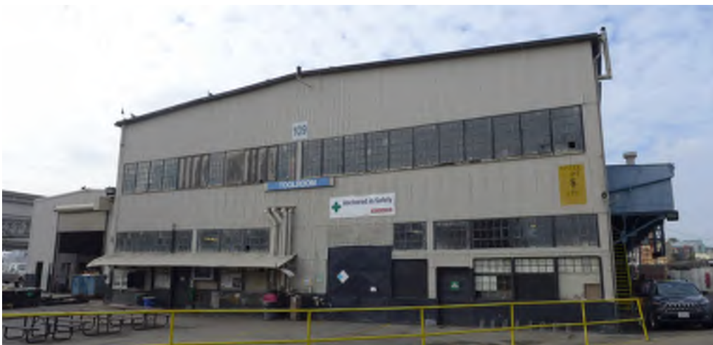
Figure 10 - Building 109, Tool Room east elevation..
