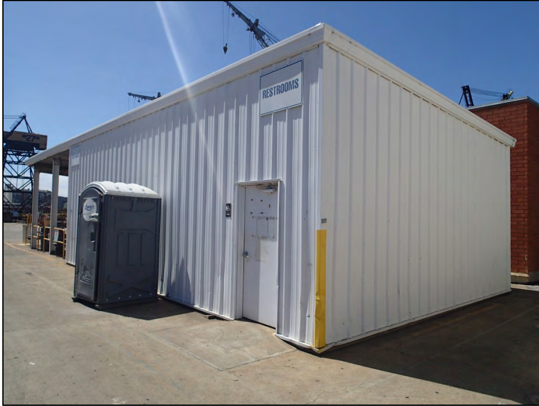
Figure 143-2 - Overall southeast view of Building 143.
