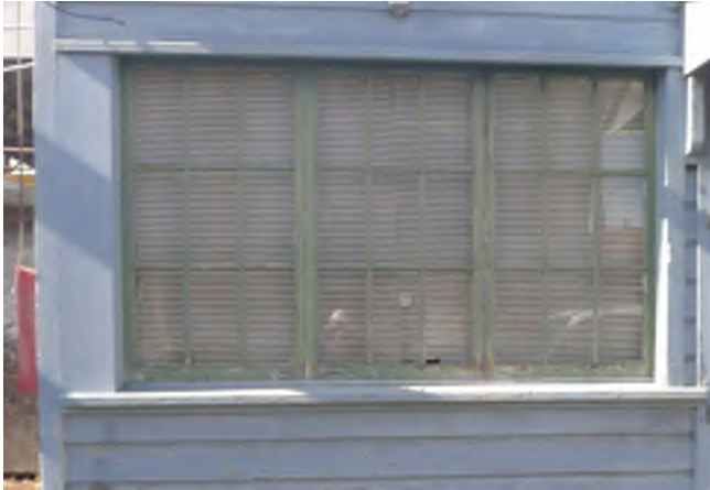
Figure 4 - Building 121: Windows at east elevation
