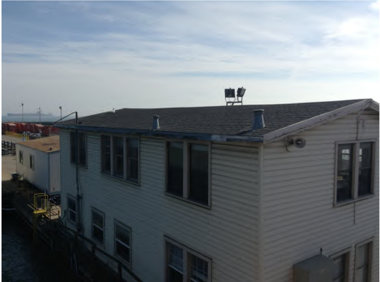
Fig. 1 - Building 127 view from bldg 68 roof top
