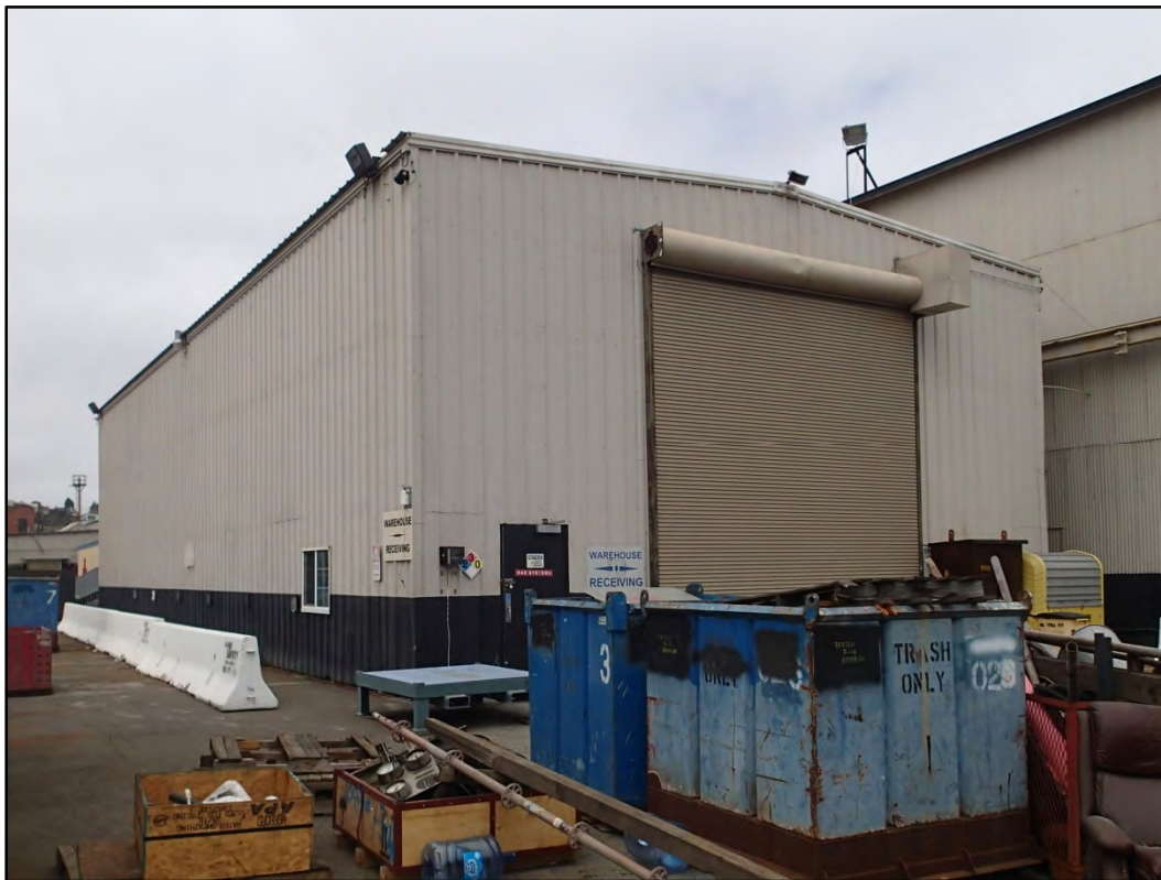
Figure 250-1 - Overall southeast view of Building 250.
