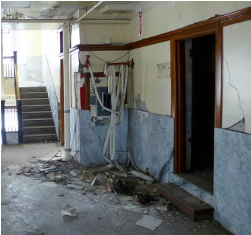
Figure 28 - Building 111, mezzanine lobby and office walls, marble wainscot
