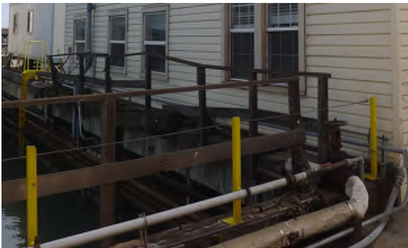
Figure 10 - Pipe chase and wood railings
