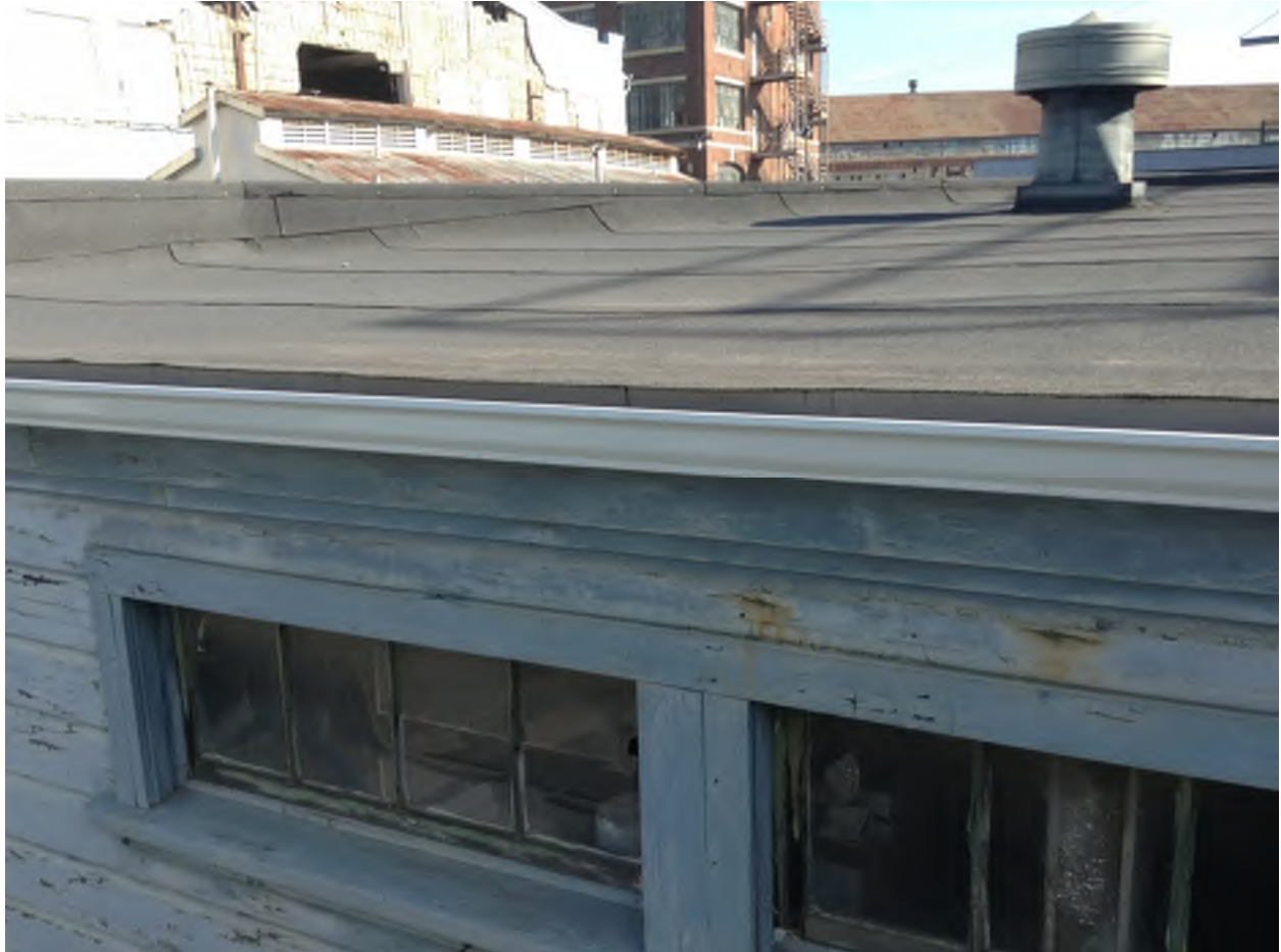
Fig. 1 - Building 121 view from adjacent mens restroom
