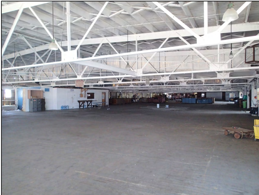
Figure 109-9 – Overall interior view of Building 109 Mold Loft.
