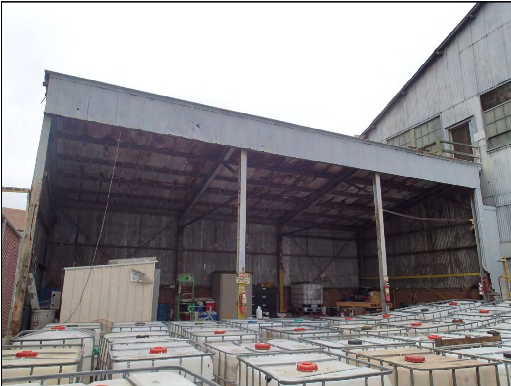
Figure 120-1 - Overall west view of Building 120.
