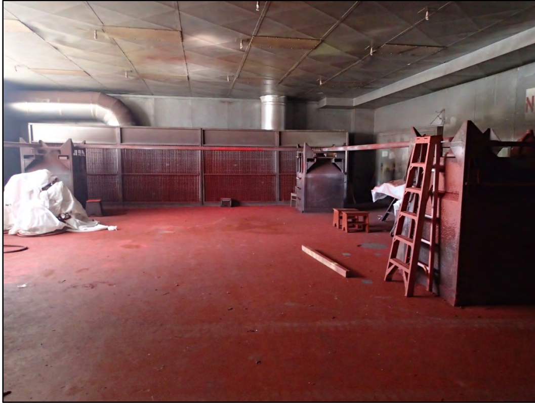
Figure 109-8 – Overall interior view of Building 109 Paint Shop booth.
