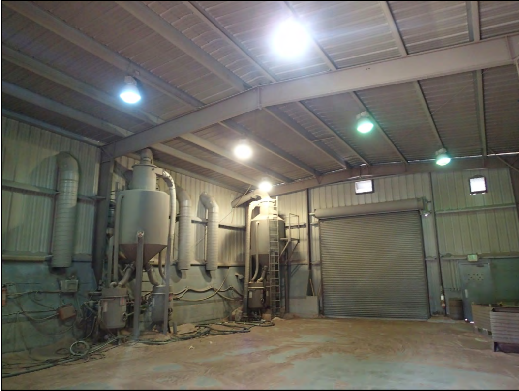
Figure 251-7 - Overall interior view of Building 251 looking southwest.
