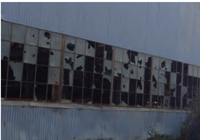
Figure 5 - Building 109, steel windows
