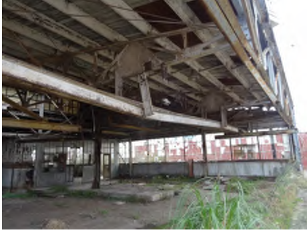
Figure 5 – Typical condition of west half of building 109
