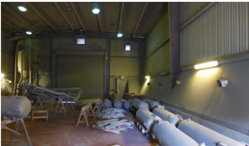
Figure. 4 - Building 250: Interior, facing west.
