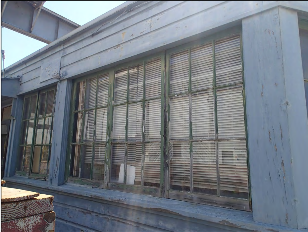
Figure 121-5 – Typical view of wood windows at Building 121.
