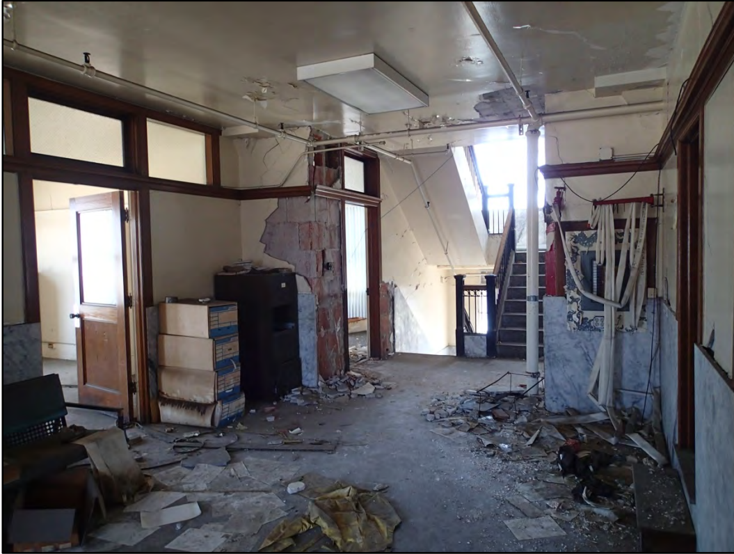
Figure 111-9 – View of second floor interior at the north end of Building 111
