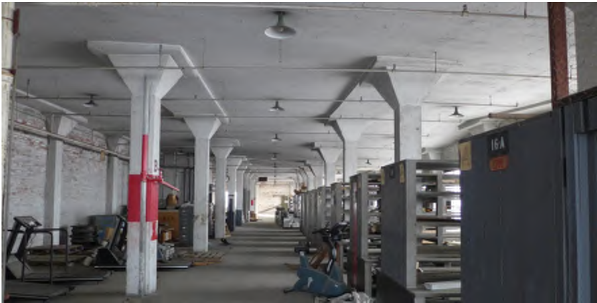
Figure 23 - Building 111, fourth floor facing south
