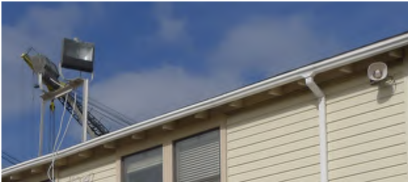
Figure 9 - Roof mounted flood lights and speakers
