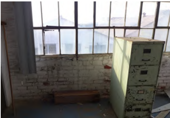
Figure 30 - Building 111, third floor exterior wall.
