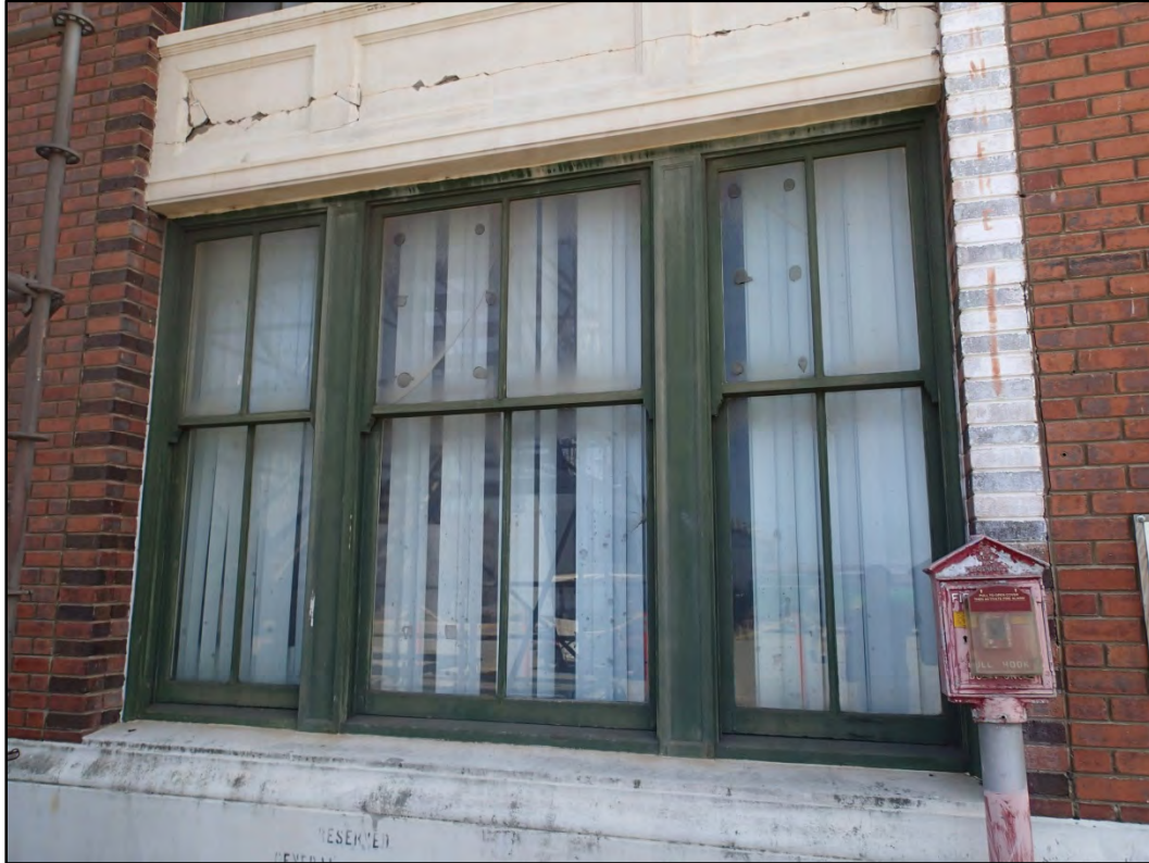
Figure 111-4 – Typical view of Building 111 wood windows.
