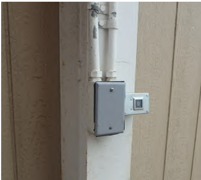
Figure 143-2 – Exterior Lighting Photosensor Controls
