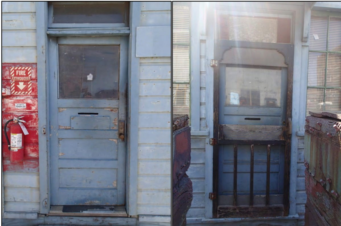
Figure 121-3 and Figure 121-4 – Typical view of the wood doors at Building 121.
