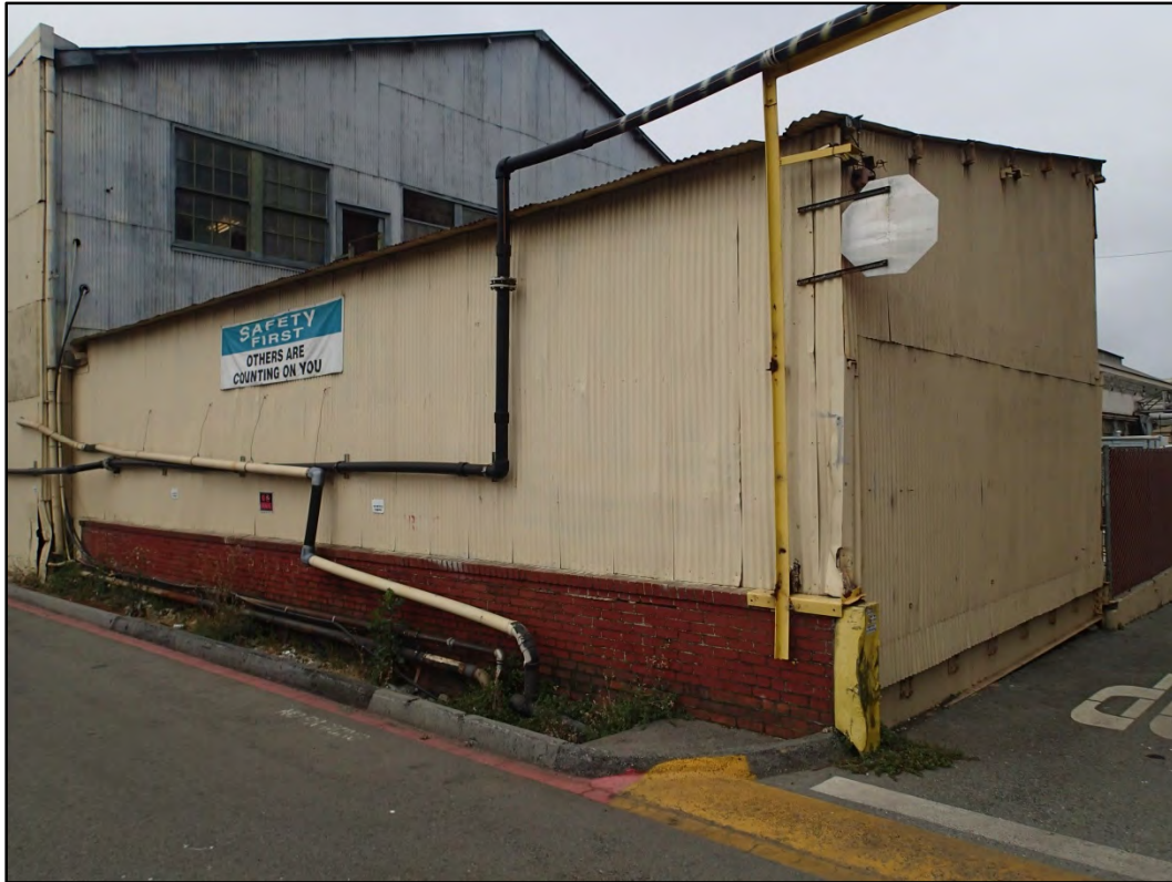
Figure 120-2 – Overall northeast view of Building 120.
