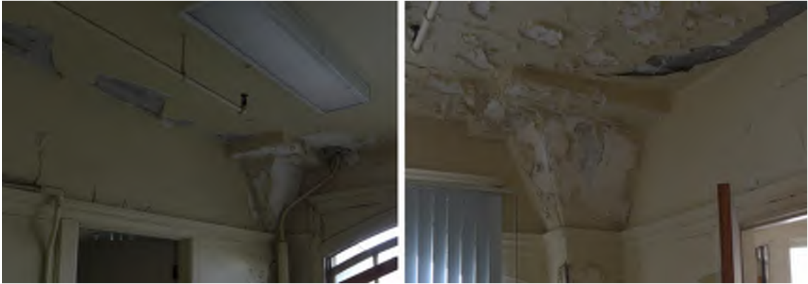
Figure 33 - Building 111, mezzanine floor ceiling
