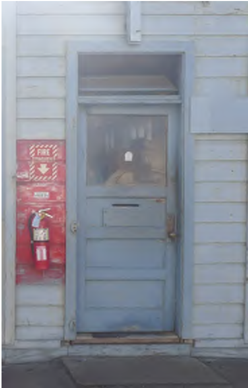
Figure 6 - Building 19: Personnel door at north elevation
