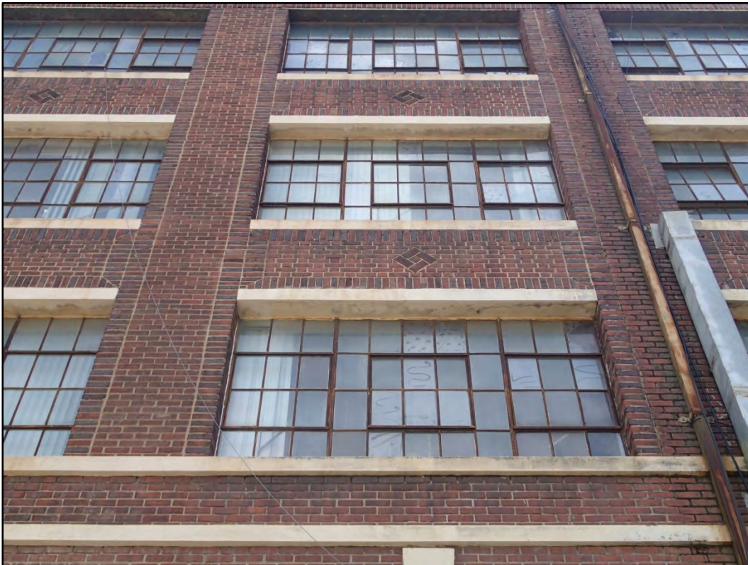
Figure 111-3 – Typical view of Building 111 steel sash windows.
