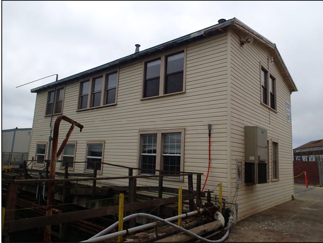
Figure 127-2 - Overall northwest view of Building 127.
