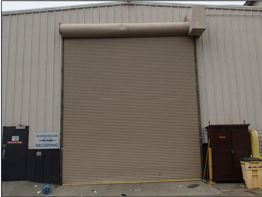
Figure 250-4 – View of steel roll-up door at Building 250.
