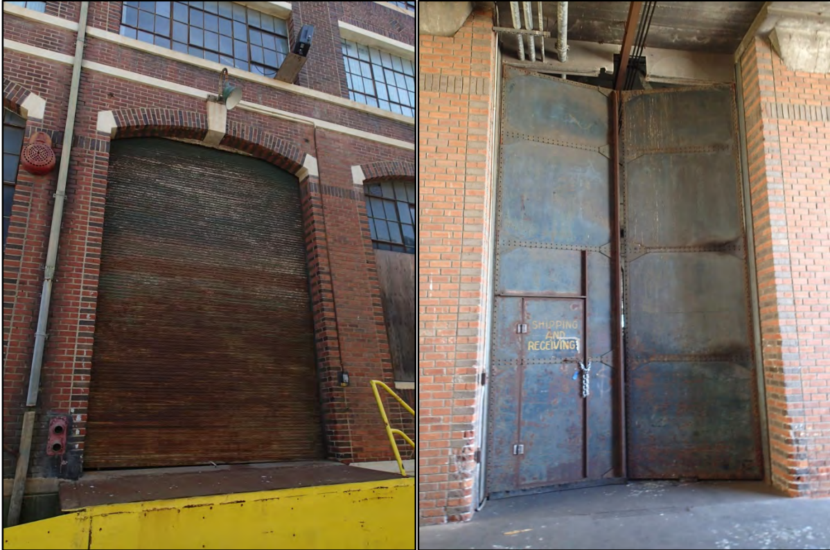
Figure 111-6 and Figure 111-7 – Typical view of Building 111 steel roll-up and double doors.
