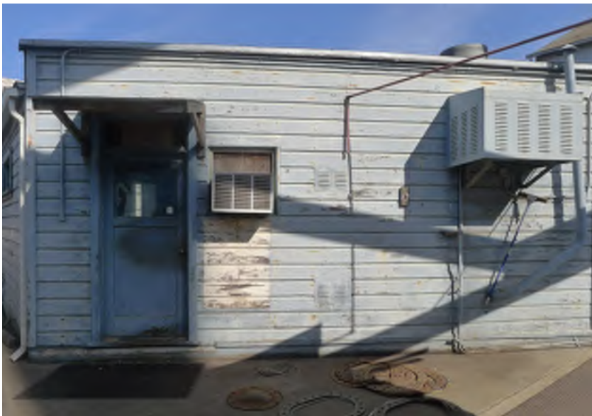
Figure 3 - Building 121: South Elevation
