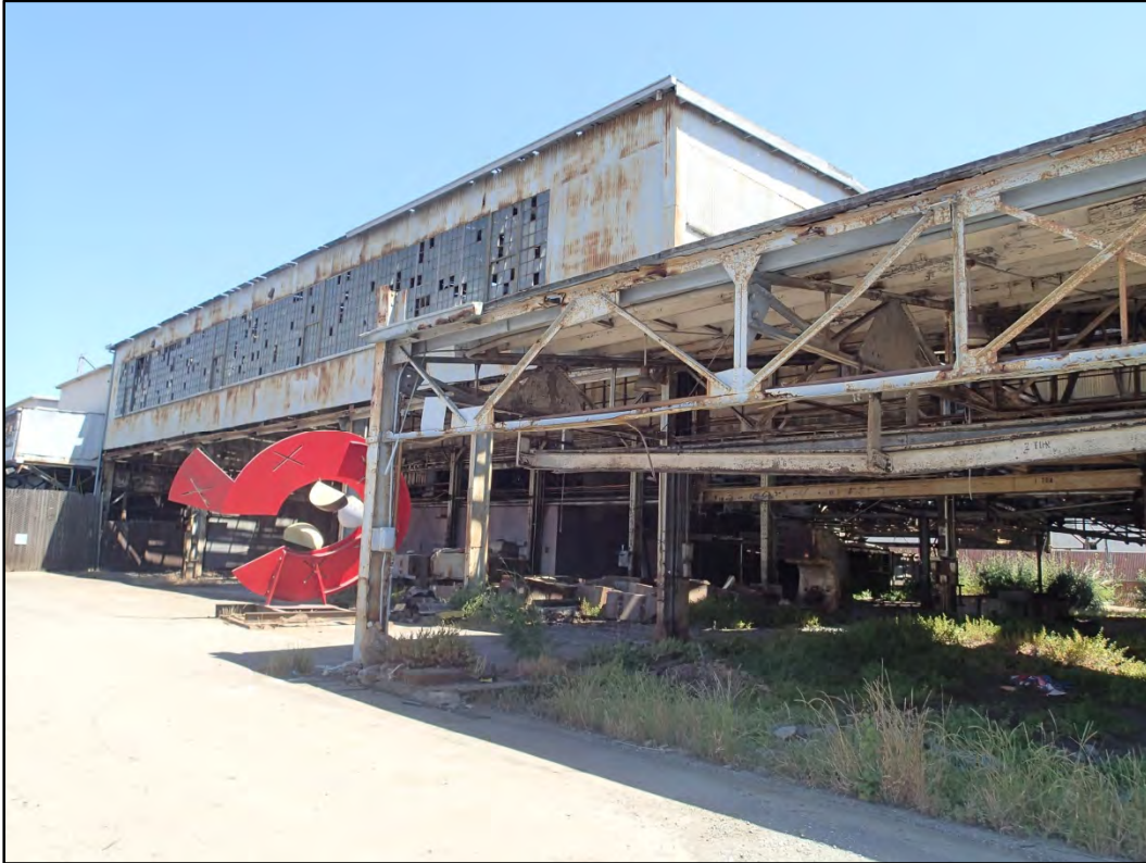
Figure 109-10 – Overall northwest view of the abandoned west section of Building 109.
