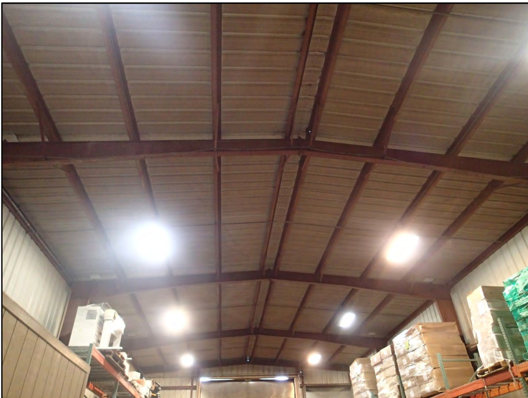
Figure 250-7 - View of Building 250 roof structure and corrugated metal panels.
