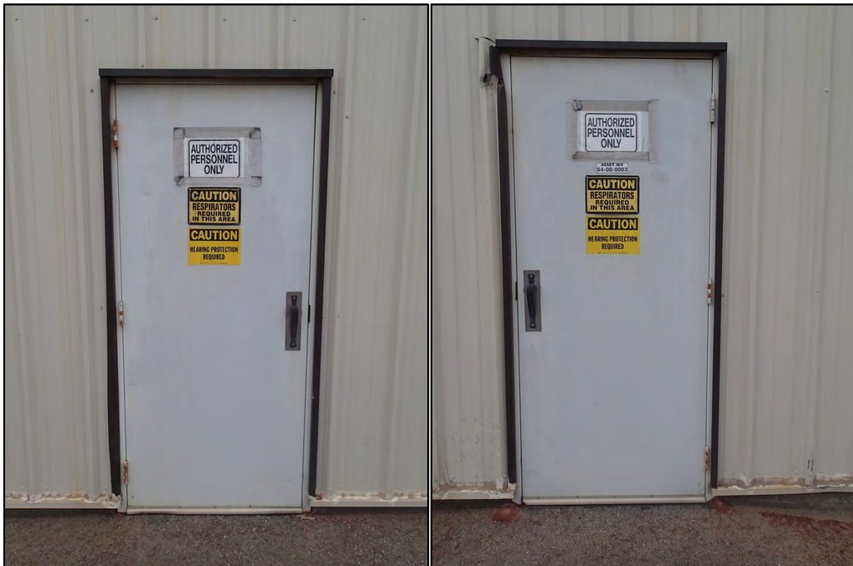
Figure 251-5 and Figure 251-6 – View two hollow metal doors at Building 251.
