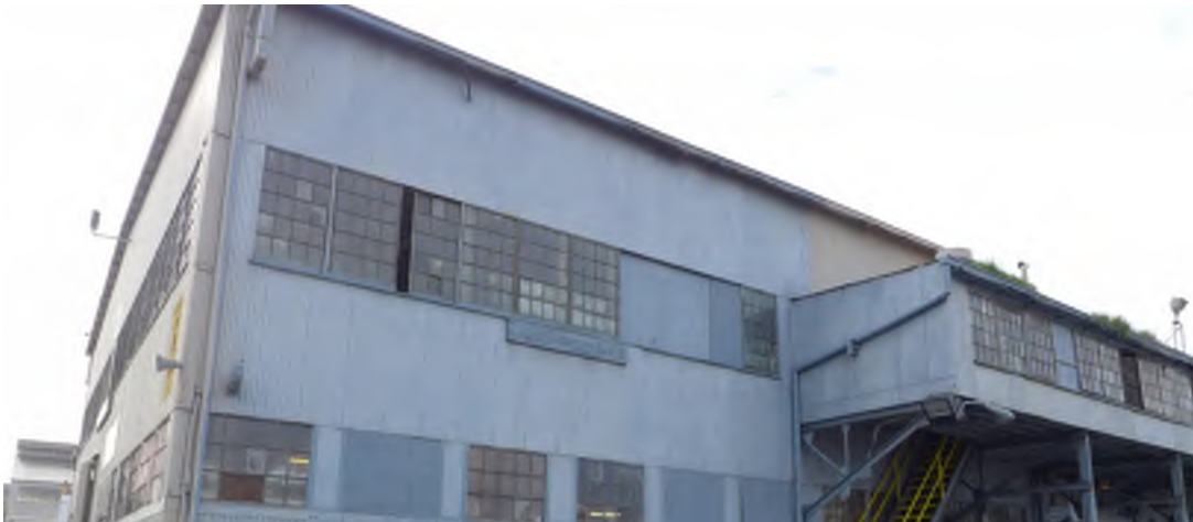
Figure 20 - Building 109, Mold loft north elevation.
