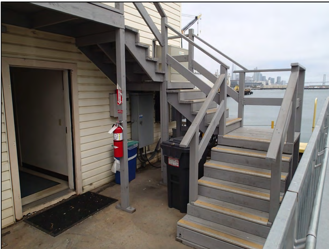
Figure 127-6 - Overall southeast view of Building 127.
