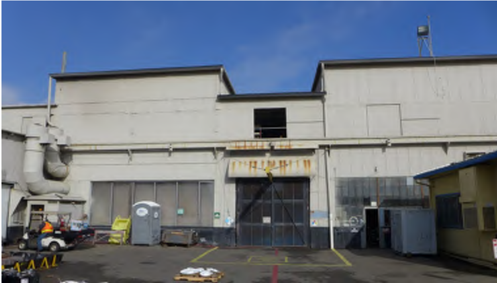
Figure 9 - Building 109, Paint Shop south wall.
