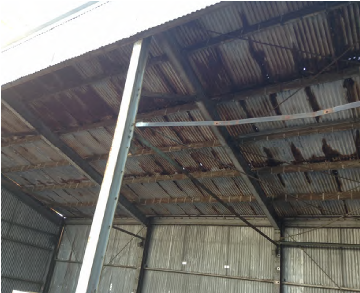
Fig. 1 - Building 120 view from Bldg. 108 2 nd floor
