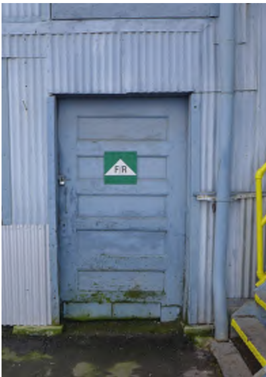
Figure 16 - Building 109, Wood panel door at north wall of Tool Room.
