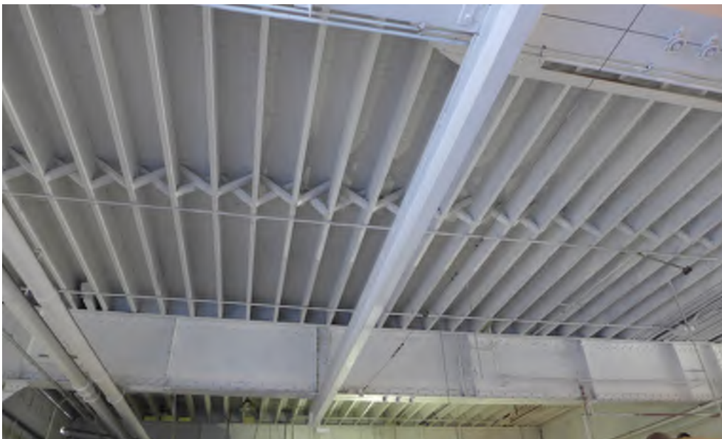
Figure 18 - Building 109, Paint shop ceiling.
