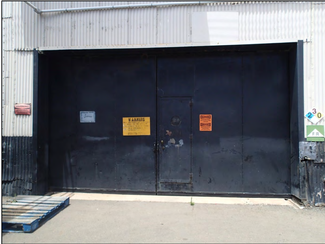
Figure 109-4 - South view of Building 109 Plate Shop metal sliding doors.
