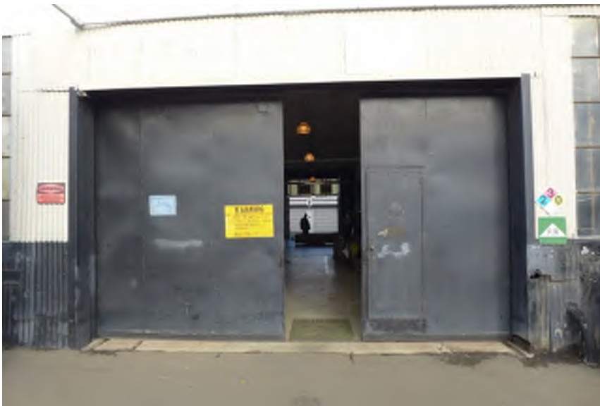
Figure 14 - Building 109, Plate shop metal sliding doors at north wall.
