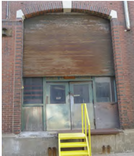
Figure 16 - Wood loading doors, west elevation
