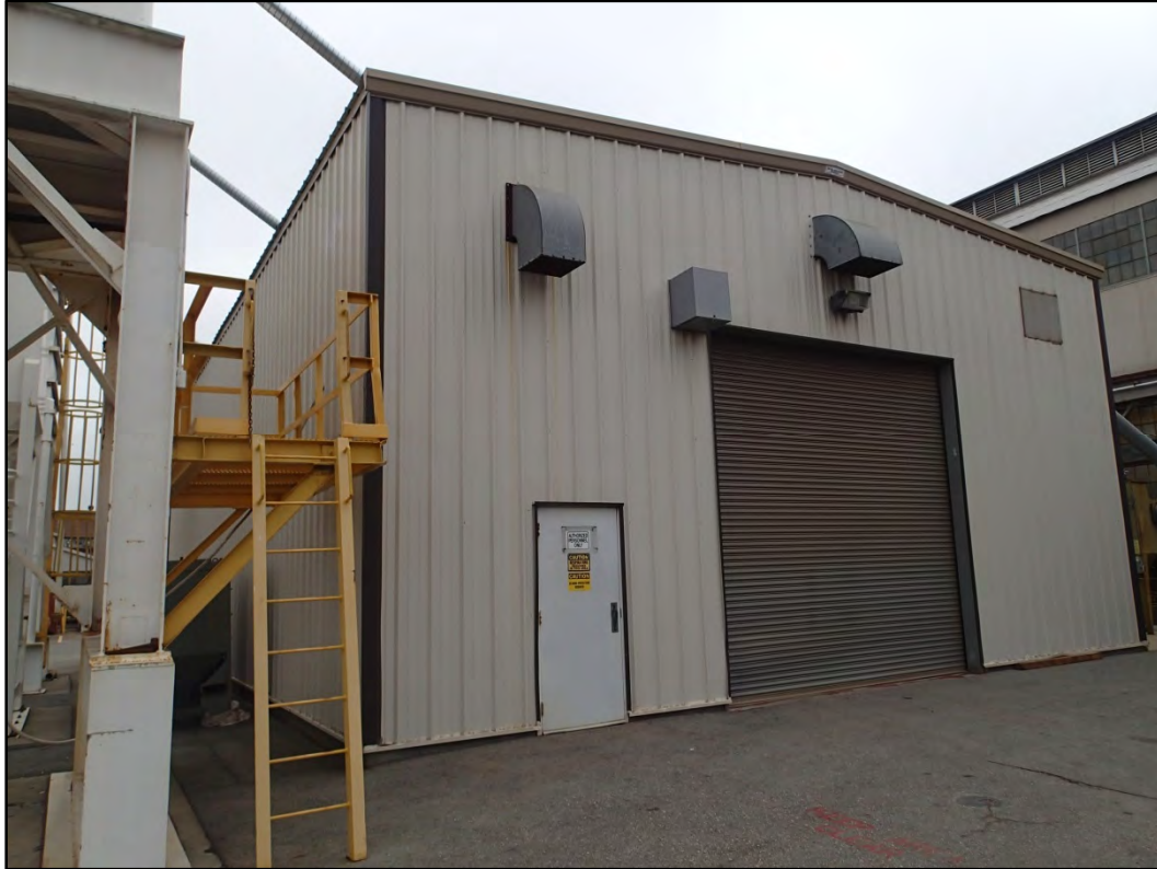
Figure 251-2 - Overall northwest view of Building 251.
