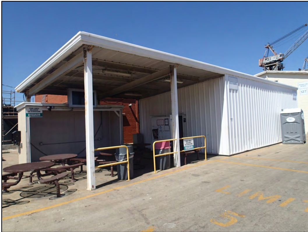
Figure 143-1 - Overall southwest view of Building 143.
