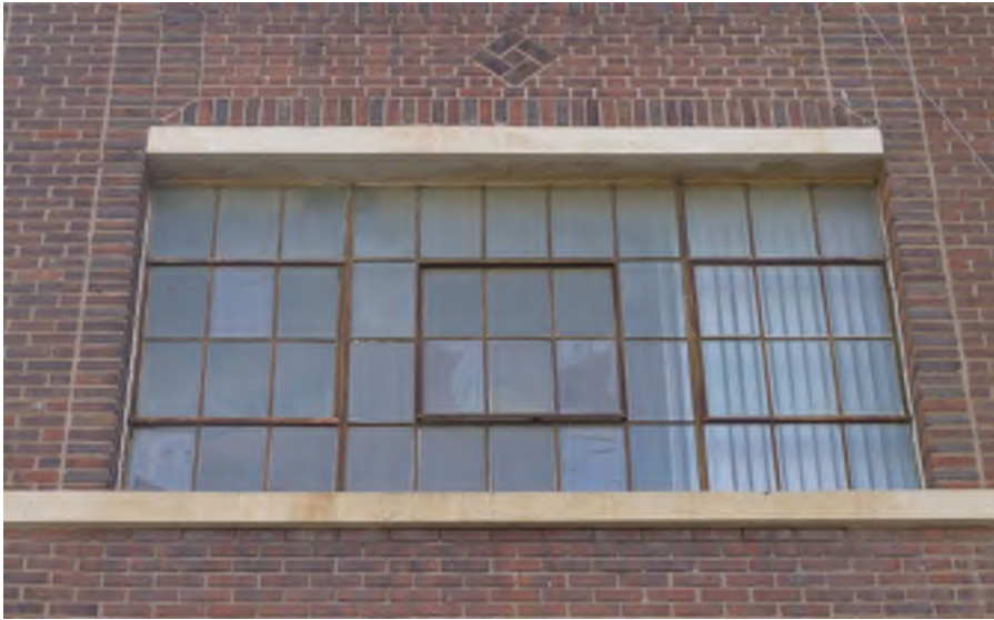
Figure 12 – Typical steel window, west elevation
