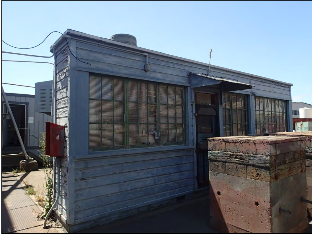
Figure 121-2 - Overall southeast view of Building 121.
