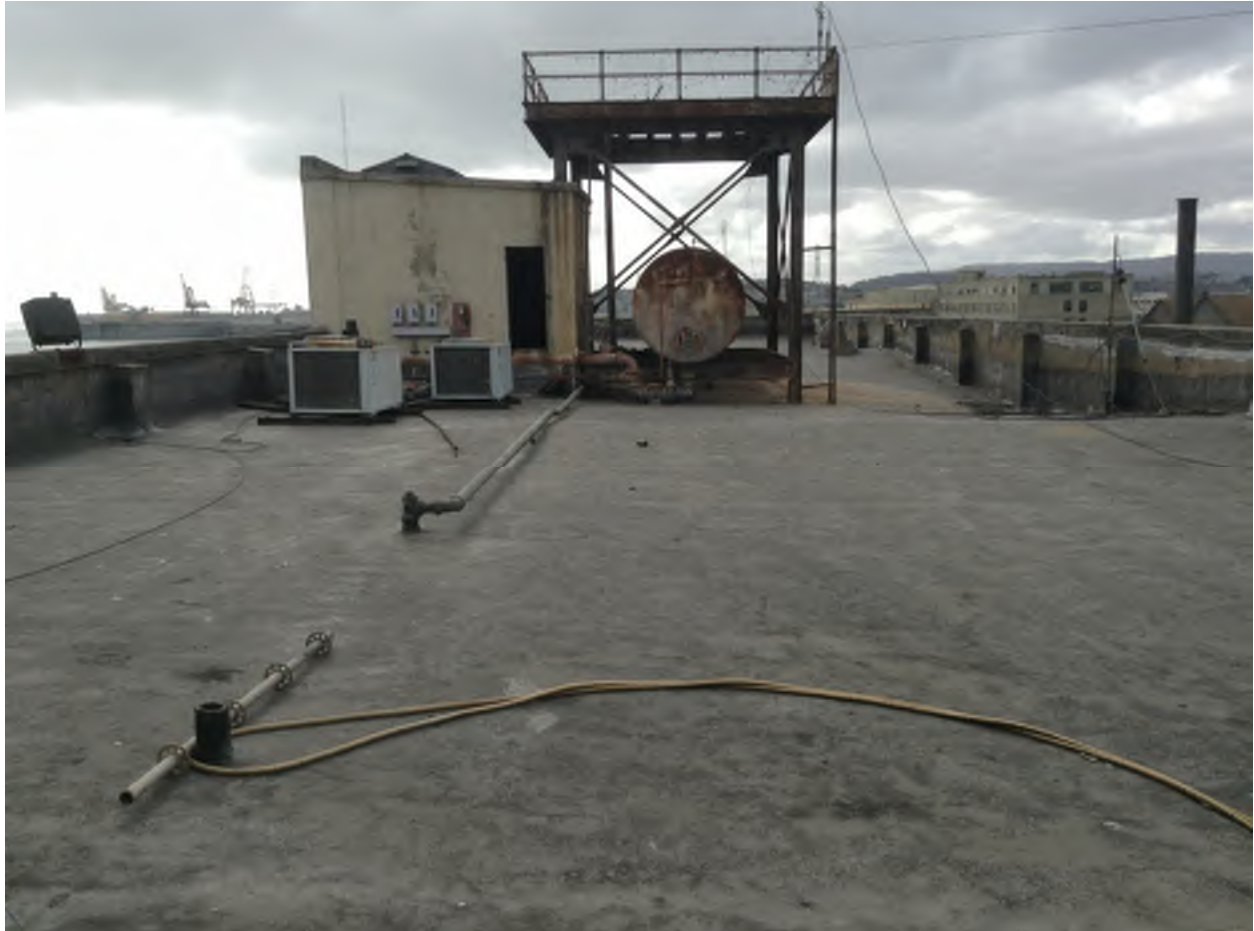
Fig. 1 - Building 111 viewed from roof
