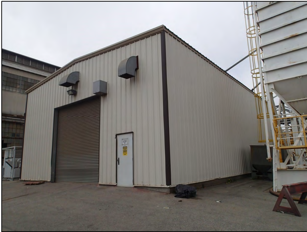
Figure 251-1 - Overall northeast view of Building 251.
