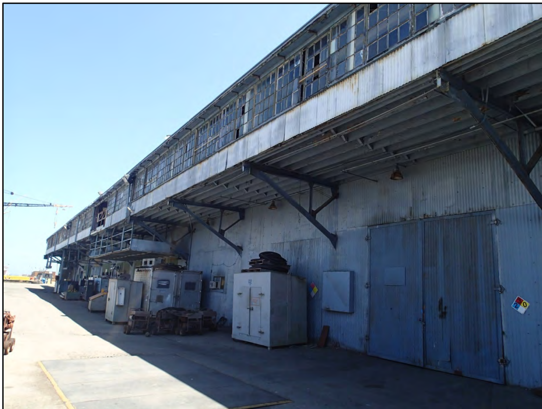
Figure 109-5 - Overall north view of Building 109 Mold Loft.
