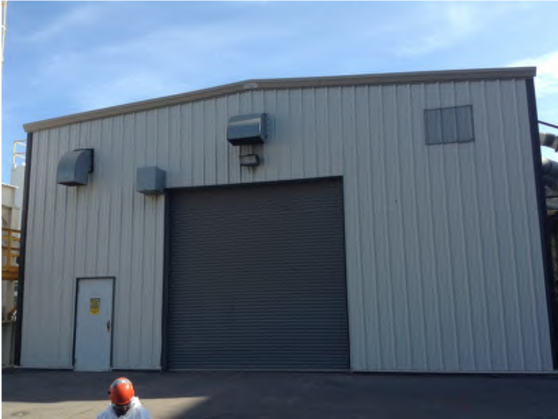
Fig. 1 - Building 251 view from front
