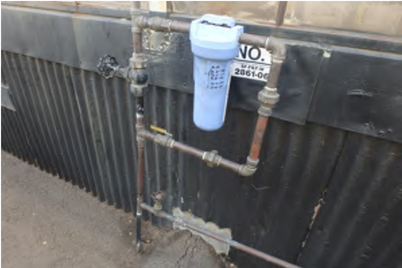
Figure 109-3 – Filtered CW service to nearby portable unit
