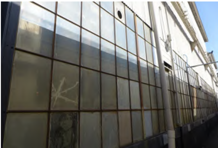
Figure 14 - Building 109, Plate shop south window.
