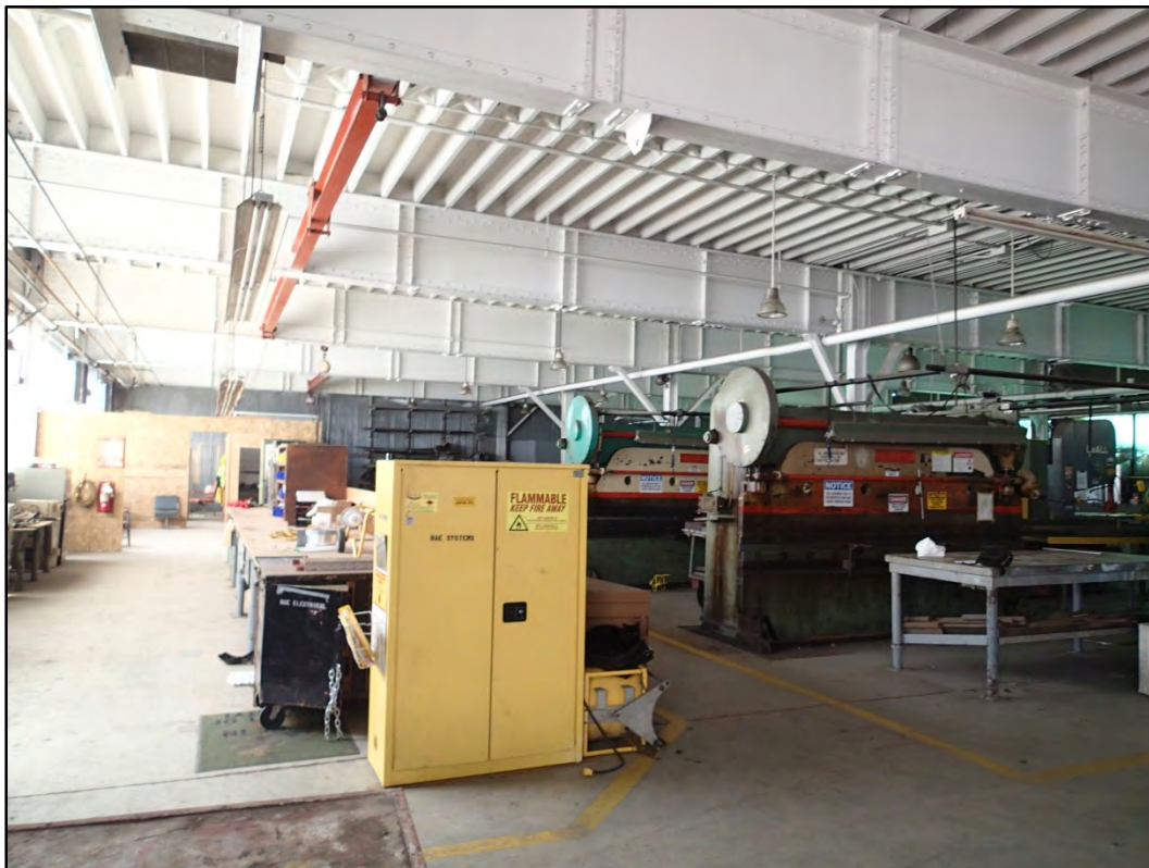
Figure 109-7 - Overall interior view of Building 109 Plate Shop.
