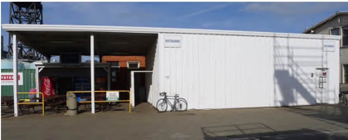
Figure 4 - Building 143: South Elevation
