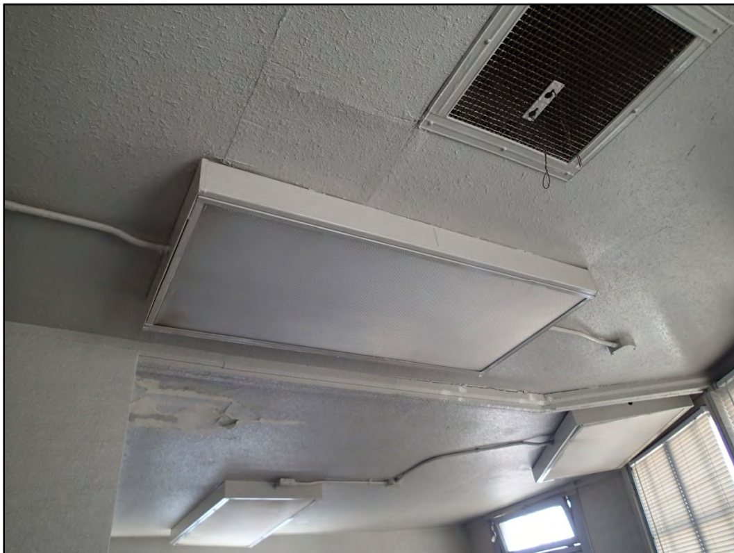
Figure 121-8 – View of typical interior ceiling condition of Building 121.
