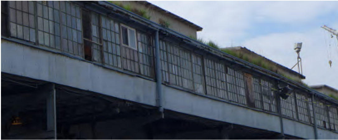
Figure 21 - Building 109, Mold loft windows, north elevation.
