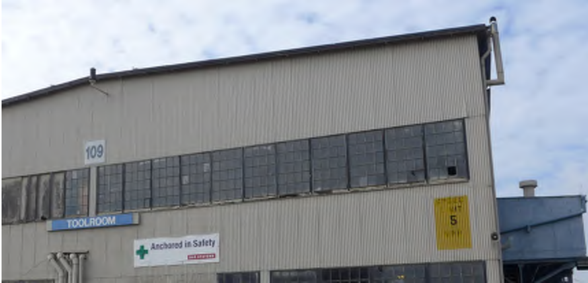
Figure 19 - Building 109, Mold loft east elevation.
