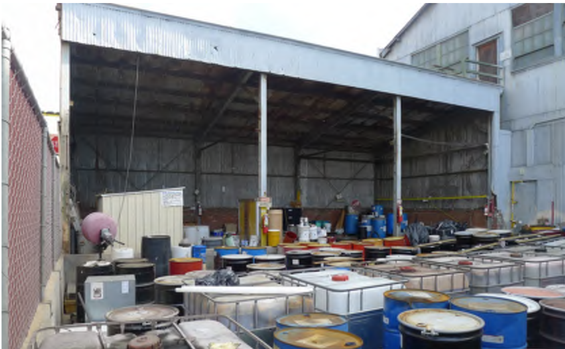
Figure 2 - Building 120: West Elevation
