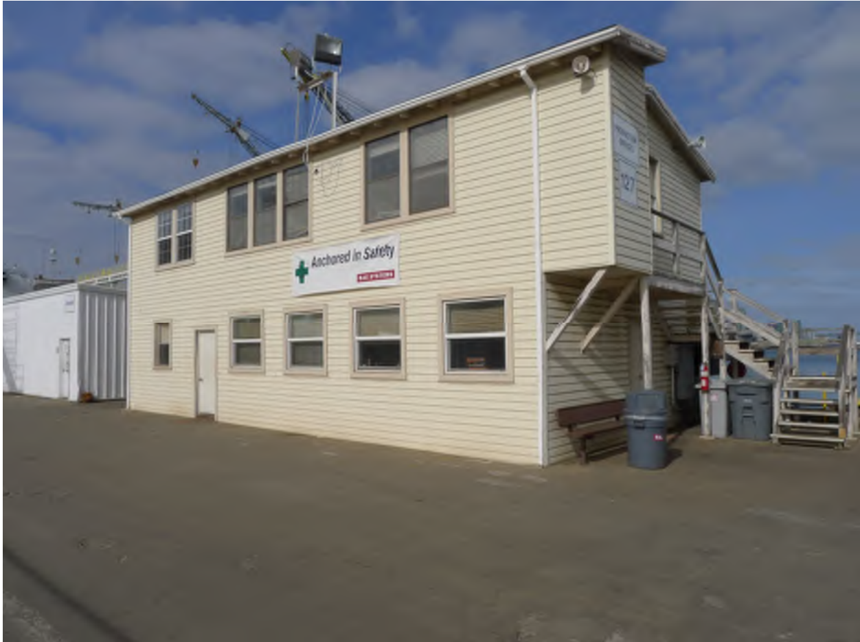
Figure 1 - Building 127, south elevation
