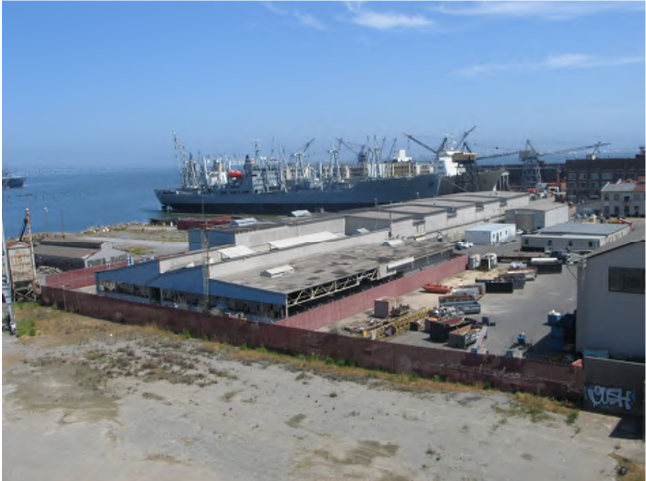
Figure 1 - Building 109, view from southwest
