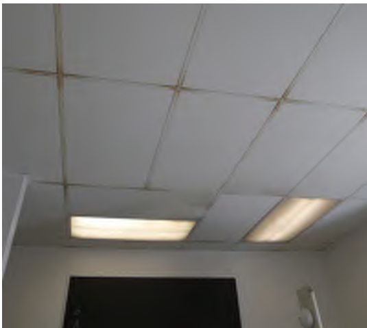
Figure 7 - Suspended ceiling, Men's Room
