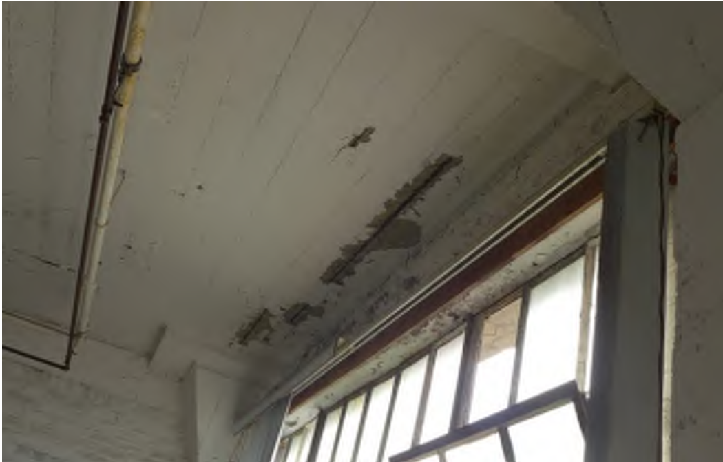
Figure 35 - Building 111, third floor ceiling
