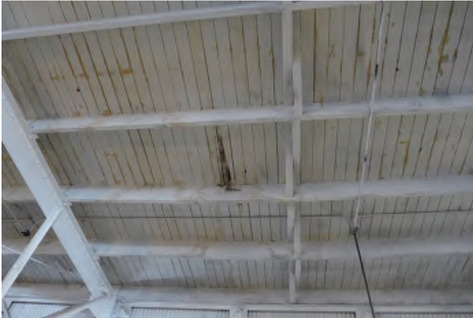
Figure 25 - Building 109, Mold loft T&G ceiling.
