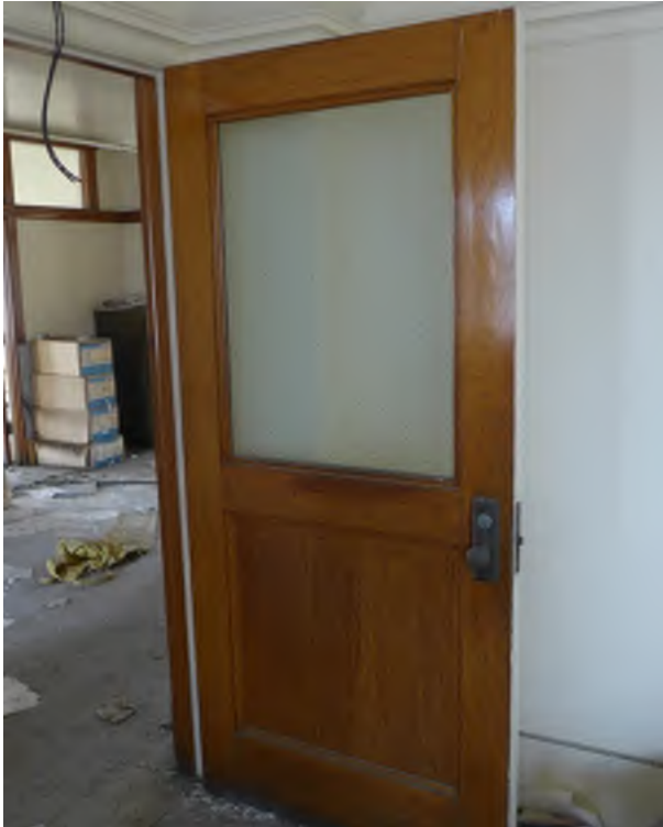
Figure 38 - Building 111, mezzanine office door
