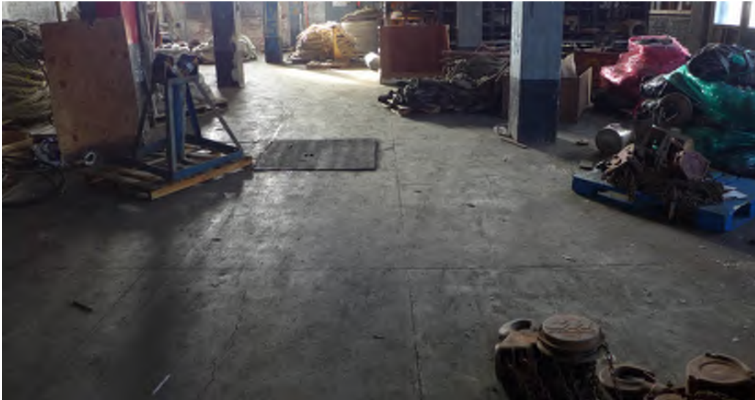
Figure 37 - Building 111, fourth floor concrete floor
