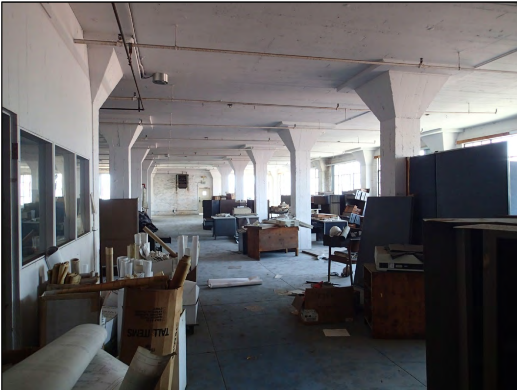
Figure 111-10 – View of fourth floor interior at the south end of Building 111.
