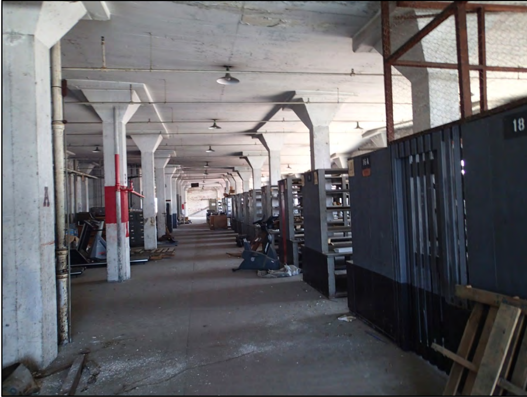
Figure 111-11 – View of fifth floor interior at the south end of Building 111.
