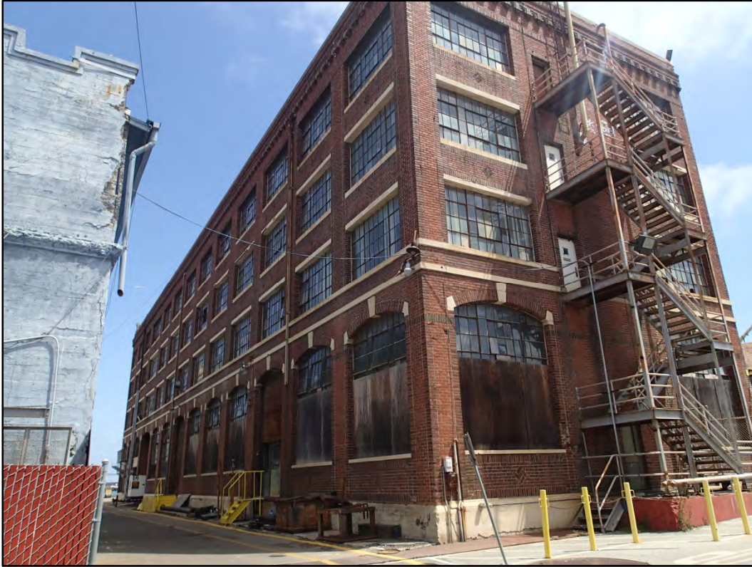
Figure 111-2 – Overall southwest view of Building 111.
