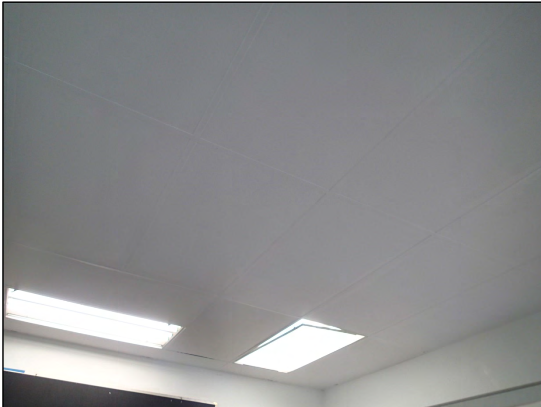
Figure 143-7 - View of typical interior ceiling condition of Building 143.
