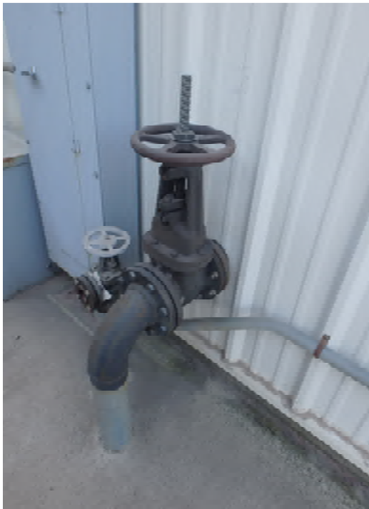
Figure 251-2 – 3” Service Line with Gate Valve
