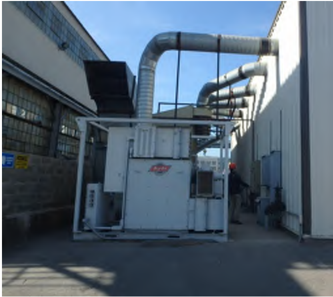
Figure 251-1 – Industrial Dehumidifiers
