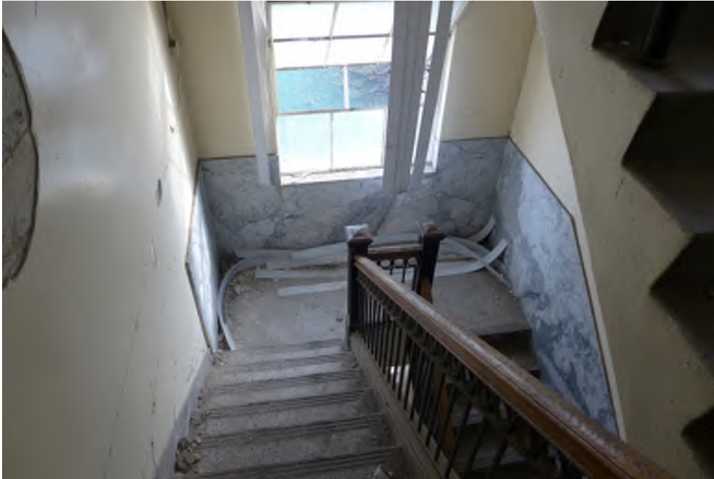
Figure 39 - Building 111, staircase from mezzanine to second floor level
