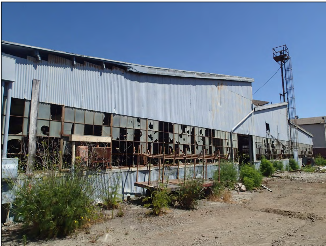
Figure 109-11 – Overall west view of the abandoned west section of Building 109.
