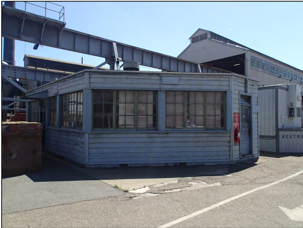
Figure 121-1 - Overall northeast view of Building 121.
