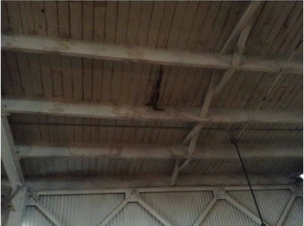
Fig. 1 - Building 109 view from the interior
