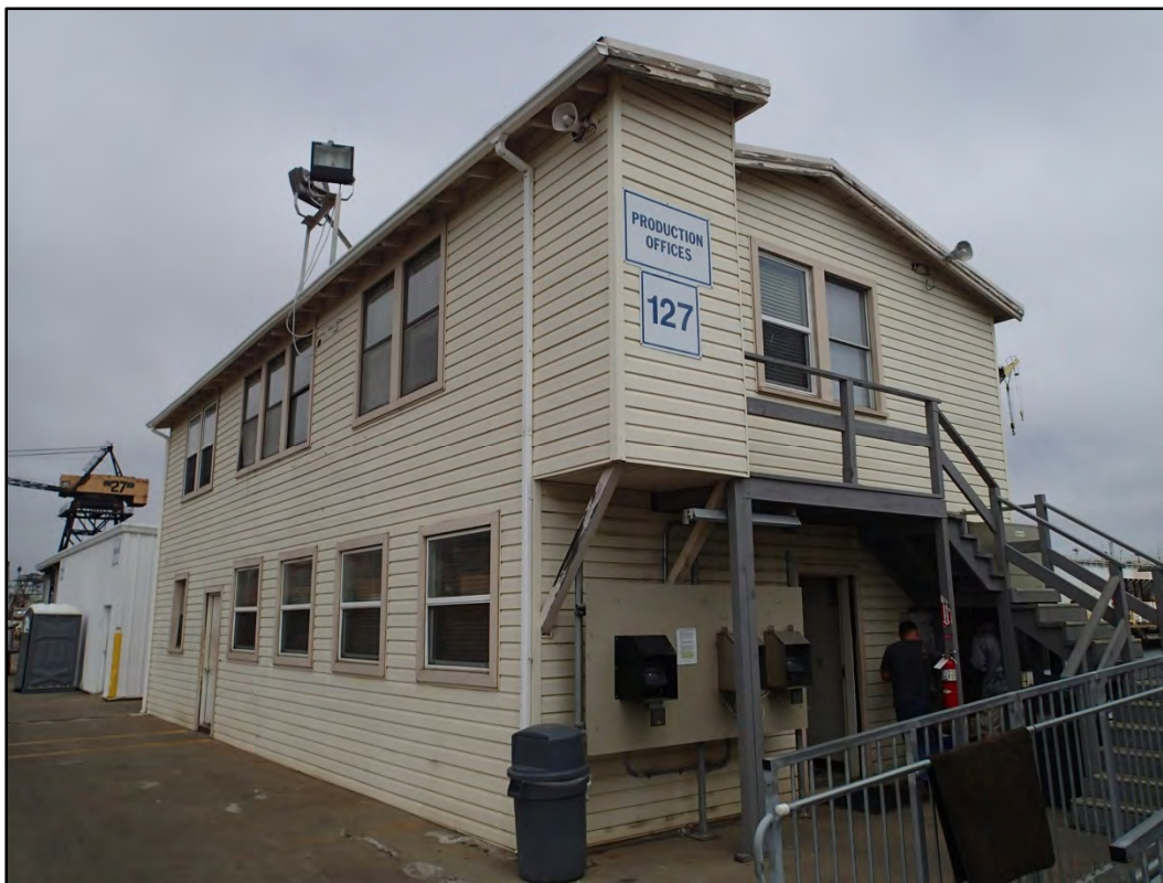
Figure 127-1 - Overall southeast view of Building 127.
