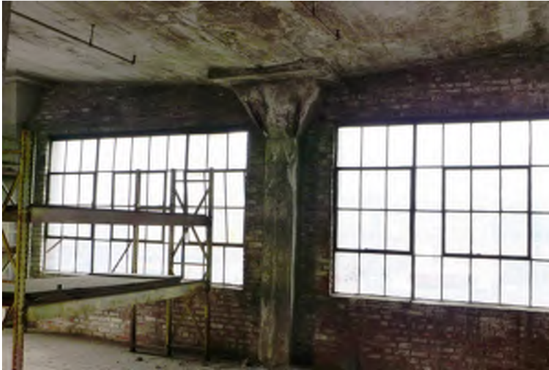
Figure 31 - Building 111, third floor exterior wall.
