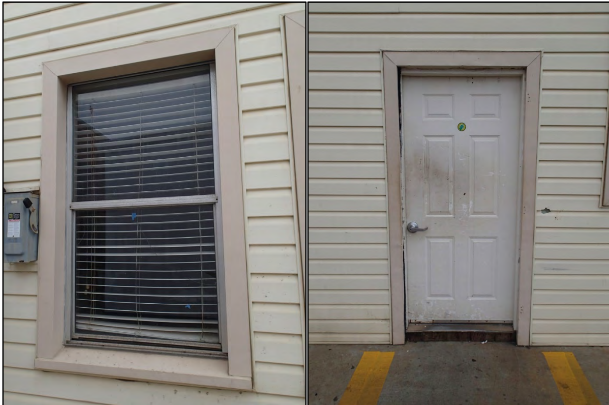
Figure 127-3 and Figure 127-4 – View of the typical windows and doors at Building 127.
