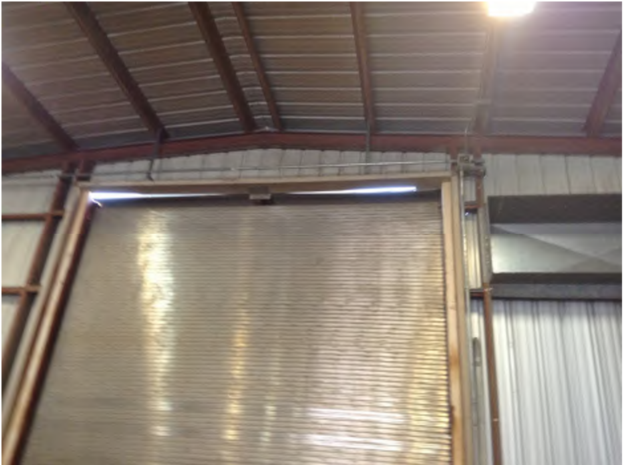
Fig. 1 - Building 250 view from interior
