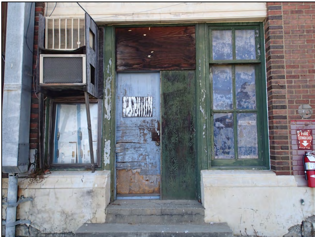
Figure 111-5 – Typical view of Building 111 wood doors.
