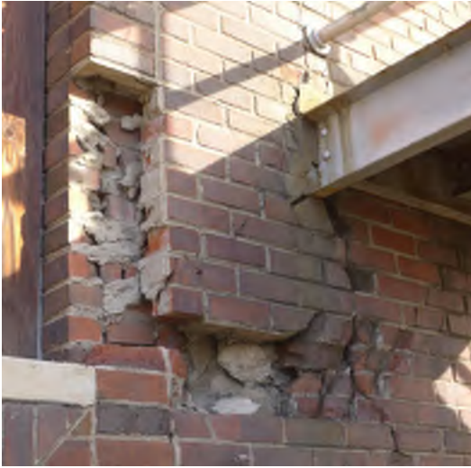
Figure 8 – Brick loss, south elevation
