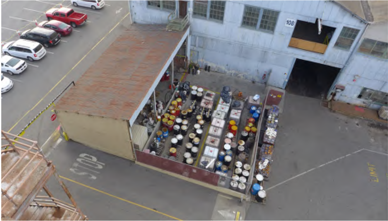
Figure 1 - Building 120, view from north
