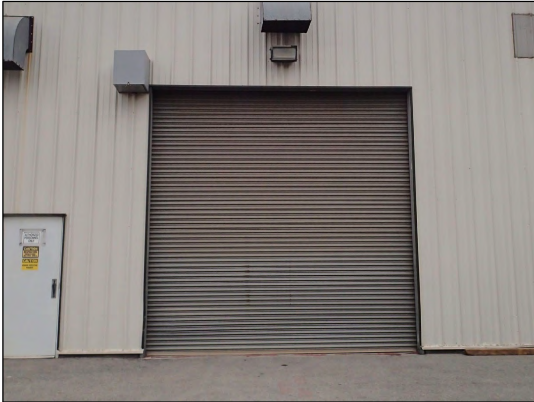
Figure 251-4 – View of steel roll-up door at Building 251.
