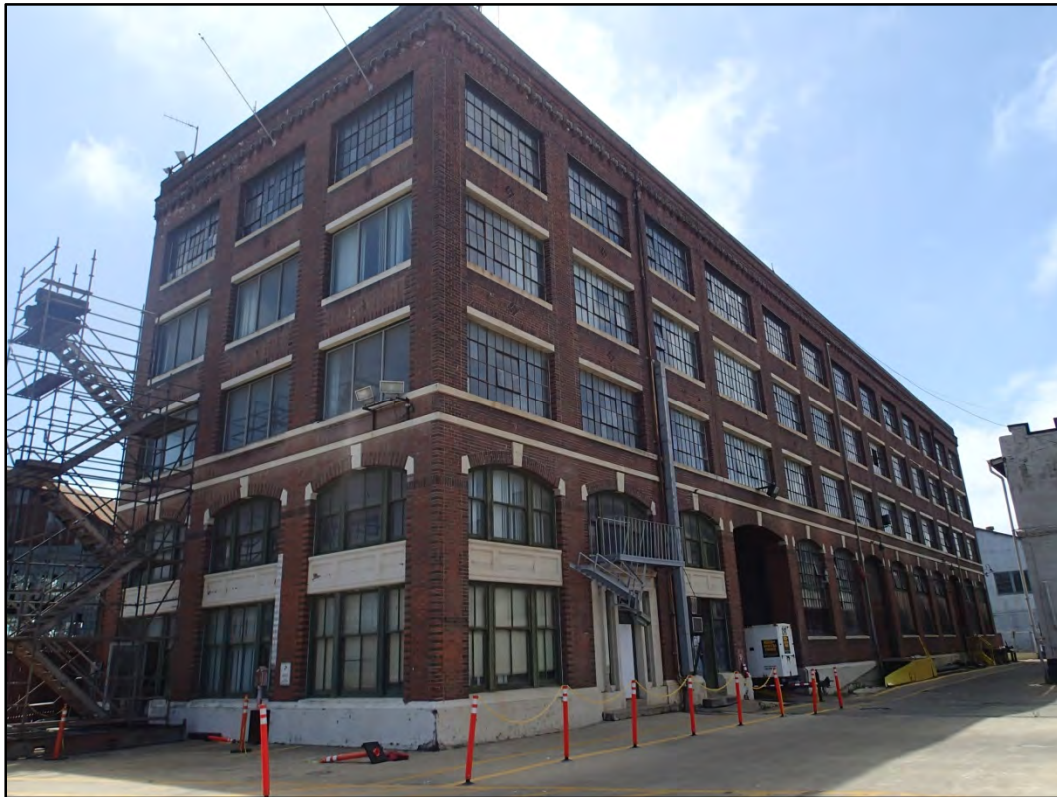
Figure 111-1 - Overall northwest view of Building 111.
