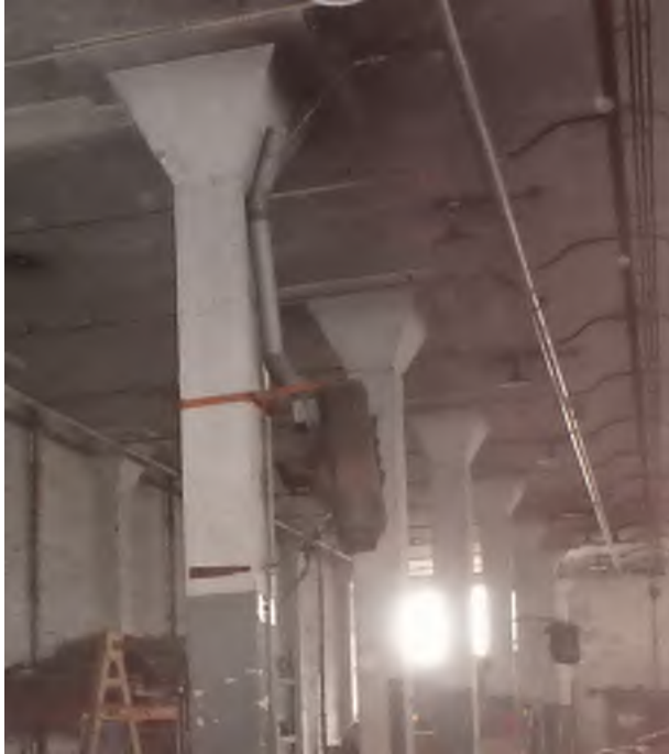
Figure 111-1 – Disused Unit Heater with Flue Connection Broken
