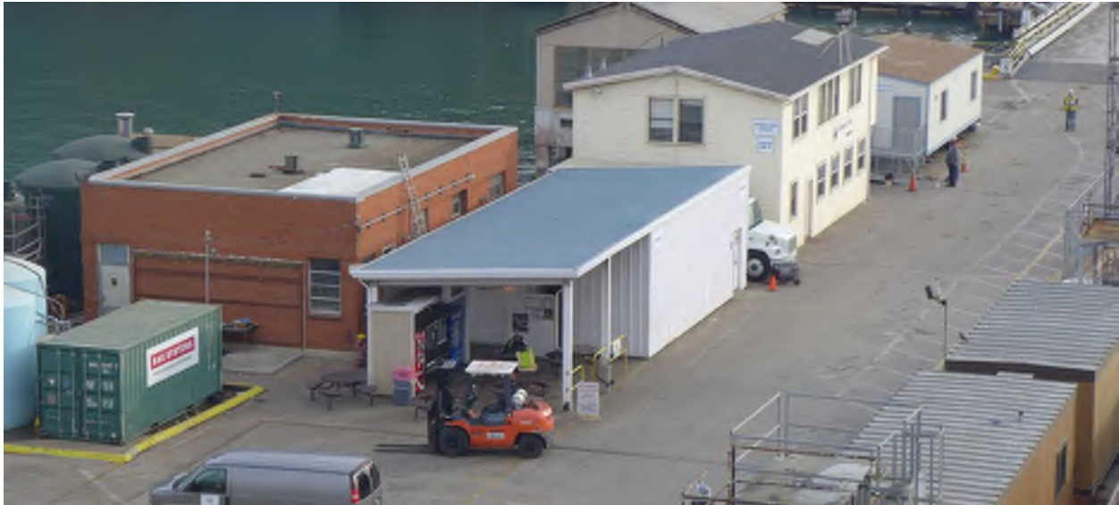
Figure 1 - Building 143, view from southwest
