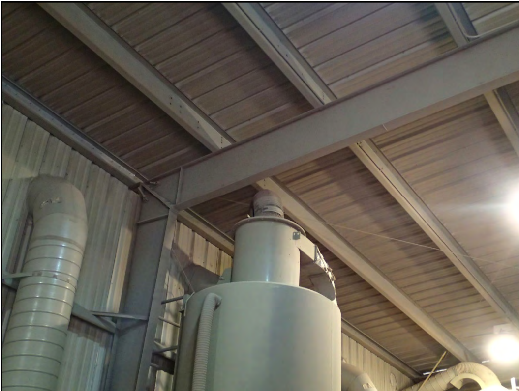
Figure 251-8 – View of the interior structural steel framing in Building 251.
