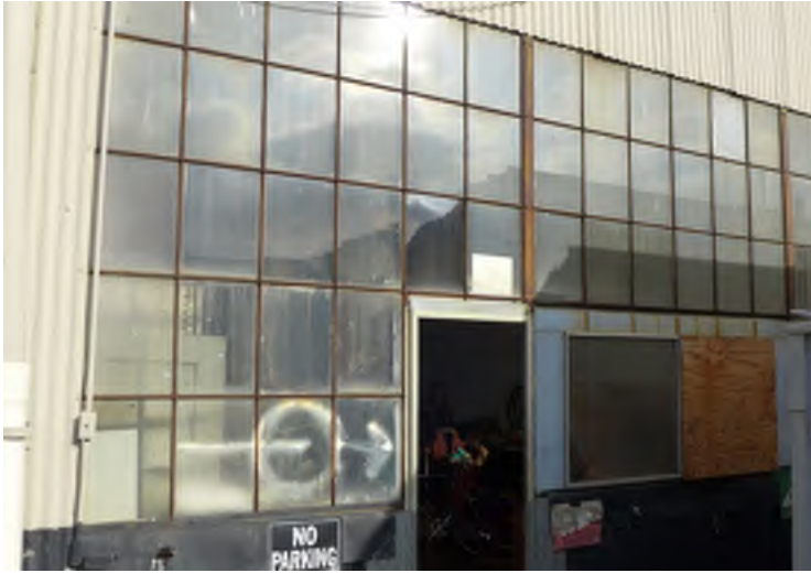
Figure 13 - Building 109, Paint shop south window.
