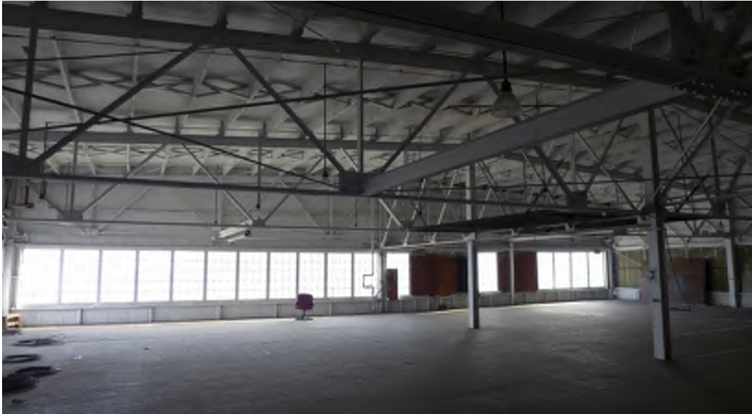
Figure 23 - Building 109, Interior of plate shop, facing west.
