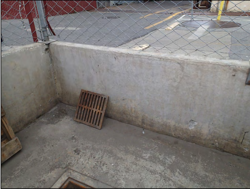
Figure 120-6 – View of typical interior paint deterioration in Building 120.
