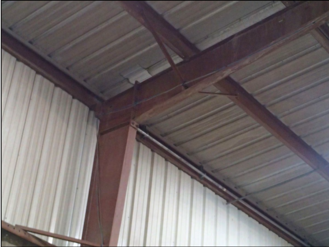
Figure 250-8 – View of the interior structural steel framing in Building 250.
