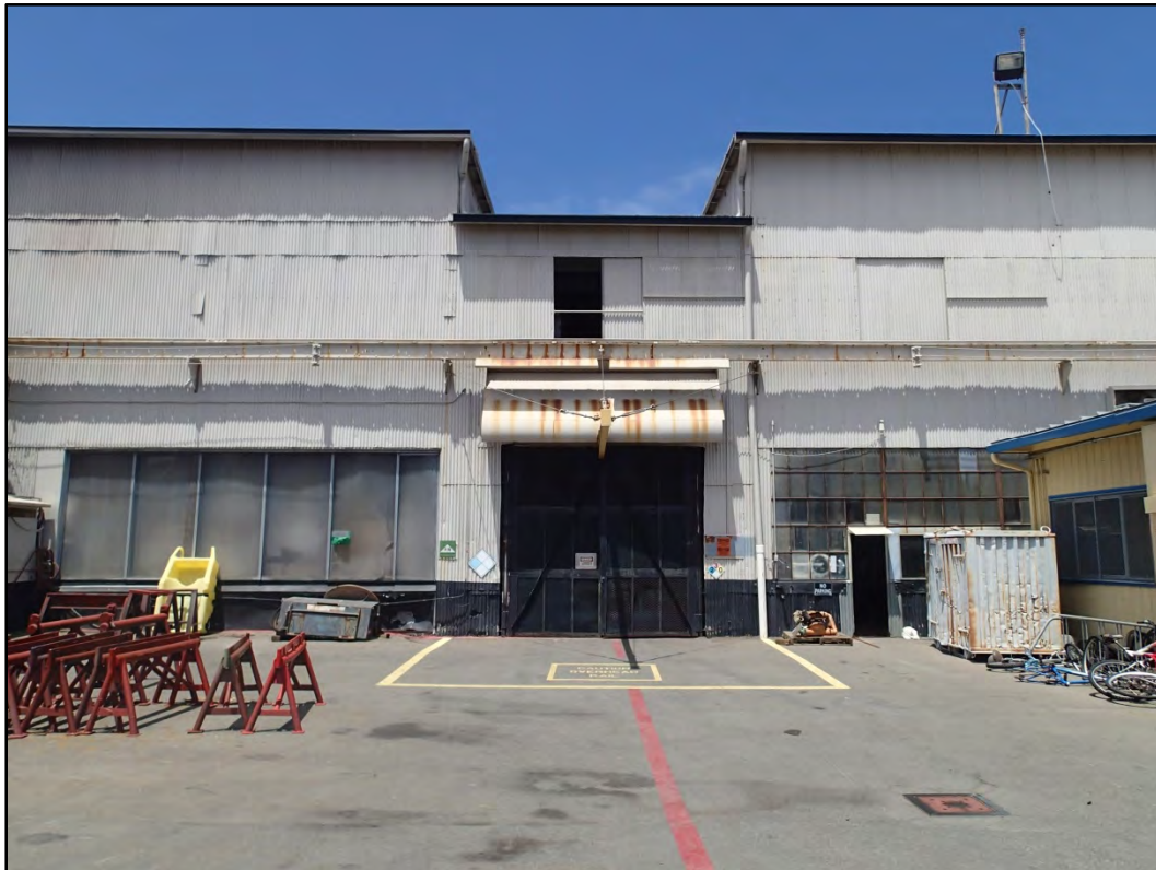
Figure 109-3 - Overall south view of Building 109 Paint Shop.
