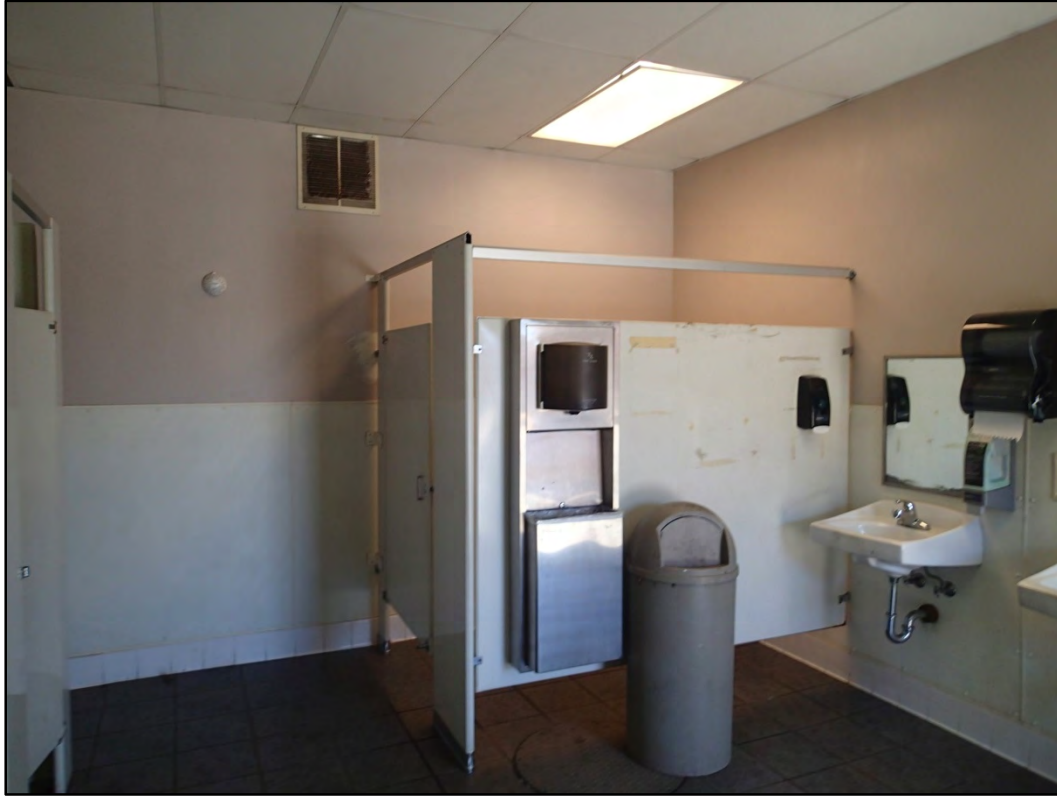
Figure 143-6 - View of typical interior condition of Building 143.
