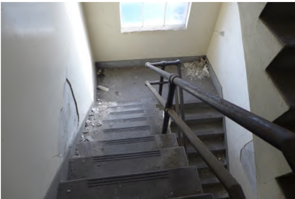
Figure 40 - Building 111, staircase from second floor to third floor
