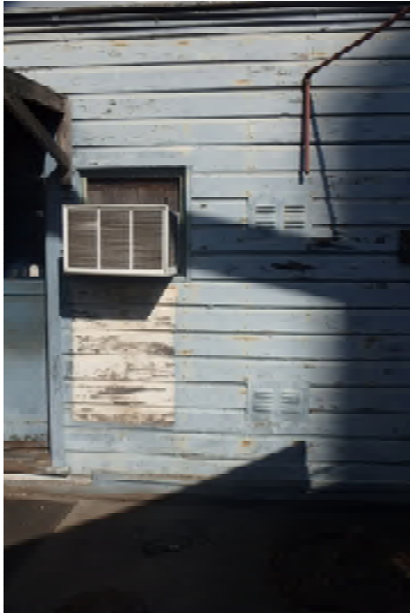
Figure 121-1 – Window-Mounted DX Cooling Unit
