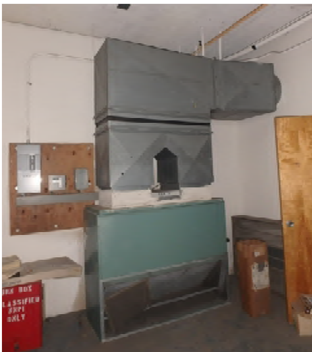
Figure 111-1 – Disused Unit Heater with Flue Connection Broken
