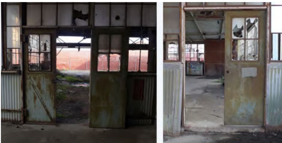
Figure 8 - Building 109, interior steel frame doors
