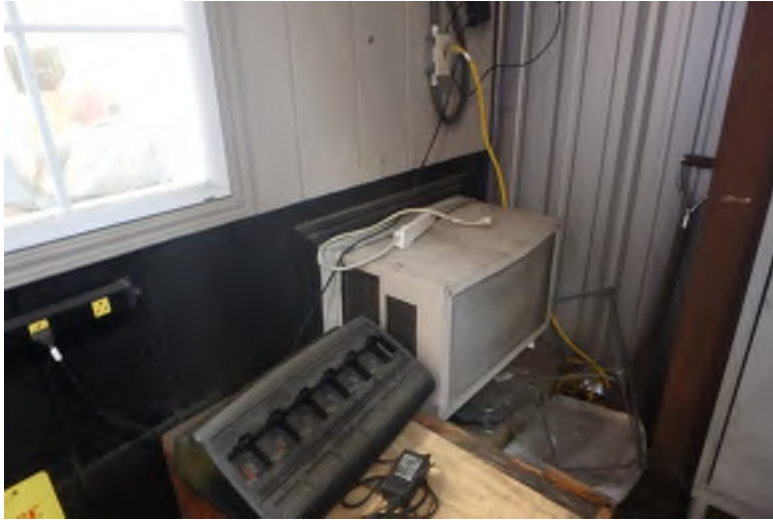
Figure 250-1 – Window Mounted DX Unit for Office
