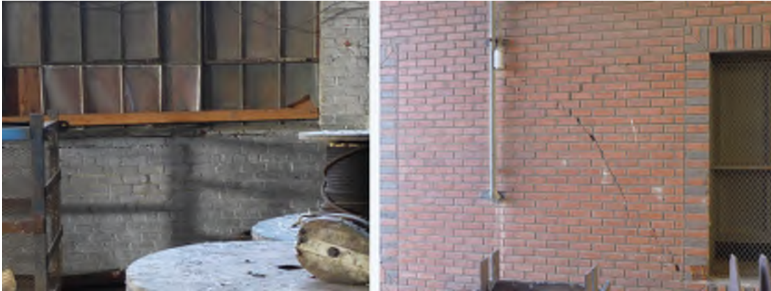
Figure 24 - Building 111, first floor warehouse wall Figure 25 - Building 111, first floor wall at loading dock
