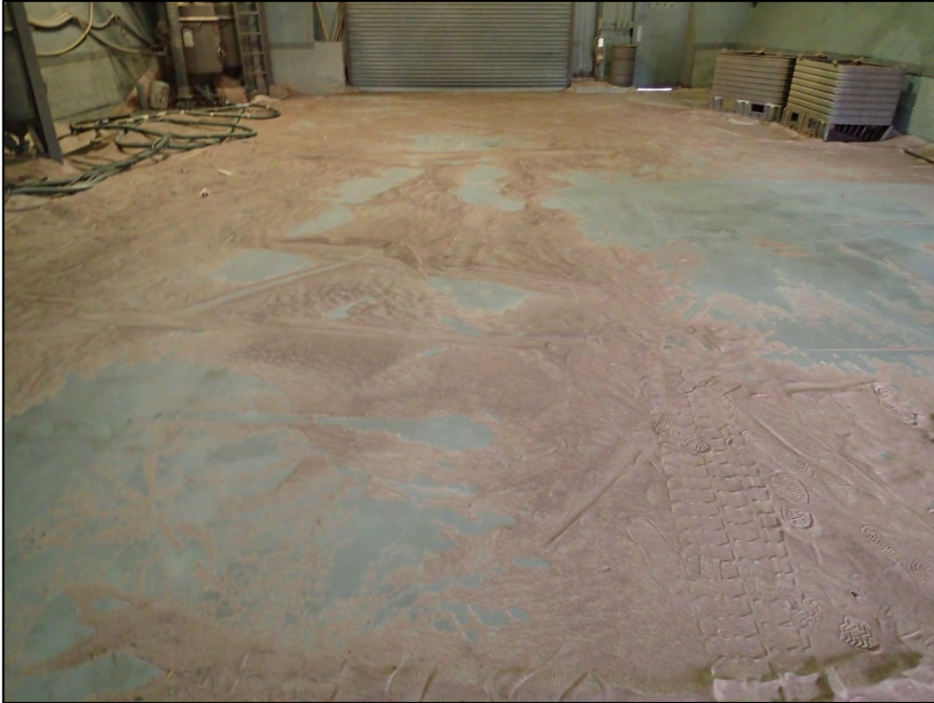
Figure 251-9 – View of the interior concrete slab in Building 251.
