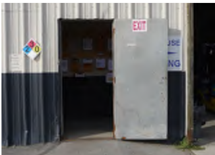
Figure 4 - East personnel door.
