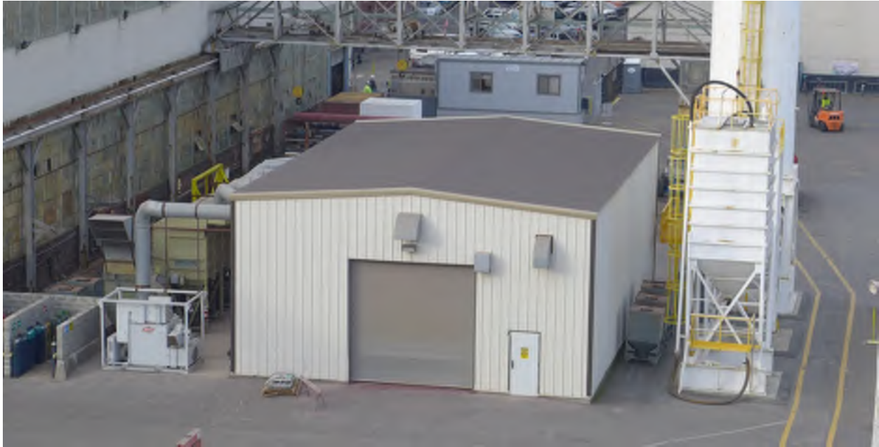
Figure 1 - Building 251, view from northwest
