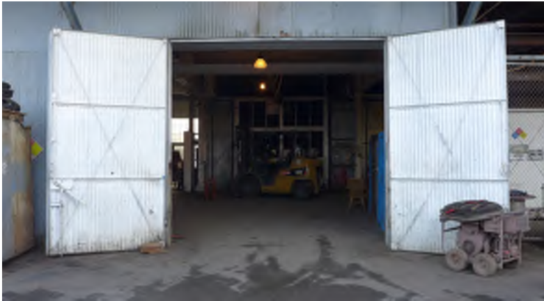
Figure 13 - Building 109, Paint shop north door.
