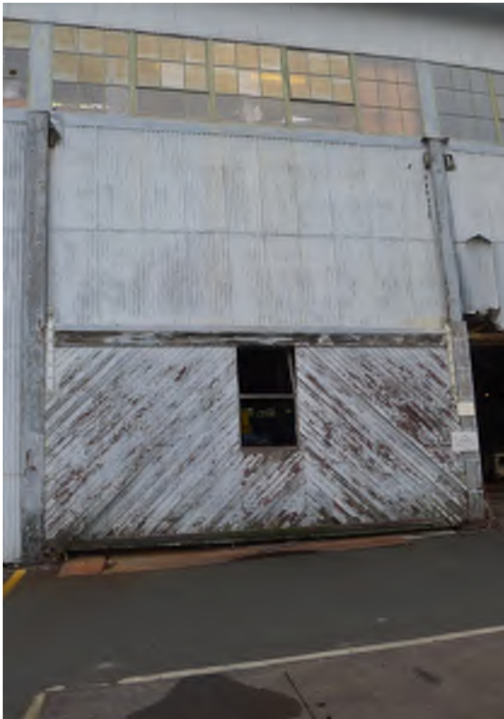
Figure 18 – West elevation, north loading door.
