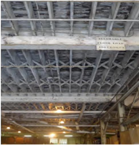
Figure 33 – Ceiling, east side looking south.
