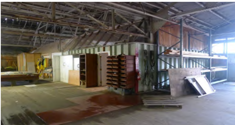
Figure 43 – Interior shed, employee area, north west side. Looking northwest.
