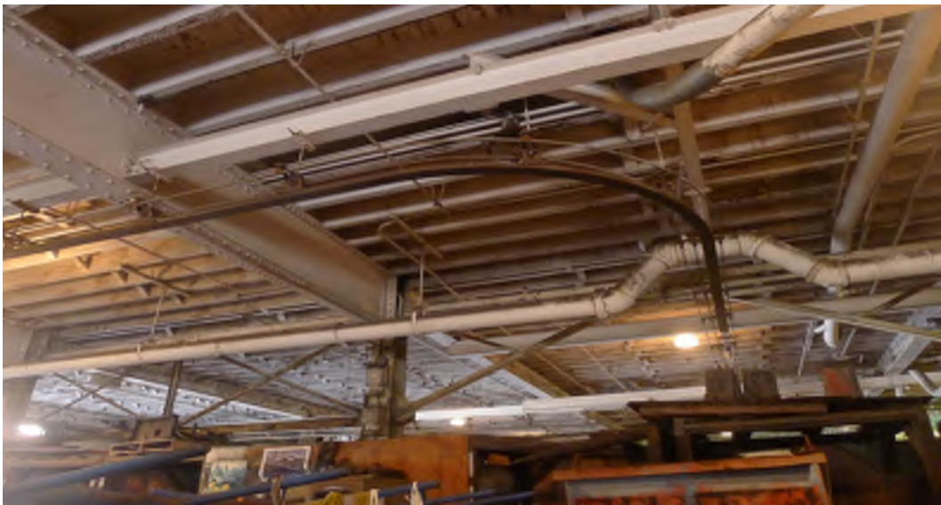
Figure 50 – First floor, overhead trolley rails
