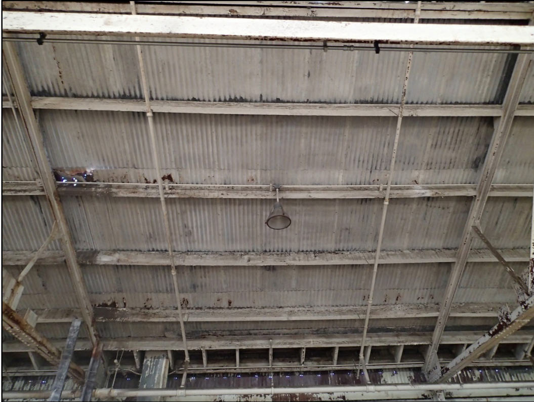
Figure 108-8 - View of Building 108 roof structure and corrugated metal panels.
