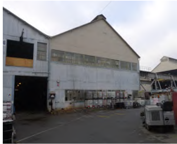
Figure 3 – North elevation, west side
