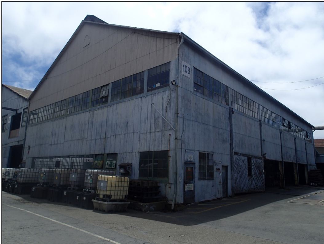
Figure 108-1 - Overall northwest view of Building 108.
