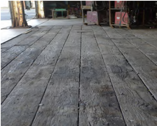
Figure 38 – Wood floor, west side at loading bays.
