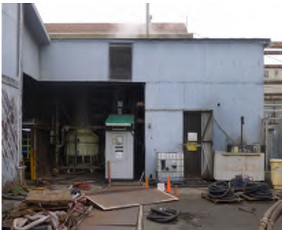
Figure 6 – South end, west side electrical shed
