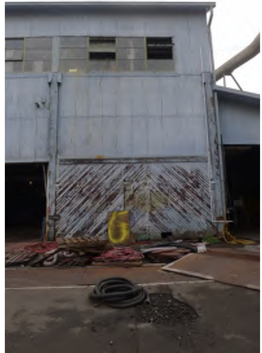
Figure 19 – West elevation, south door
