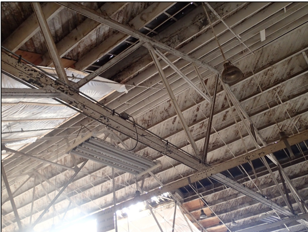
Figure 108-9 - View of Building 108 roof structure and wood diagonal sheathing.
