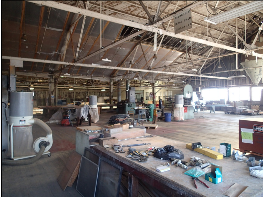
Figure 108-6 - Overall second floor interior view of Building 108, looking southeast.
