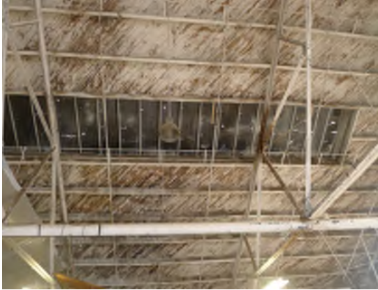
Figure 36 - Wood ceiling, east side.
