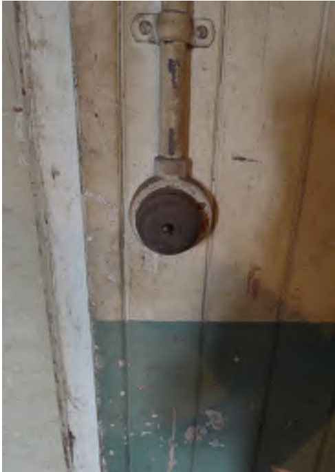
Figure 48- First floor, historic light switch.
