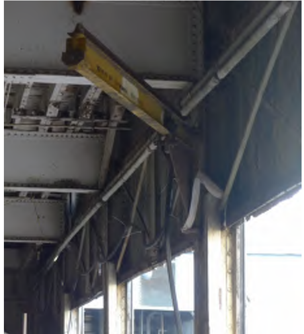
Figure 49 –First floor, swinging arm crane,
