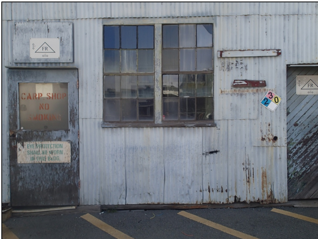
Figure 108-5 - View of typical condition of Building 108 windows and doors.
