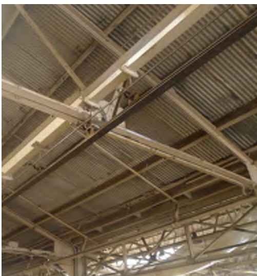
Figure 35 – CMP ceiling looking southwest.
