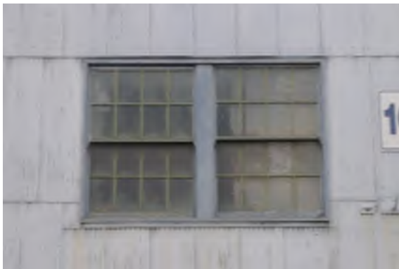
Figure 14 –South wall, typical bay
