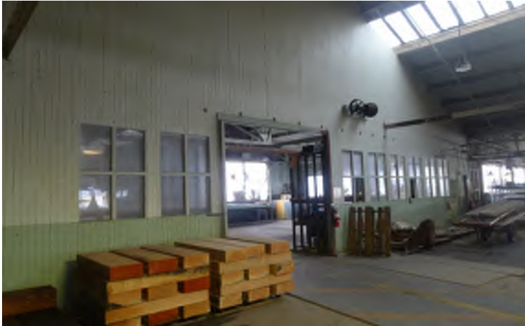
Figure. 30 – Second floor T&G wood partition wall, south end, east side.
