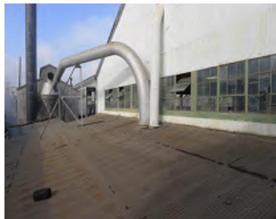
Figure 7 – South elevation, west side
