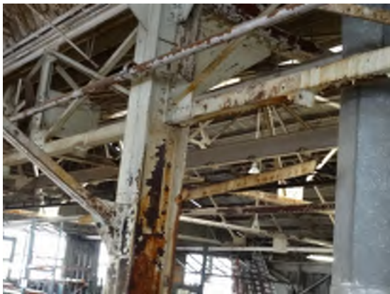
Figure 3 – Removed/Damaged brace
