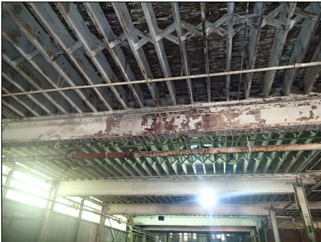
Figure 108-7 - Overall interior view of Building 108 second floor framing.
