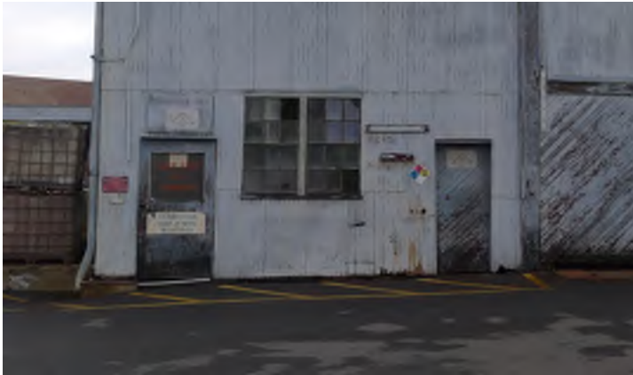
Figure 15 –Wood personnel doors, west elevation
