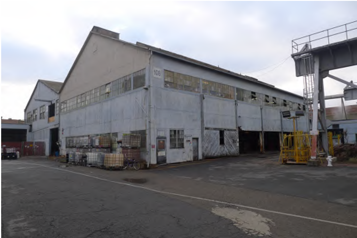
Figure 1 - Building 108, view from the northwest
