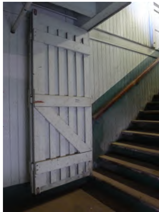
Figure. 32 – Unique, bi-fold door to second floor.
