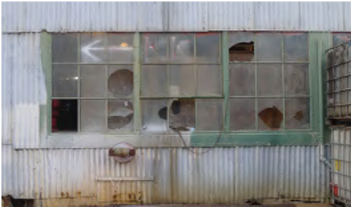
Figure 13 - view from the northwest
