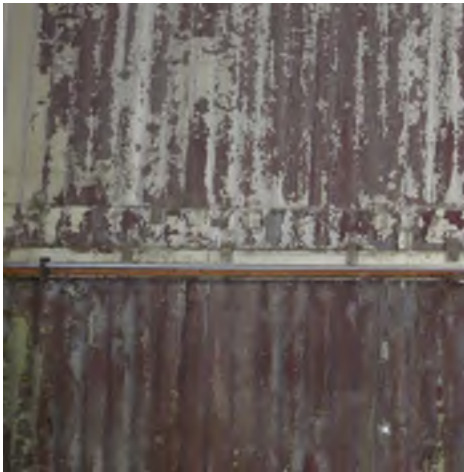
Figure. 27 – Interior side CMP, second floor.
