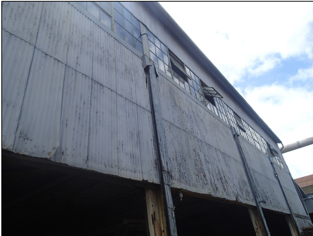
Figure 108-3 - Typical view of Building 108 exterior corrugated metal panels.
