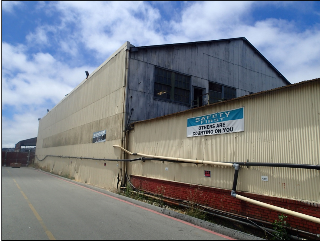
Figure 108-2 - Overall northeast view of Building 108.
