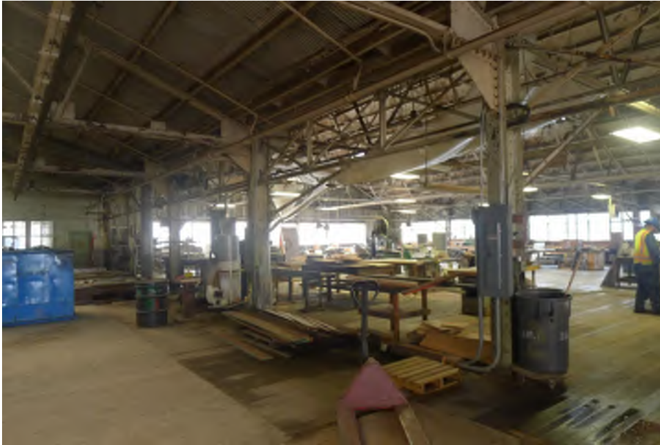
Figure 40 - Steel structure in east side, looking southwest.
