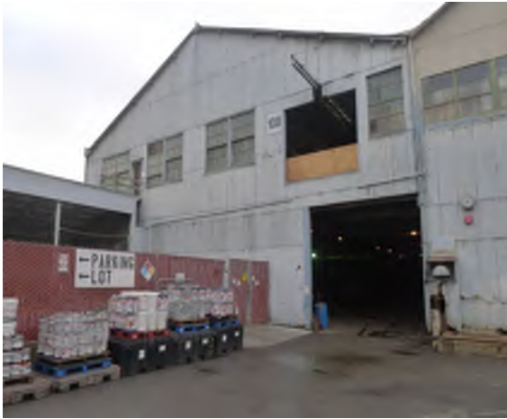
Figure 2 –North elevation, east side
