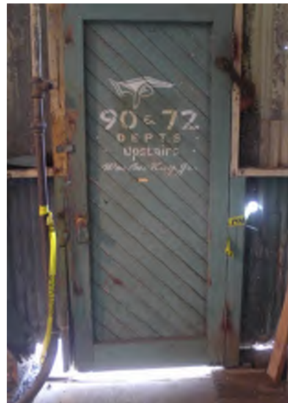
Figure 17 - Interior of same personnel door
