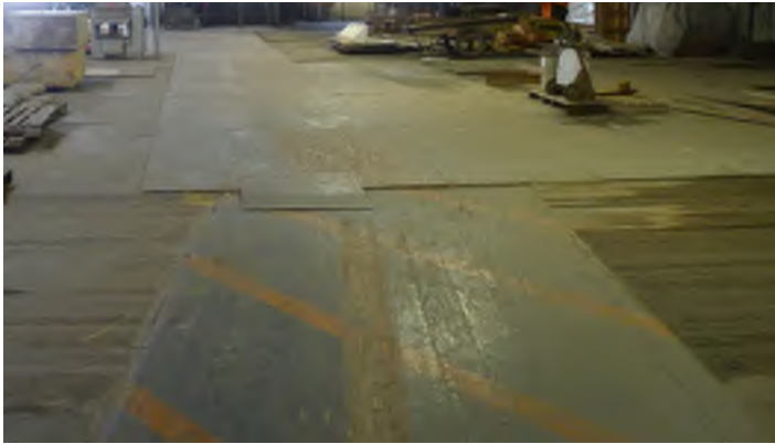
Figure 39- Typical second floor, floor with plywood over-lay.
