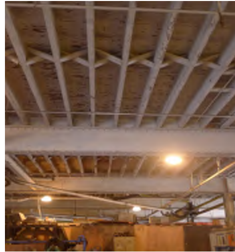
Figure 34 – Ceiling, west side looking south...
