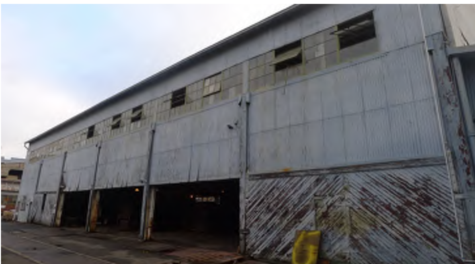
Figure. 8 – West elevation showing two out of five vertical lift loading doors.
