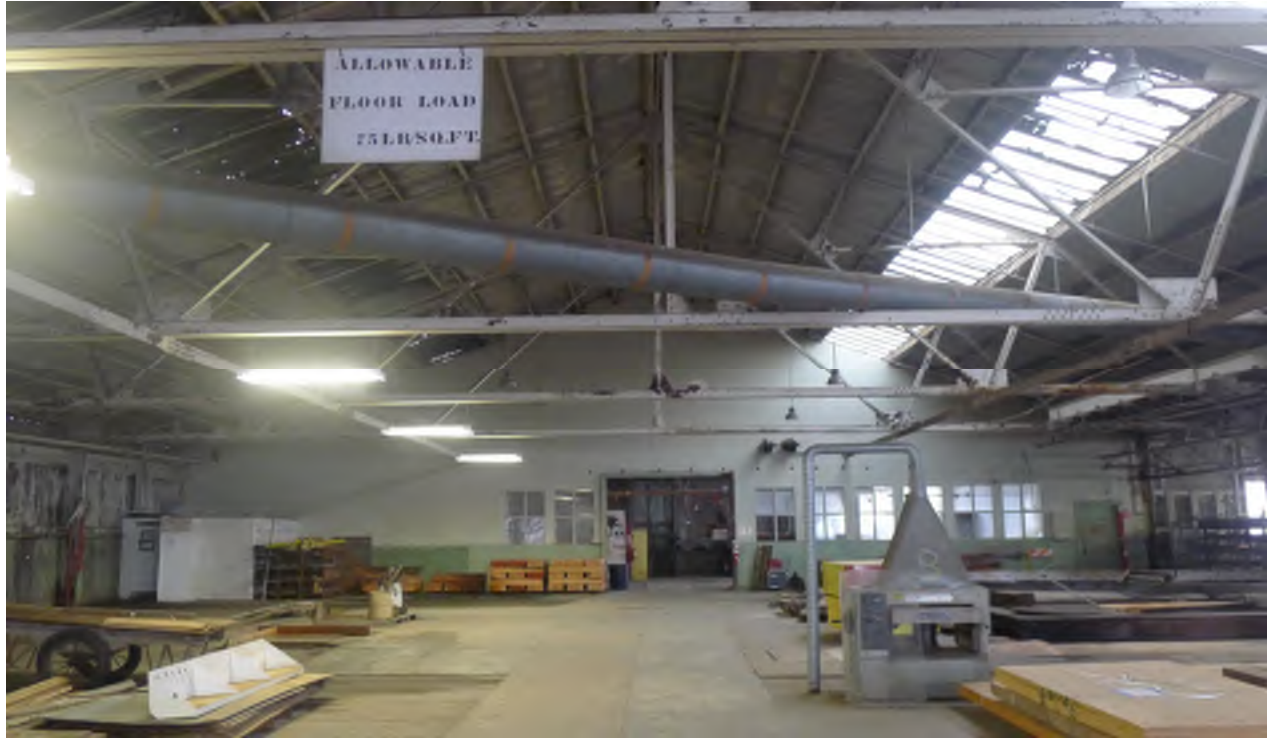
Figure. 25 - Building 108: Second floor, interior view looking south, east side.
