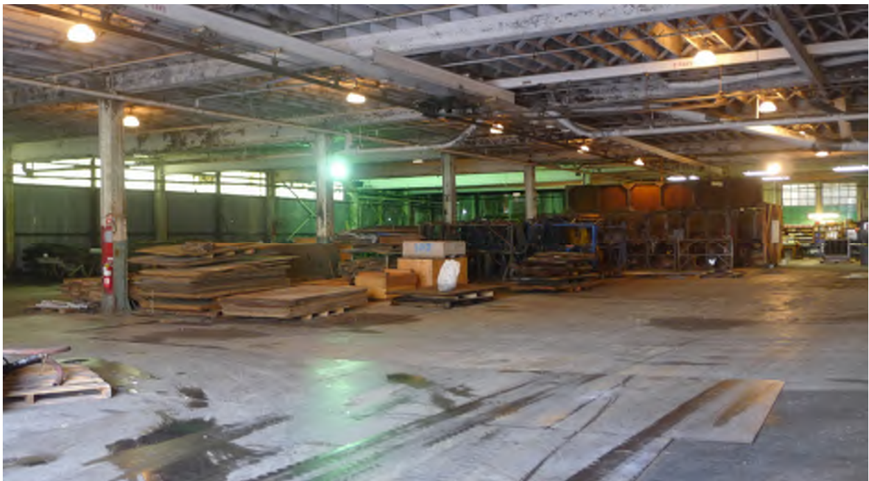
Figure. 24 - Building 108: First floor, interior view looking south, east side.
