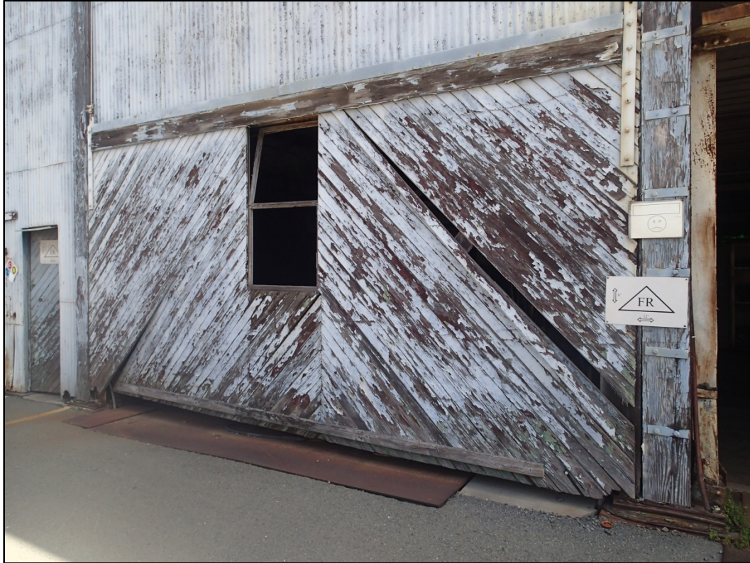
Figure 108-4 - View of Building 108 wood sliding door located on the west side.
