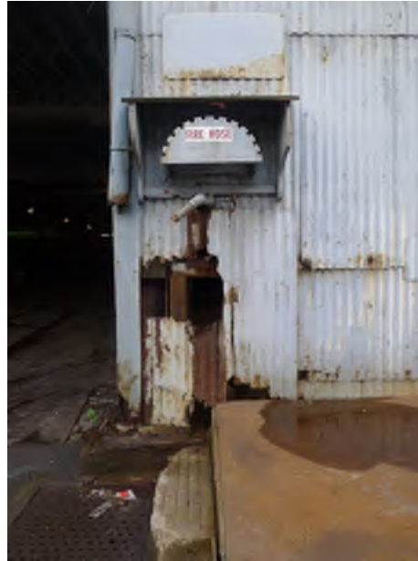
Figure 21 – North elevation, electrical equipment
