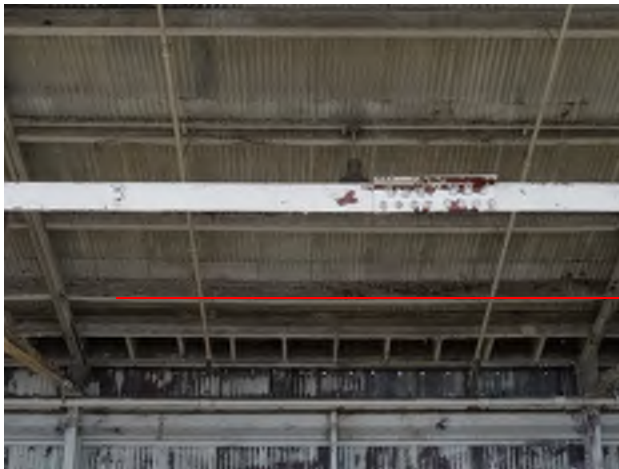
Figure 6 – Typical wood purlin sagging (redline drawn for clarity)
