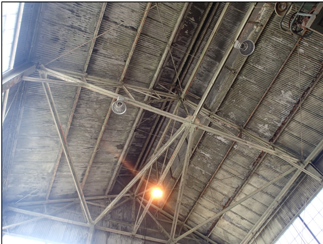
Figure 103-6 – View of Building 103 roof structure and corrugated metal panels.
