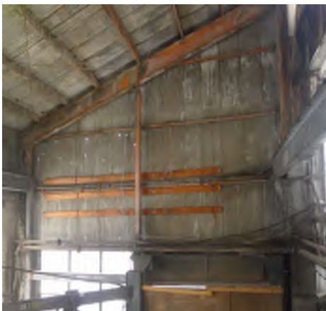
Figure. 24 - View looking west, south shed CMP
