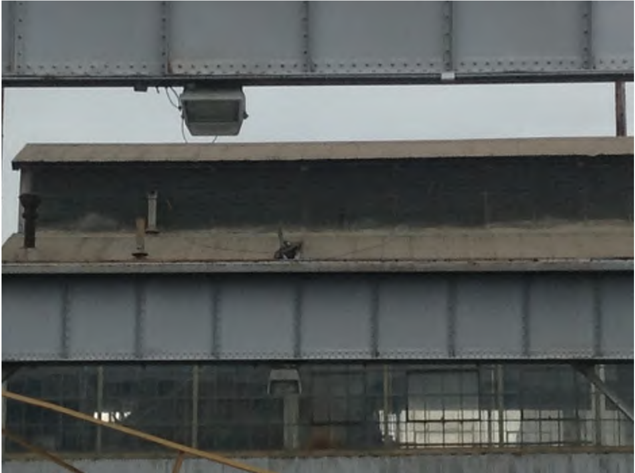
Fig. 1 - Building 103 view from N.W exterior
