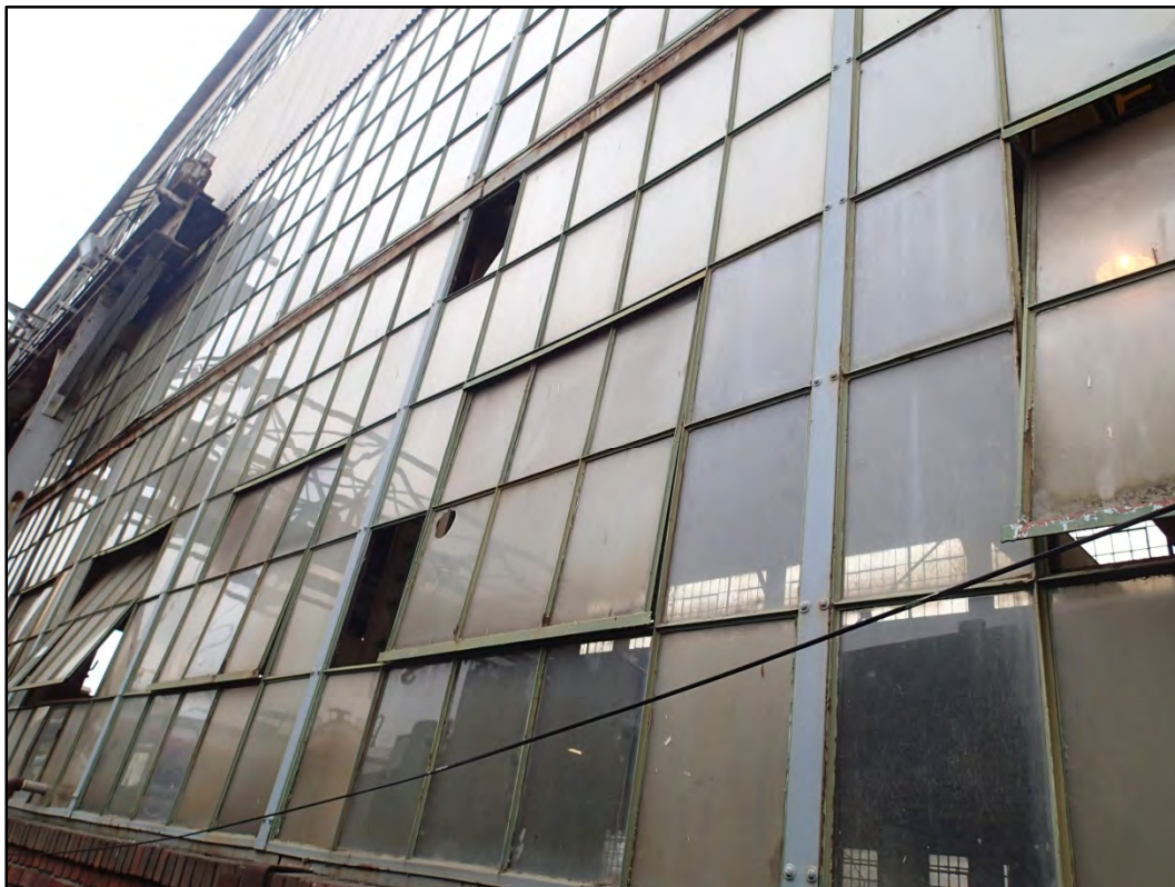
Figure 105-3 - View of Building 105 typical exterior steel window condition.
