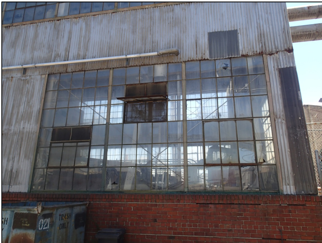
Figure 103-3 - View of Building 103 typical exterior window condition.
