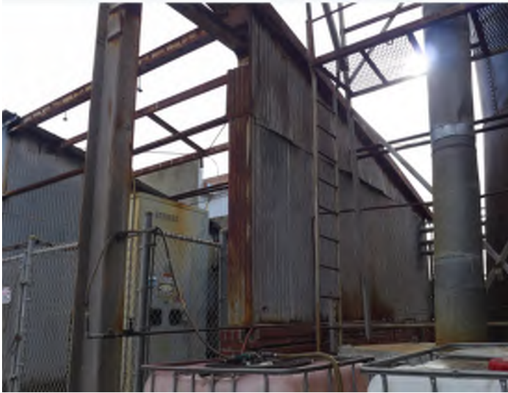
Figure 2 - Building 107: West Elevation
