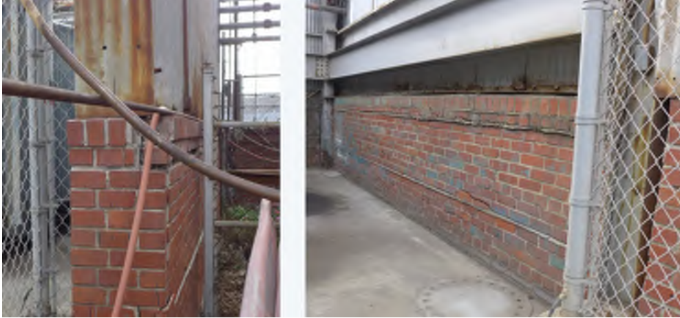
Figure 3 - Building 107: Brick at west wall. Figure 4 - Building 107: Brick at south wall.
