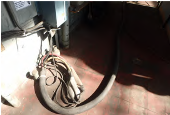
Figure 103-2 – Flexible Cable Power Feed
