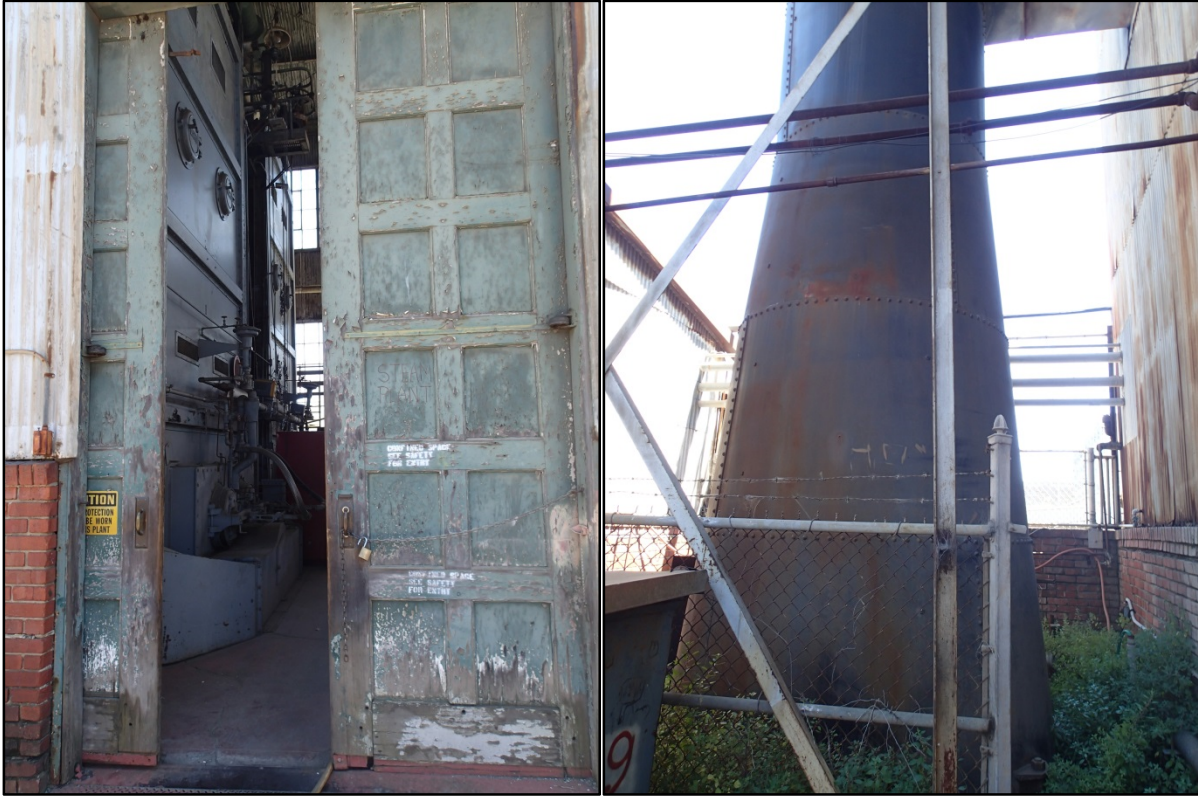
Figure 103-4 & Figure 103-5 –View of Building 103 exterior sliding door and smokestack, respectively.
