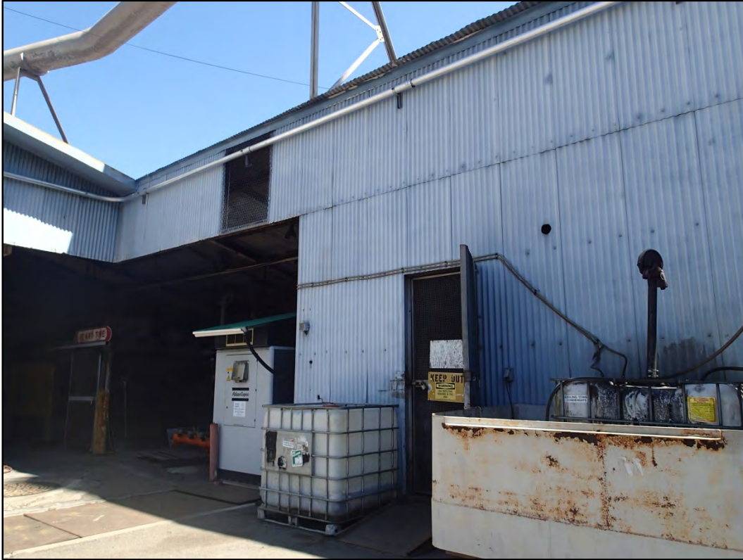
Figure 107-2 – Typical view of Building 107 exterior corrugated metal panels.
