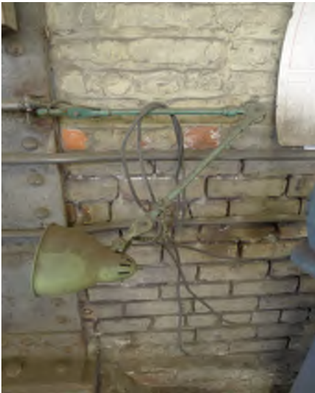
Figure. 26 – South shed brick wall.
