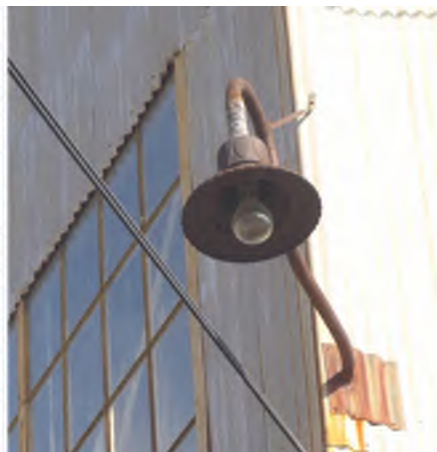
Figure 11 - Building 103: Lamp at southwest corner
