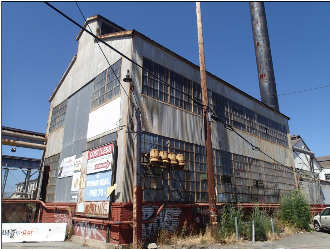
Figure 103-1 - Overall southwest view of Building 103.
