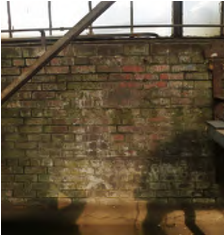
Figure. 25 - North main shed brick base wall.
