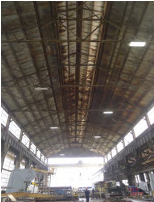
Figure. 20 - View looking east, main shed
