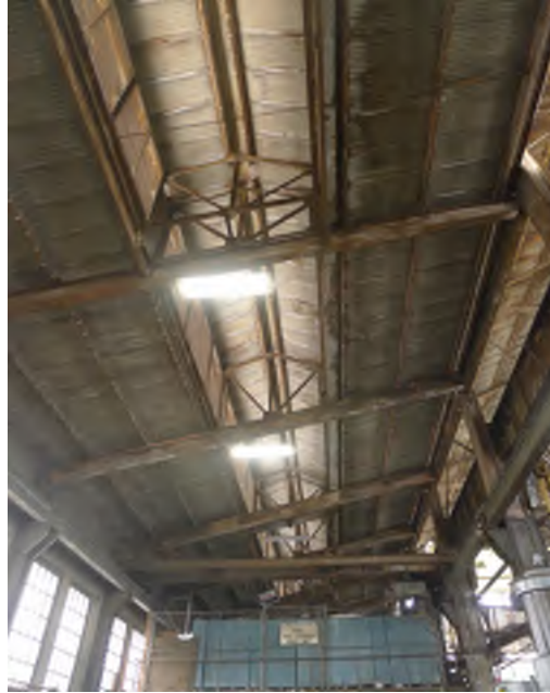
Figure. 23 - View looking west, south shed ceiling
