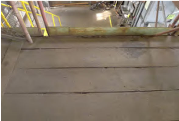
Figure 29 - Locker room mezzanine looking north.
