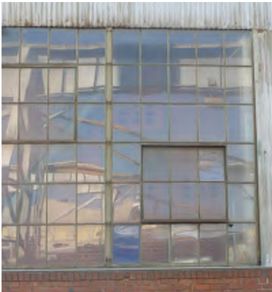
Figure 8 - Building 103: Window detail
