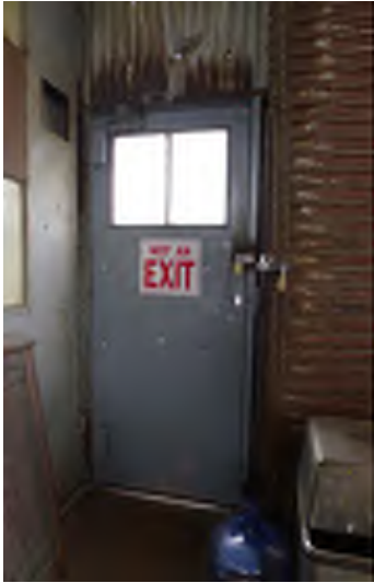
Figure 17 – West wall, steel personnel door
