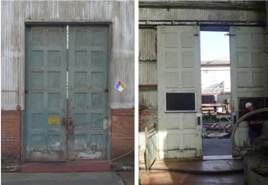
Figure 9 - Building 103: Rolling door at north elevation
