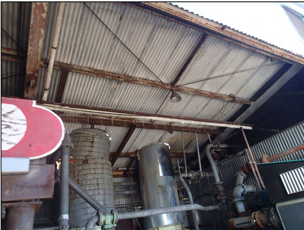
Figure 107-5 – Overall view of Building 107 west interior shed area, looking southwest.
