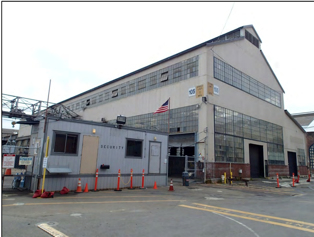
Figure 105-1 - Overall northwest view of Building 105.
