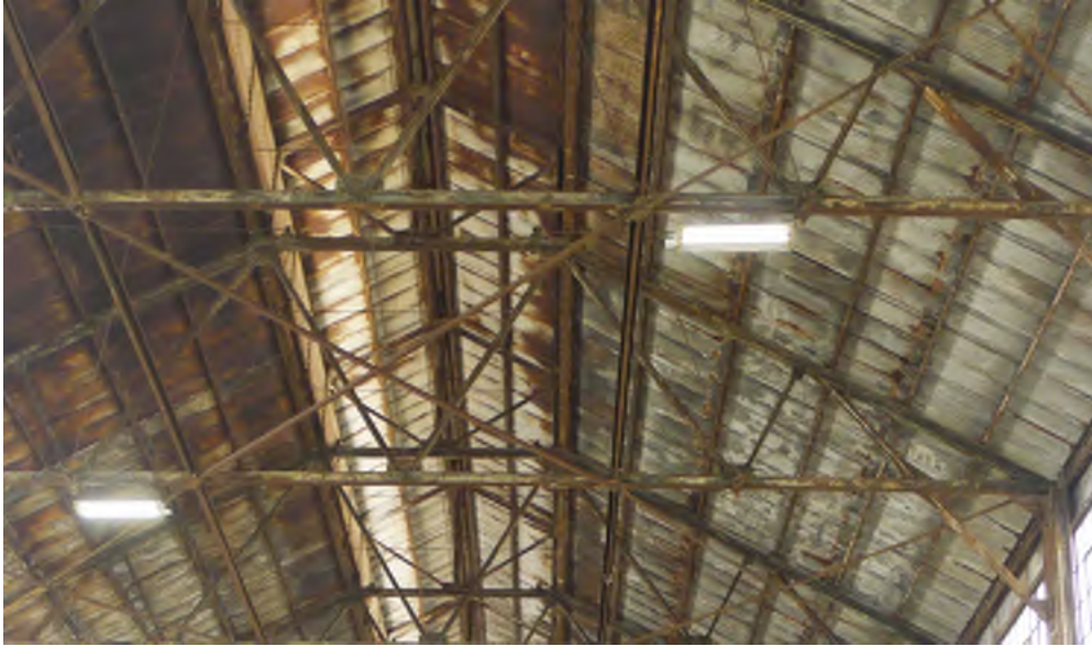
Figure 27 - Interior main shed ceiling looking west.
