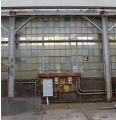
Figure 13 – North wall, typical bay
