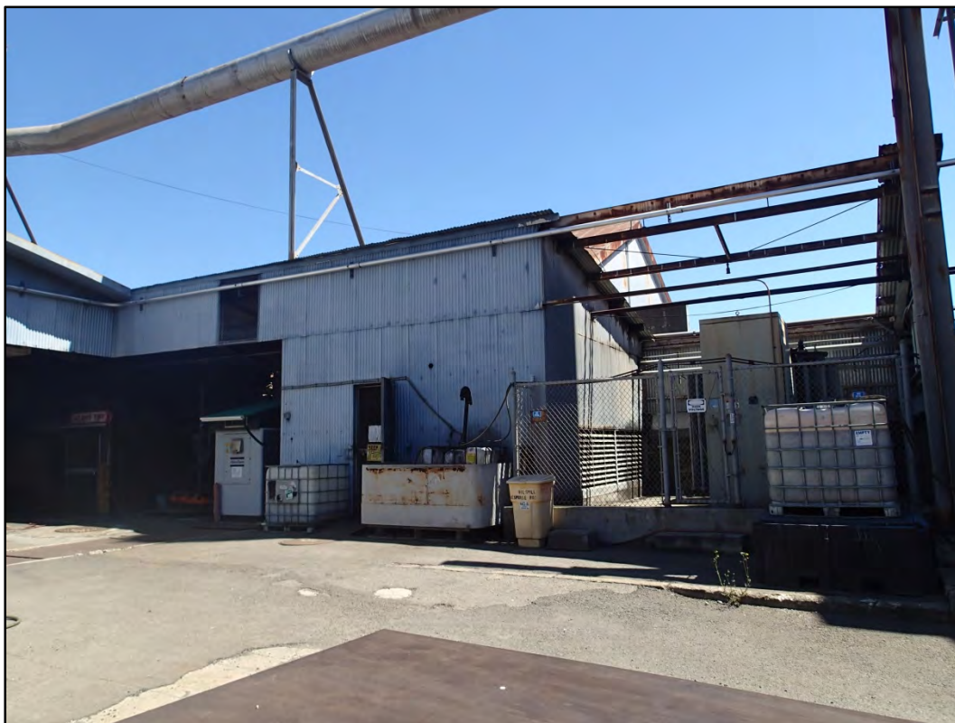
Figure 107-1 - Overall northwest view of Building 107.
