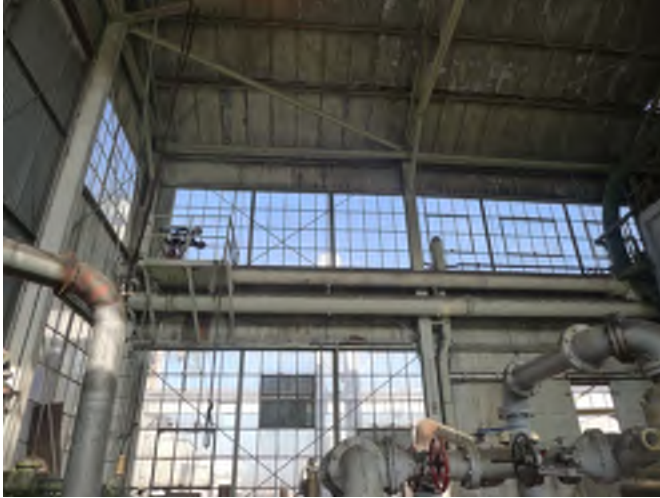
Figure. 12 - Building 103: Interior view
