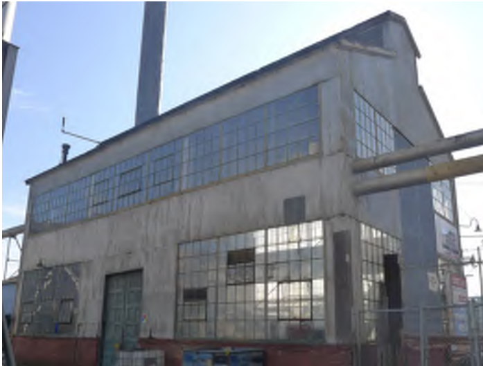
Figure 7 - Building 103: Windows at north & west elevations
