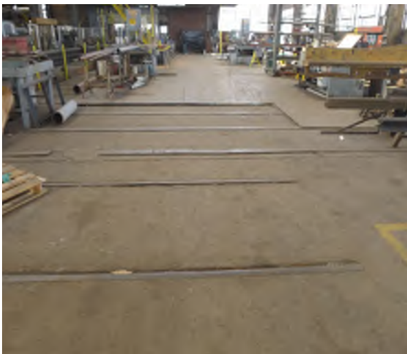
Figure 28 - Interior main shed floor looking west.
