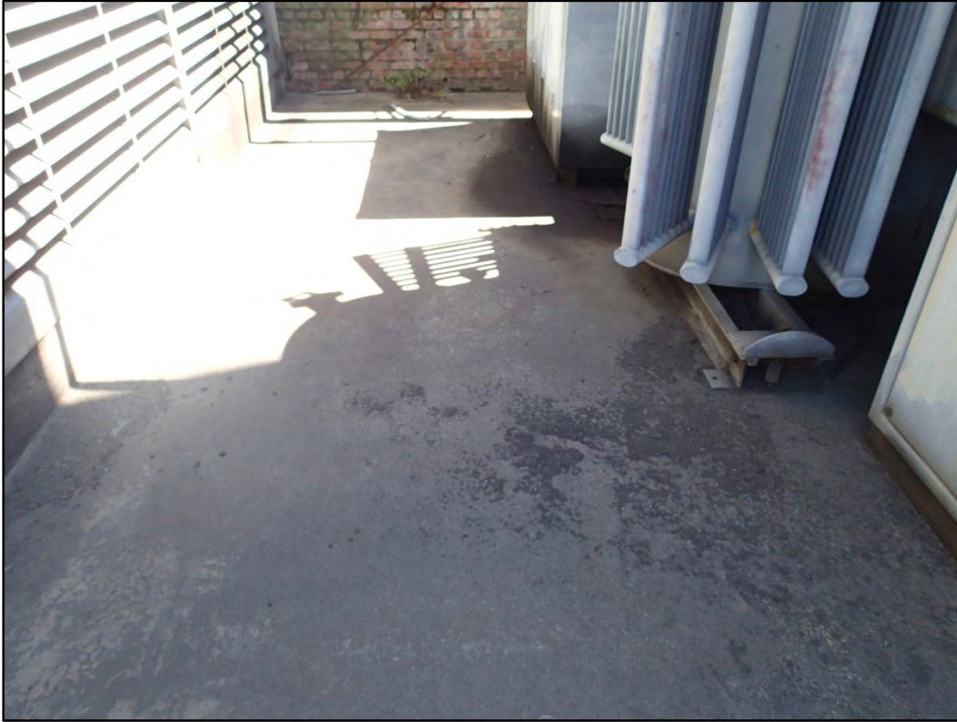
Figure 107-6 – View of Building 107 concrete slab located at the western end.
