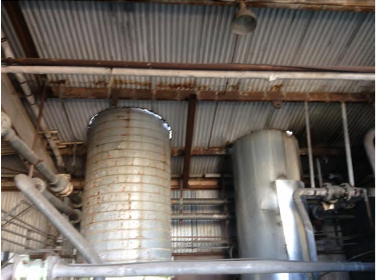
Fig. 1 - Building 107 view from interior.
