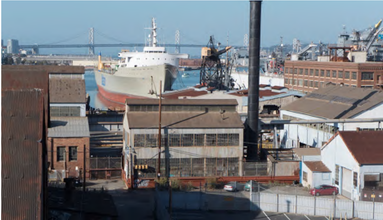
Figure 1 - Building 103, view from south
