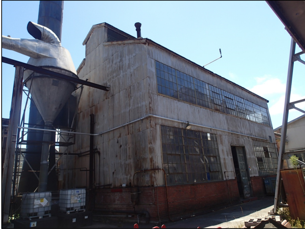
Figure 103-2 – Overall northeast view of Building 103.
