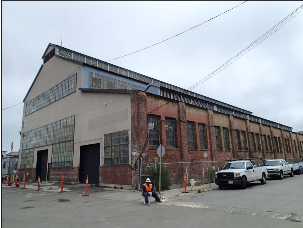
Figure 105-2 – Overall southwest view of Building 105.
