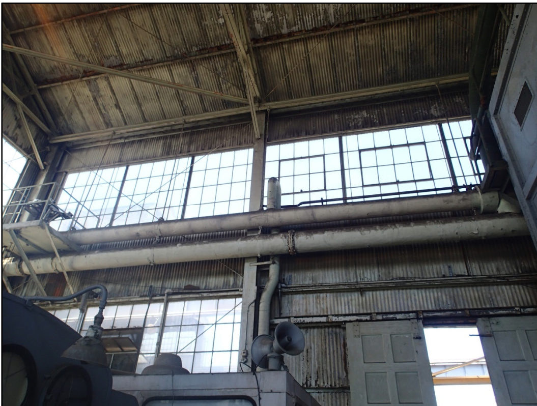
Figure 103-8 – View of Building 103 typical interior wall corrugated metal panels.
