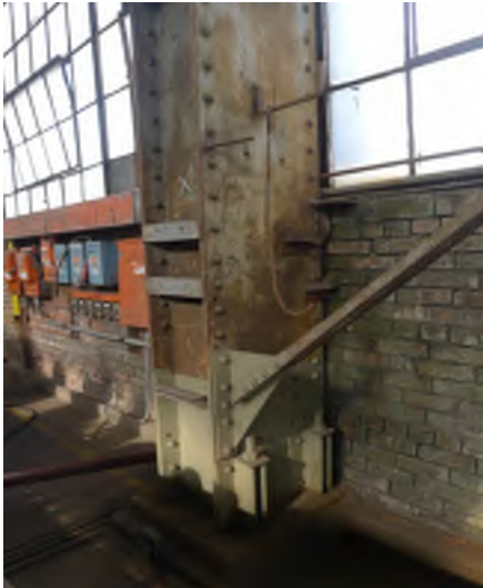
Figure 32 – Main shed north wall column
