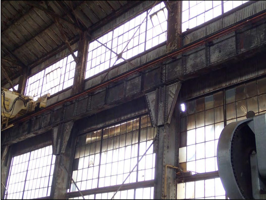
Figure 105-8 – View of Building 105 interior structure and wall corrugated metal panels.
