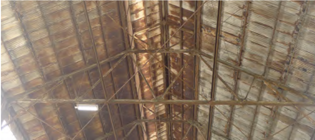
Figure 31 - Main shed truss
