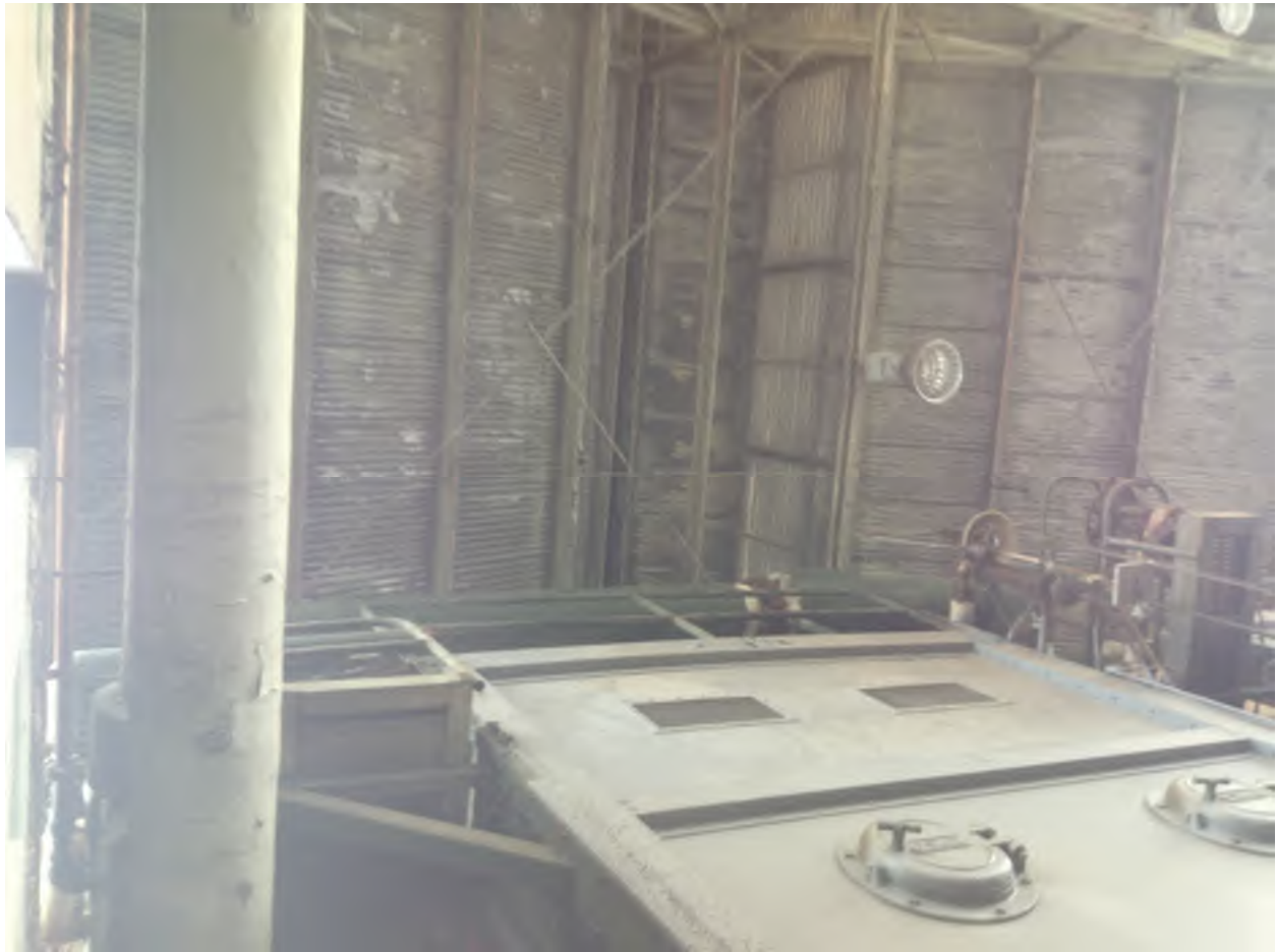
Fig. 1 - Building 103 view from fixed building ladder
