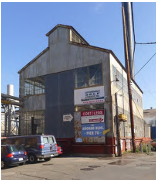
Figure 3 - Building 103: West Elevation
