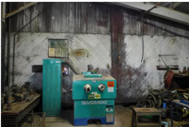
Figure 5 - Building 107: Interior wood wall.
