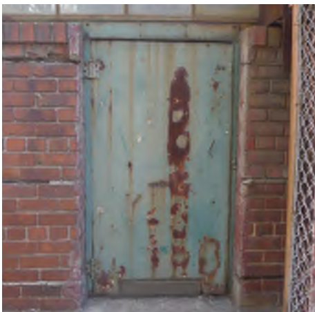
Figure 10 - Building 103: Fire door
