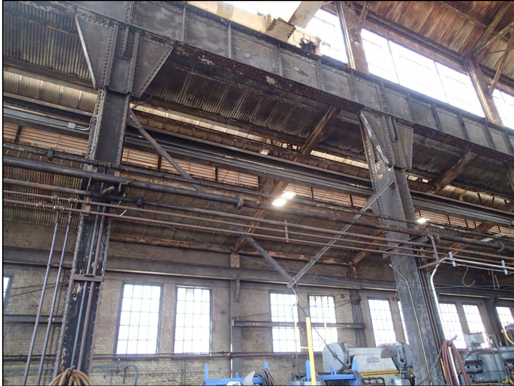
Figure 105-10 – View of Building 105 cut interior braced frames.
