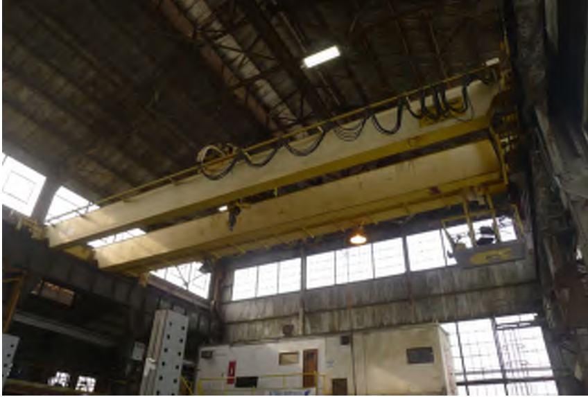
Figure 34 – Main shed, overhead rolling crane on tracks.
