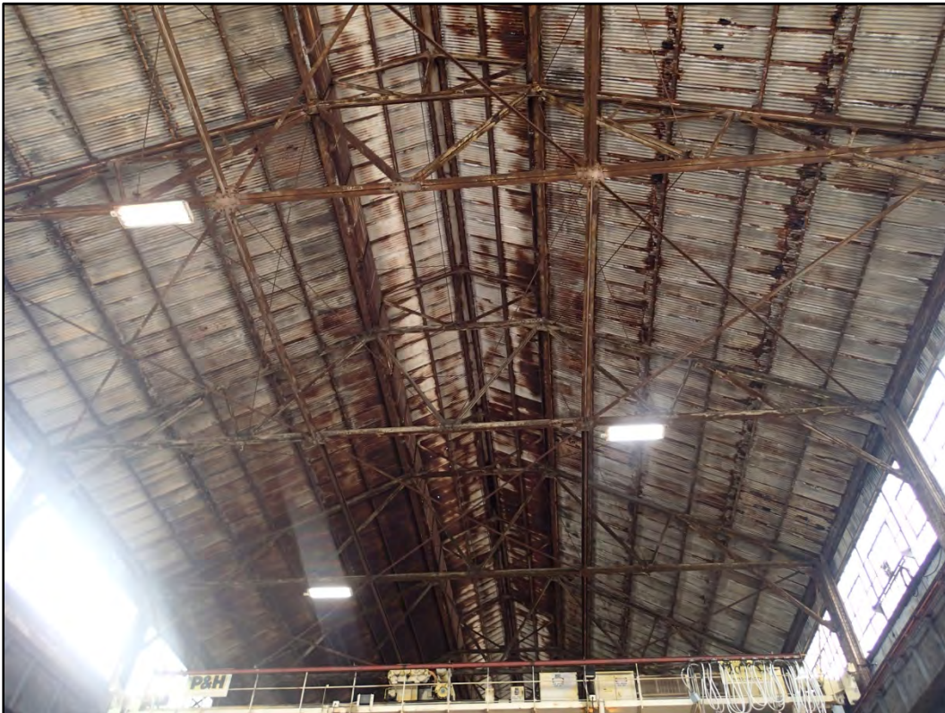
Figure 105-9 – View of Building 105 roof structure and corrugated metal panels
