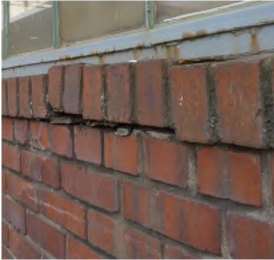
Figure 8 - North wall, detail, displaced bricks at sill
