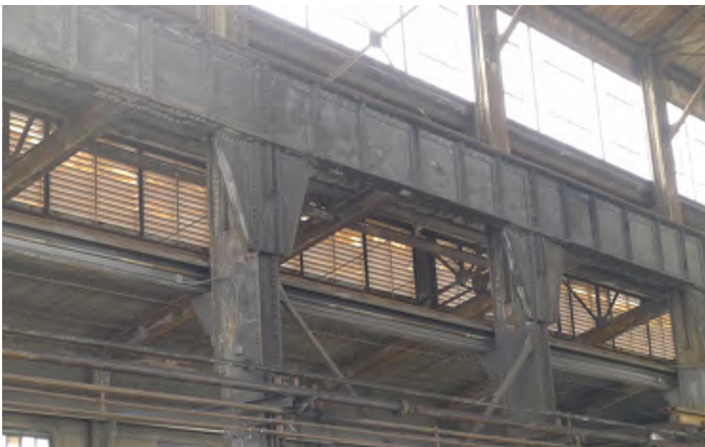
Figure 30 - Structure of main shed looking into south shed
