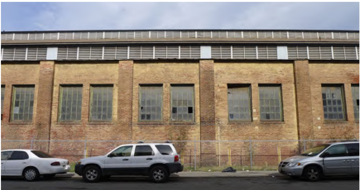
Figure 9 - South wall, typical view of bays.
