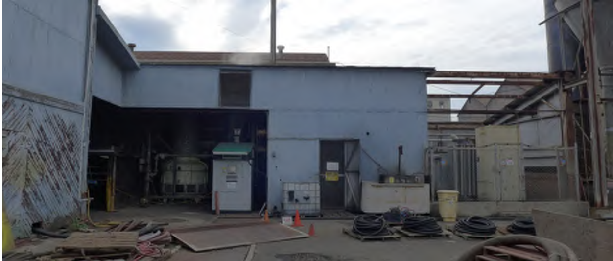
Figure 1 - Building 107, view from north
