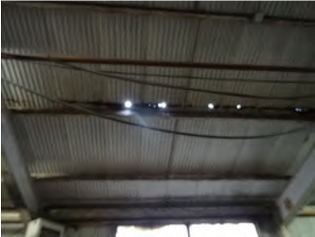
Figure 5 – Typical CMP corrosion with rust holes
