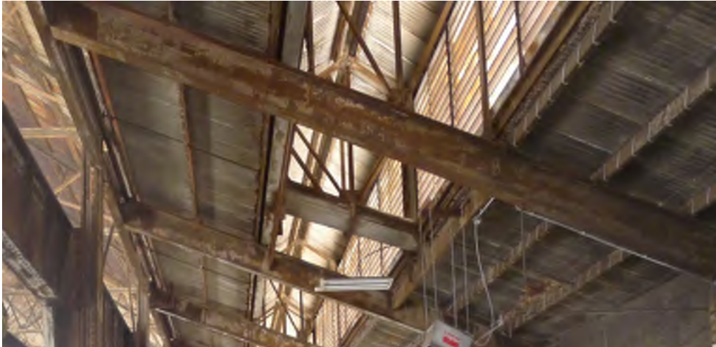
Figure 31 - Rolled steel spanning sections in the south shed.
