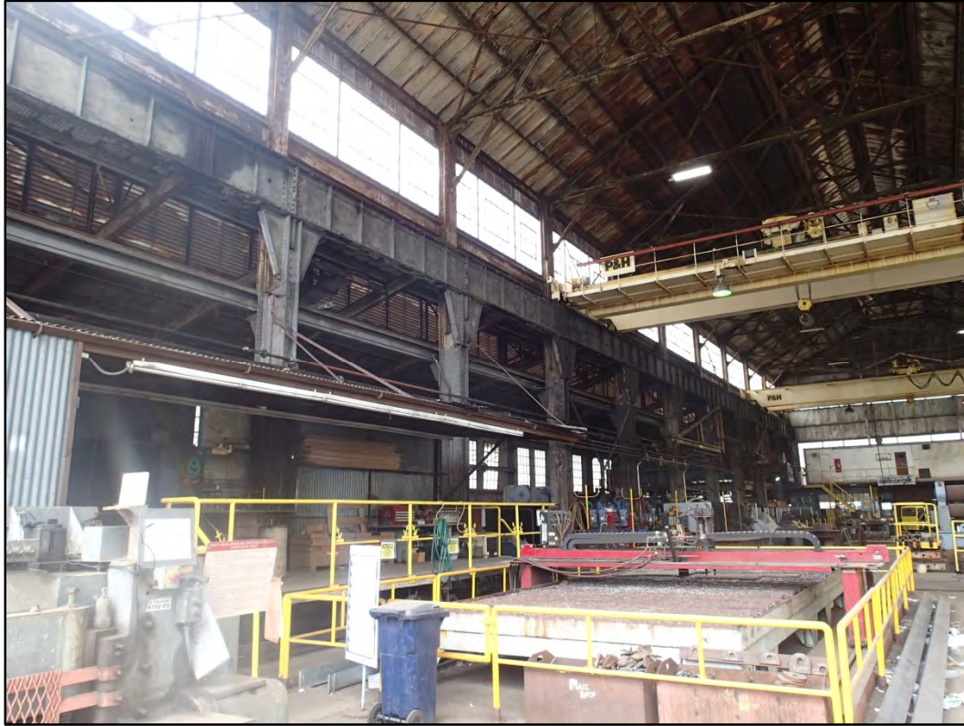
Figure 105-6 – Overall view of Building 105 interior, looking southwest.
