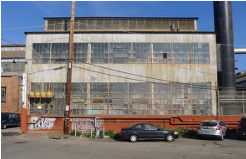
Figure 2 - Building 103: South Elevation
