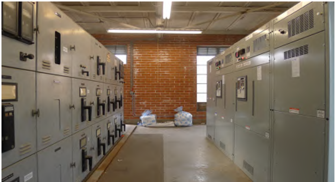
Figure. 15 - Building 68: Interior view
