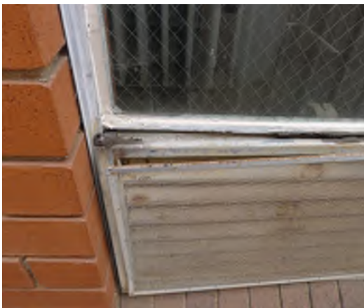
Figure 10 - damaged louver
