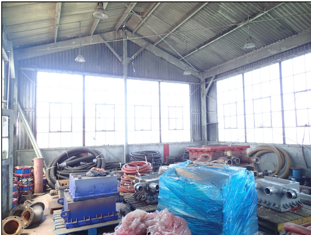
Figure 58-5 - Overall view of Building 58 interior, looking northwest.
