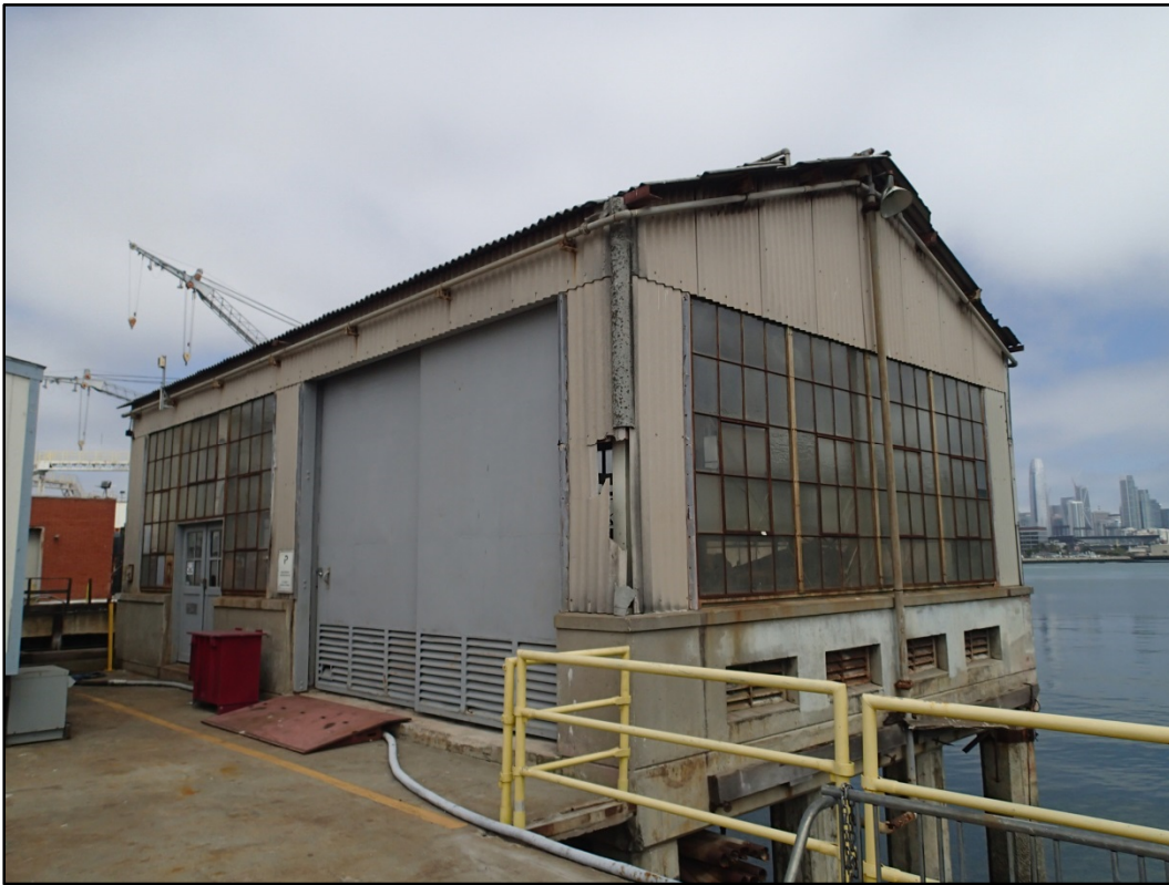
Figure 58-1 - Overall southeast view of Building 58.
