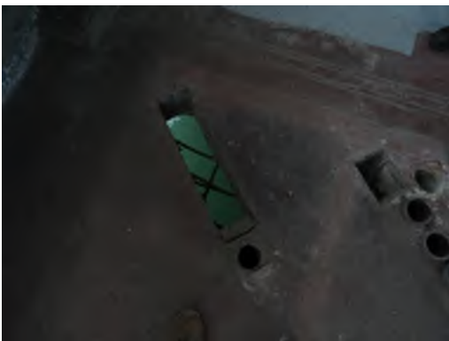
Figure 2 – Building 58 cut holes in slab
