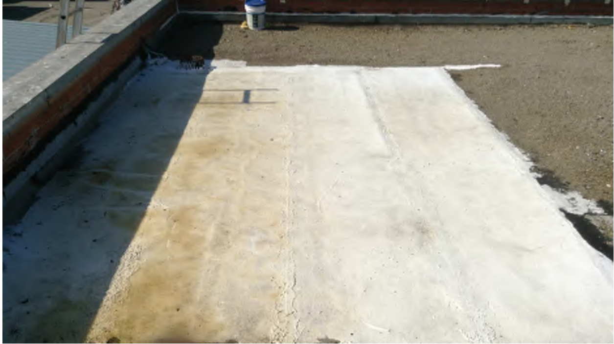
Fig. 1 - Building 68 view from roof top
