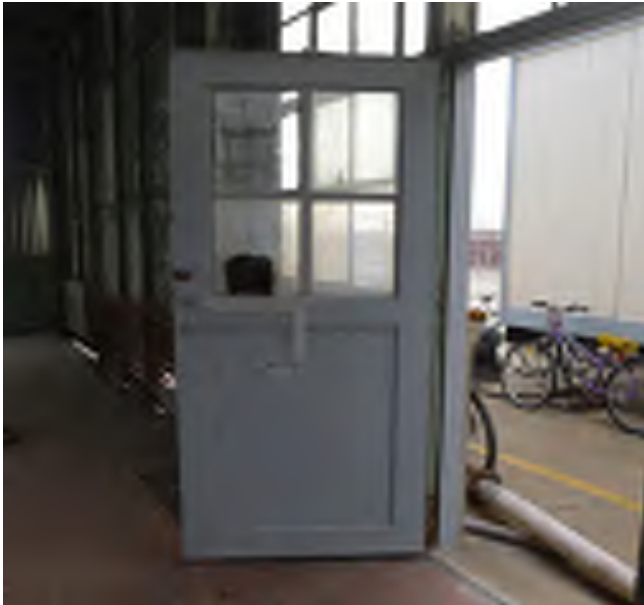
Figure 8 – One leaf of steel personnel door, interior view
