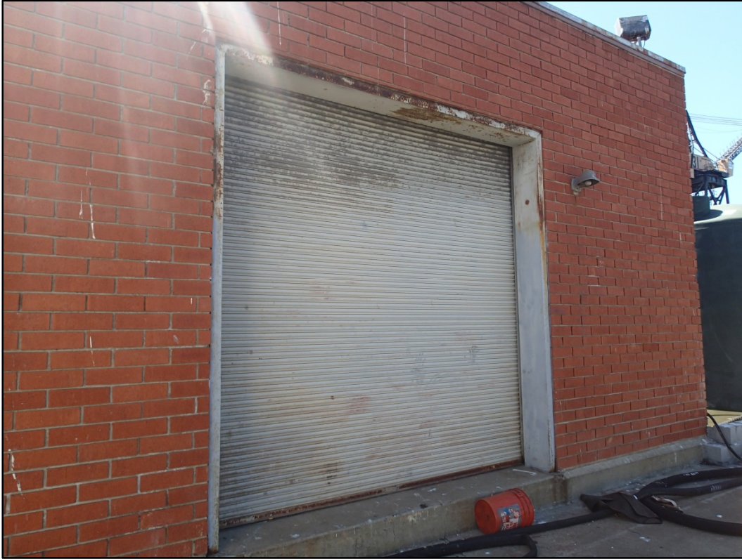
Figure 68-5 –View of Building 68 exterior steel roll-up door.
