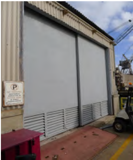
Figure 10 – Sliding door exterior
