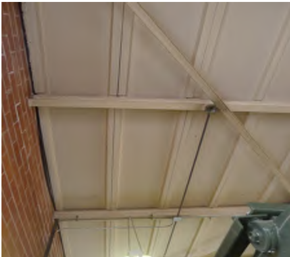
Figure 17 - Painted precast concrete ceiling panels.
