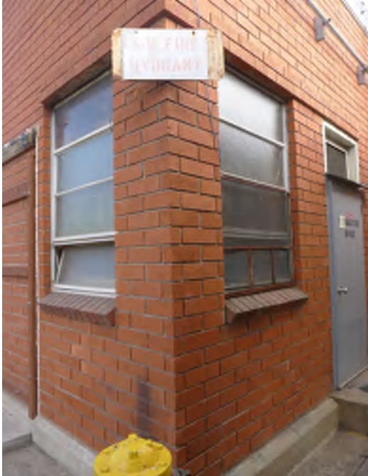
Figure 8 - Aluminum sash. at southwest corner
