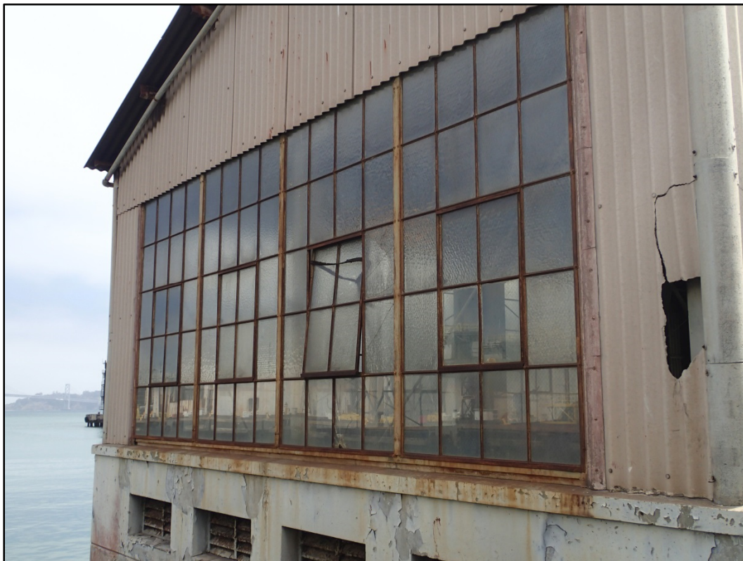
Figure 58-3 - View of Building 58 typical exterior window condition.
