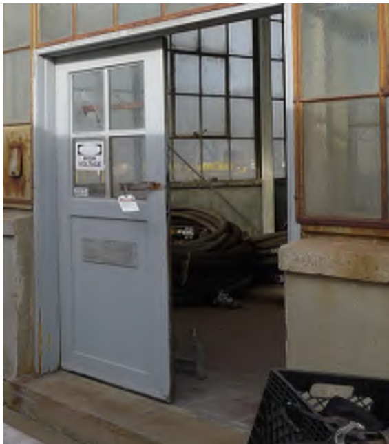
Figure 9 - Steel personnel door, exterior view
