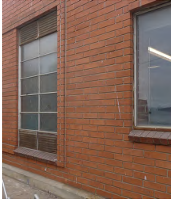
Figure 9 - Steel sash with louvers (left) and plate glass window (right), west elevation
