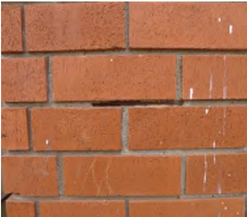
Figure 7 - Masonry joint with exposed rebar
