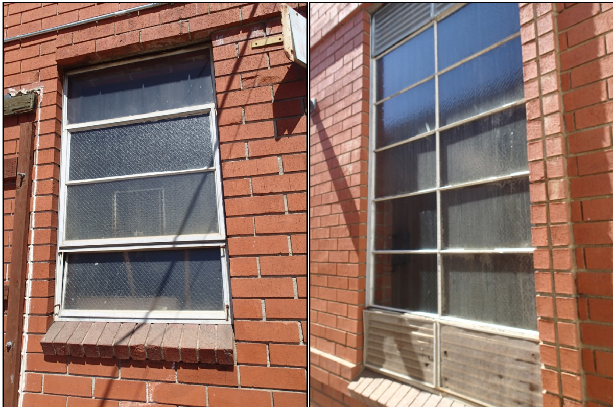
Figure 68-3 & Figure 68-4 - View of Building 68 typical exterior window condition.
