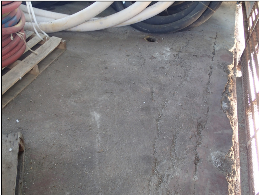
Figure 58-7 - View Building 58 interior concrete slab.
