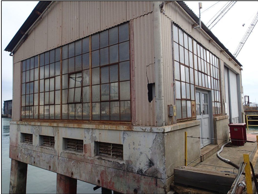
Figure 58-2 – Overall southwest view of Building 58.
