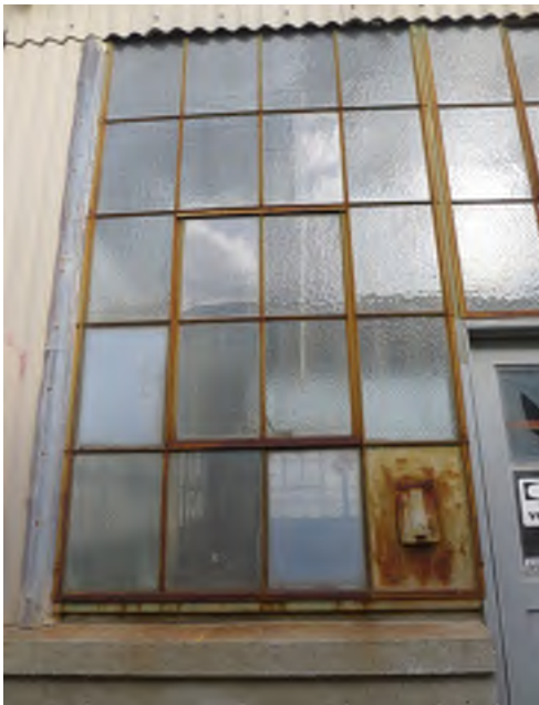
Figure 6 - Window at south elevation
