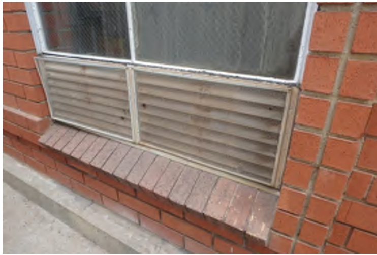
Figure 68-1 – Building Windows w/ Louvers
