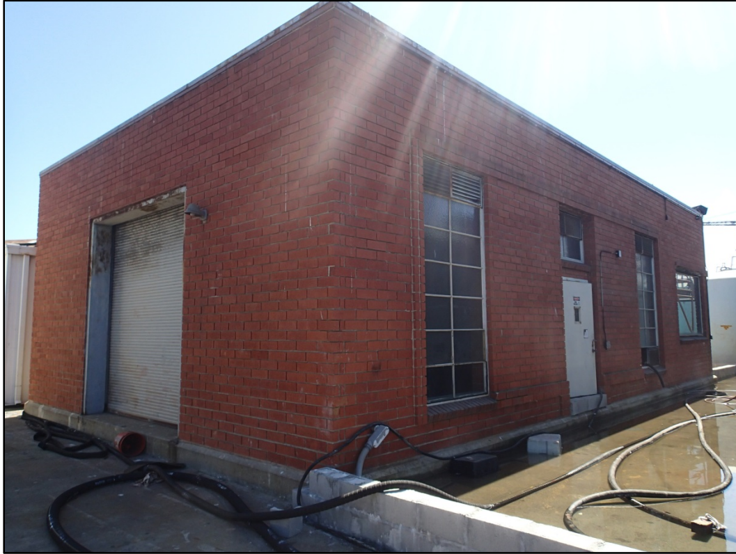
Figure 68-2 – Overall northeast view of Building 68.
