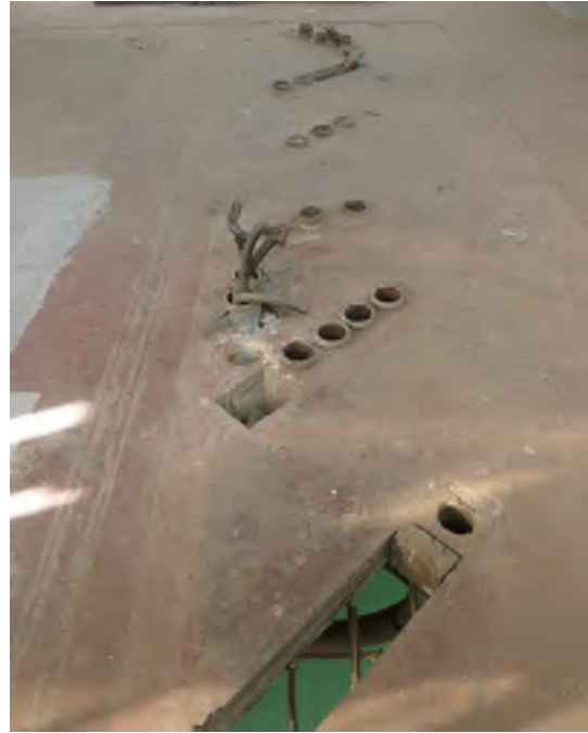
Figure. 14 - Interior view floor with penetrations
