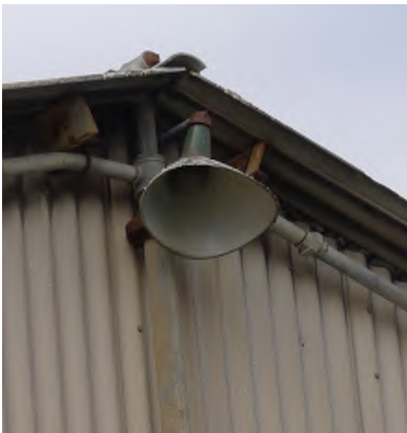
Figure 12 - Lamp at ridge, east elevation
