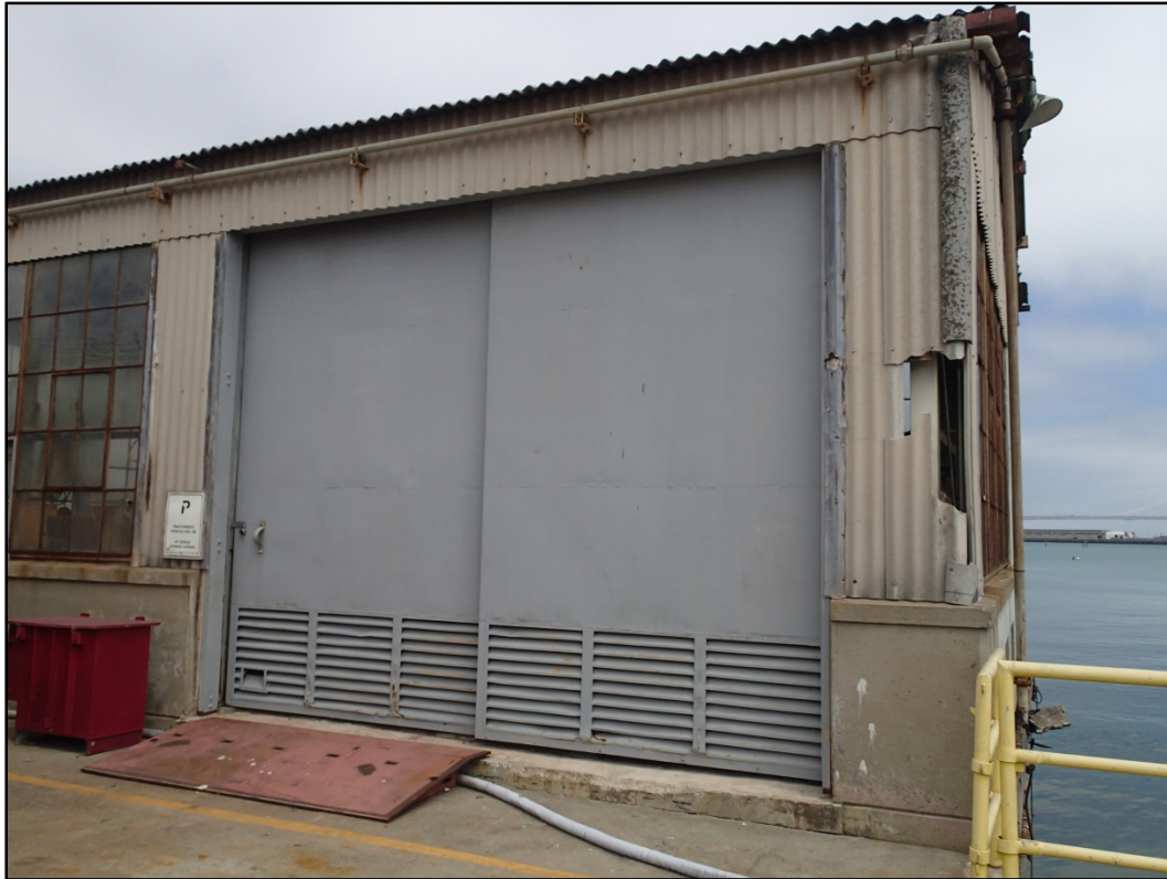
Figure 58-4 –View of Building 58 exterior steel sliding door.
