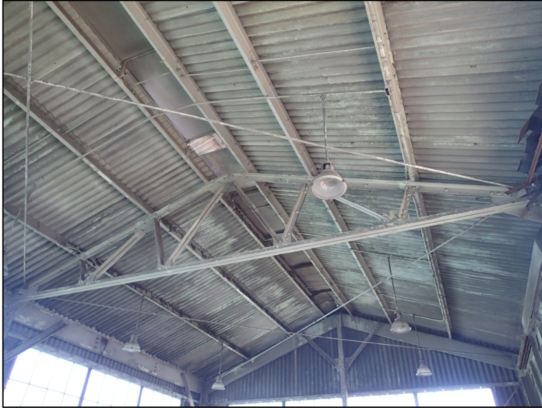
Figure 58-6 – View of Building 58 roof structure and corrugated transite panels.
