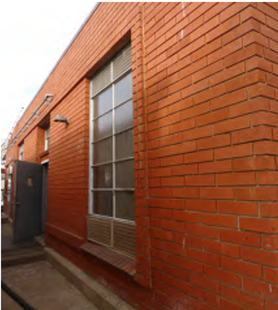
Figure 6 - Brick band detail at windows
