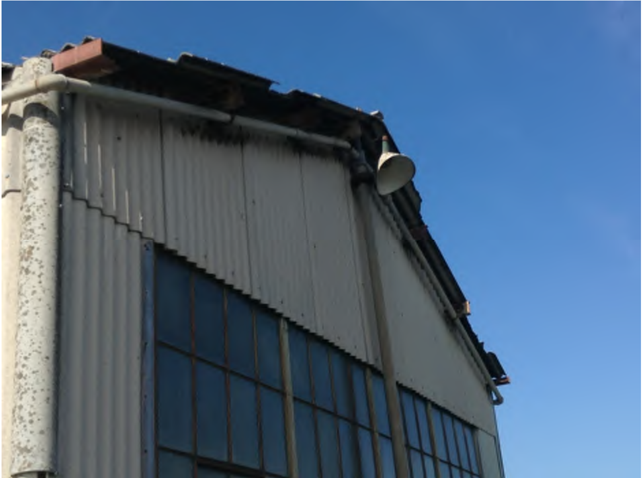
Fig. 1 - Building 58 view from ground at S. E. corner
