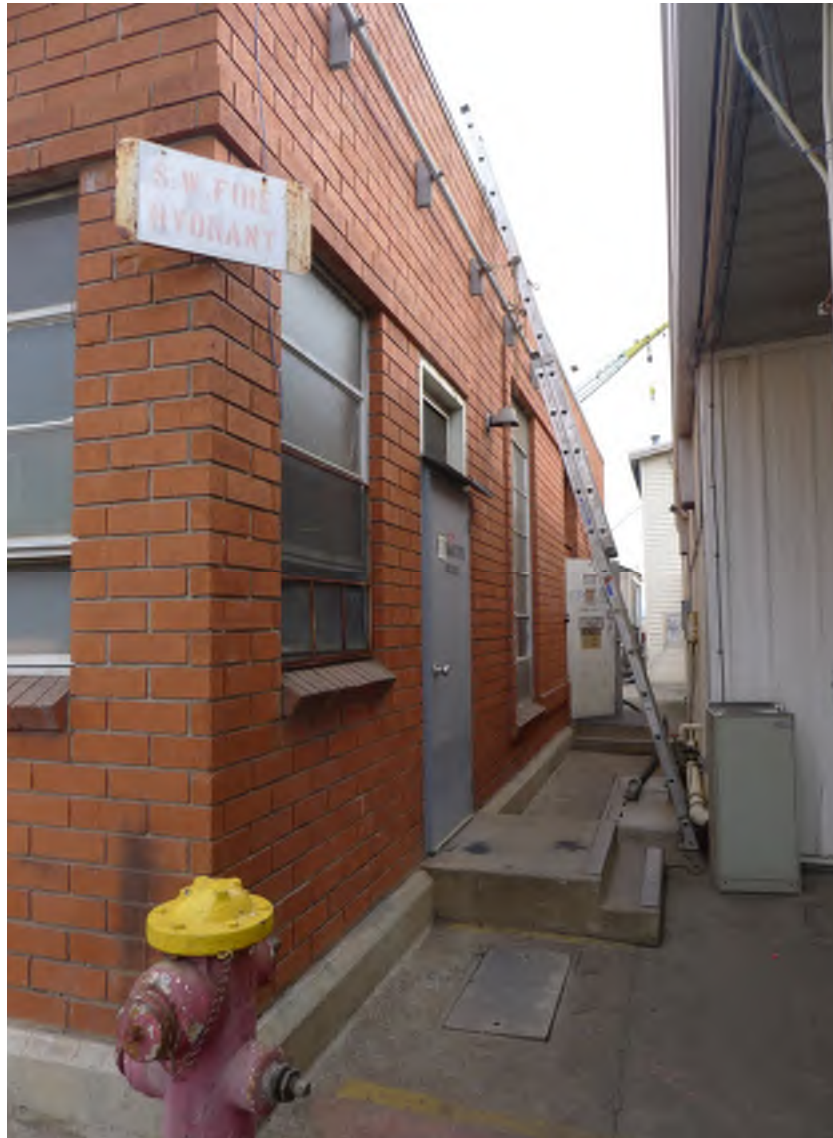
Figure 1 - Building 68, South elevation
