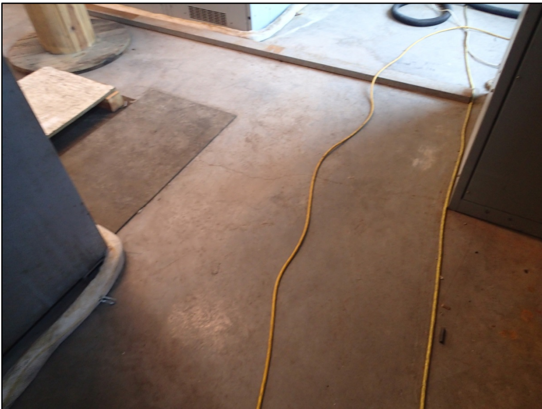
Figure 68-8 - View of Building 68 interior concrete slab.
