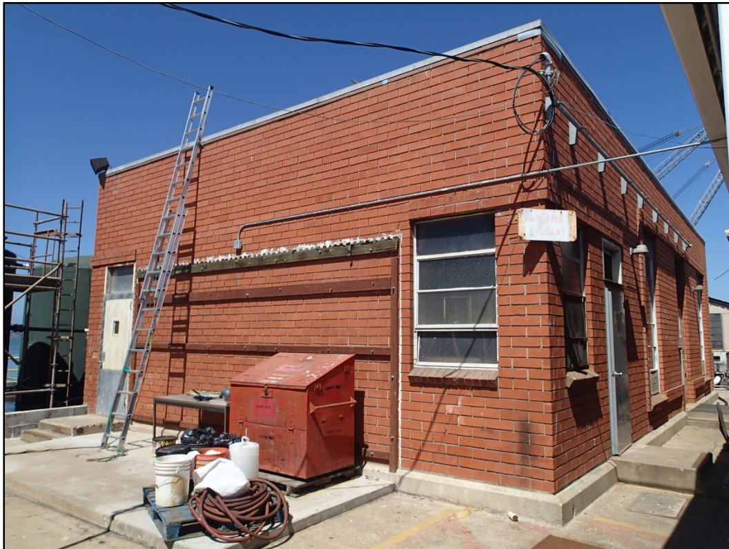
Figure 68-1 - Overall southwest view of Building 68.
