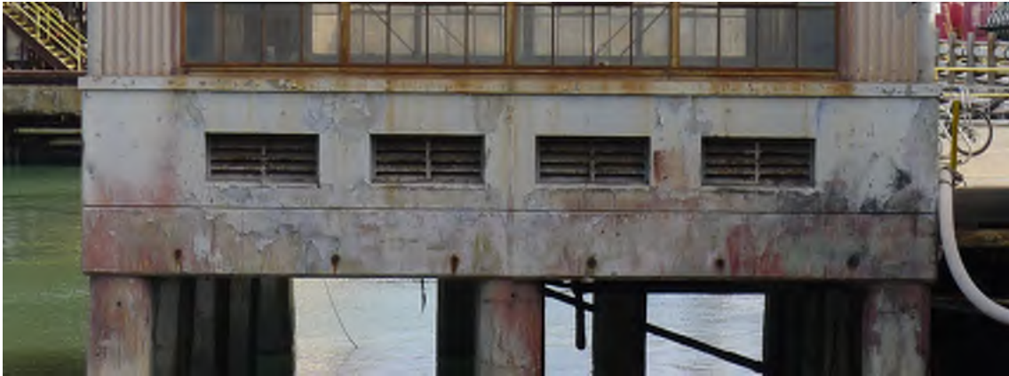
Figure 5 – Concrete stem wall showing penetrations with ventilation louvers
