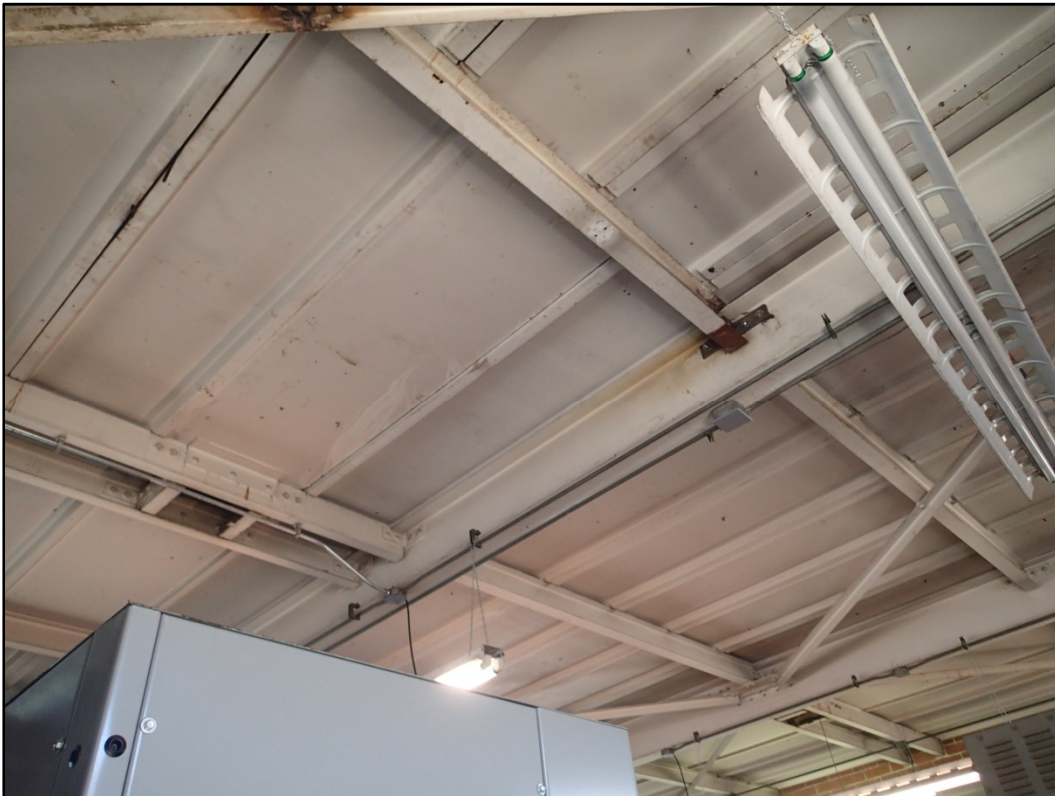
Figure 68-6 – View of Building 68 roof structure and painted ceiling panels.
