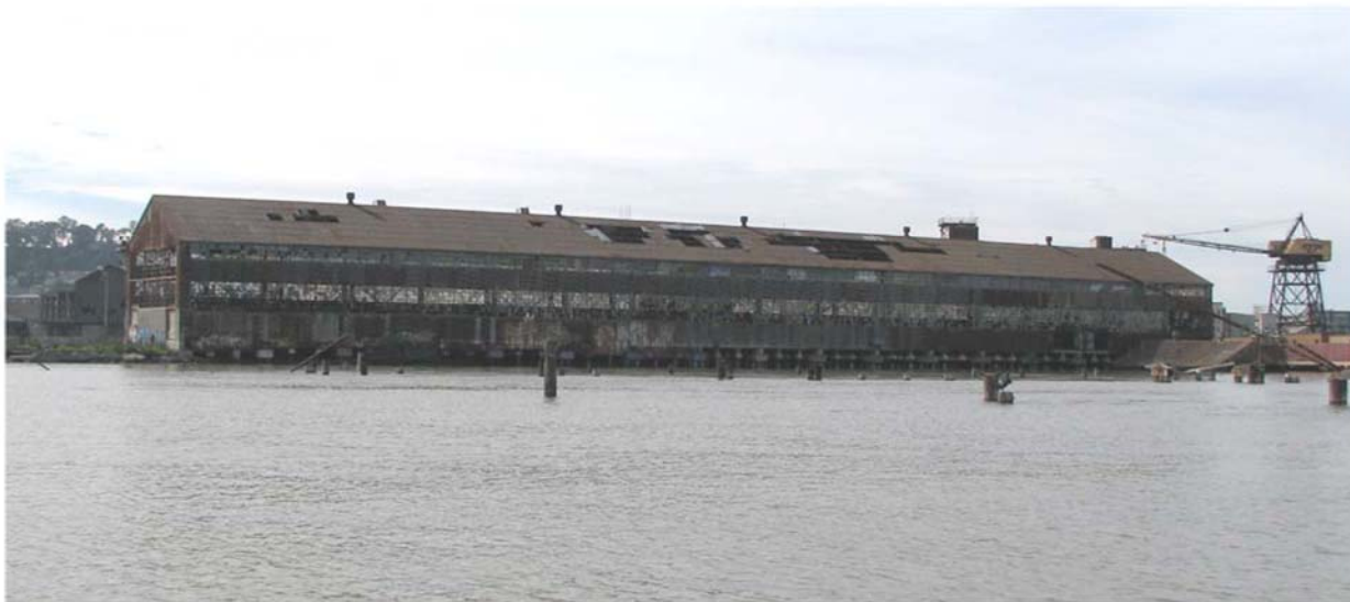
Figure 1 Pier 70 Building 6 as seen from the water looking west.
