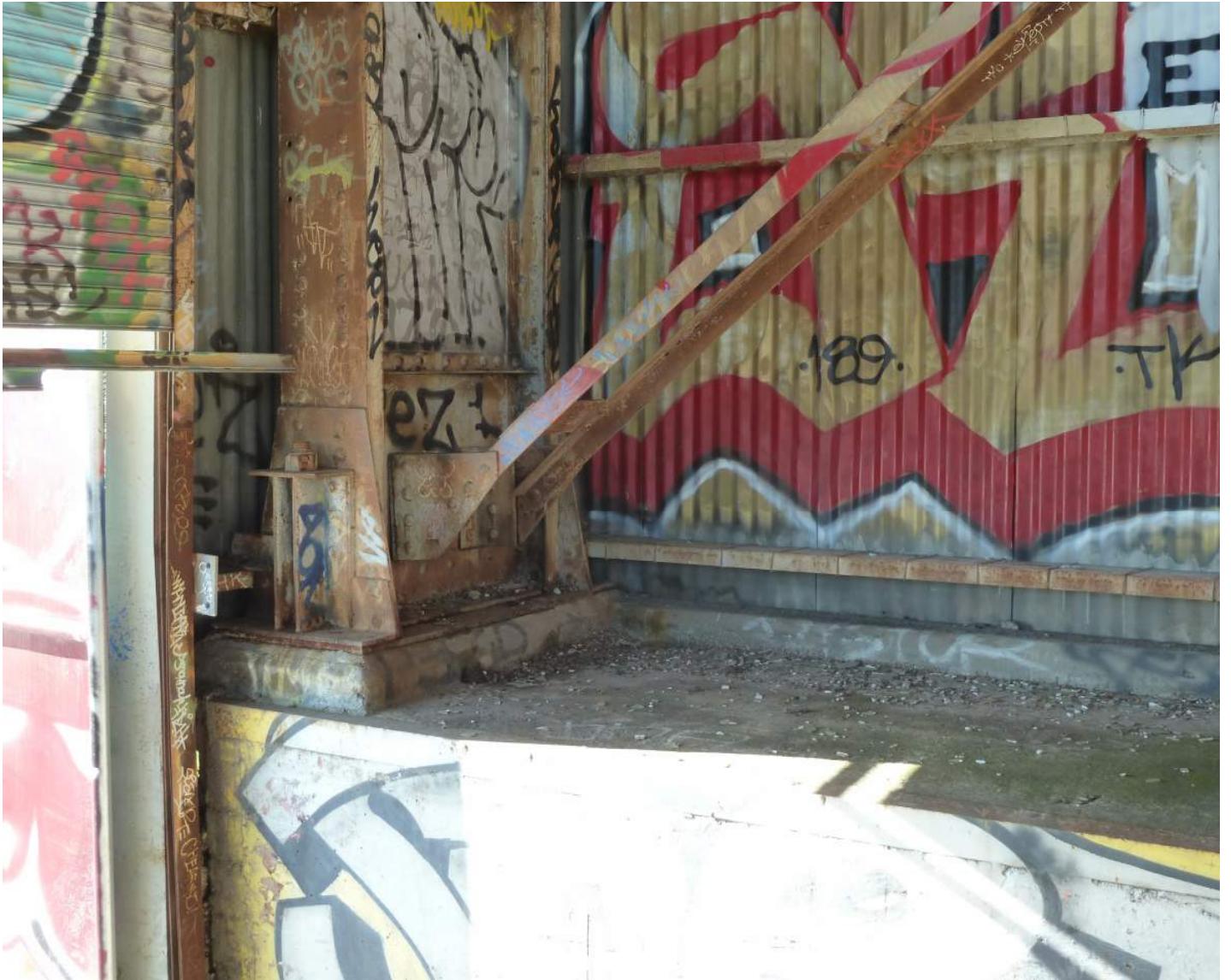
IMAGE 6: Typical Brace to Column Connection
