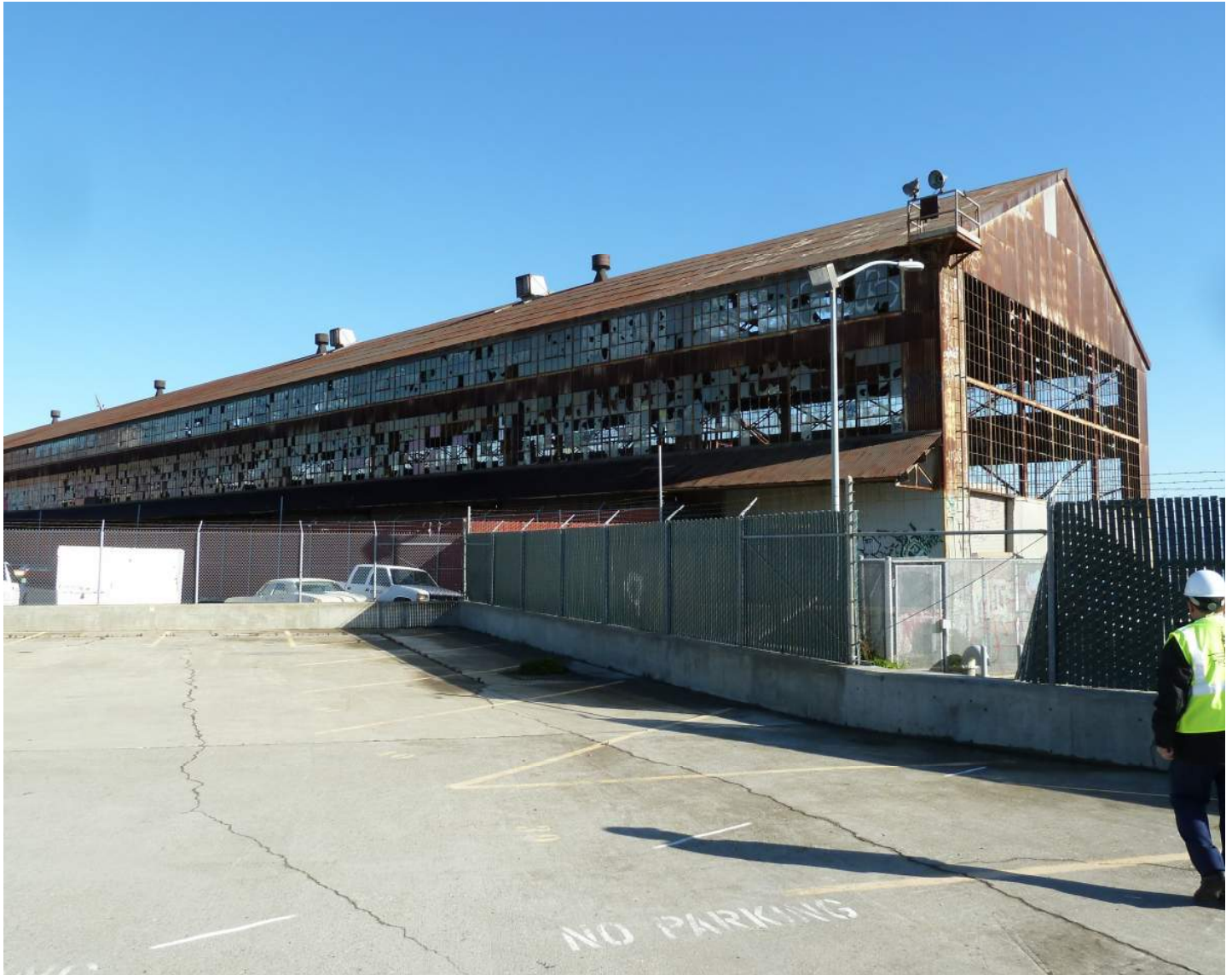
IMAGE 1: EXTERIOR VIEW OF BUILDING 6 LOOKING NORTH
