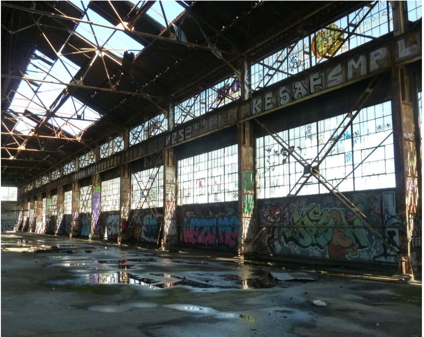
IMAGE 4: "X"-Brace at Every Other Bay at East Face
