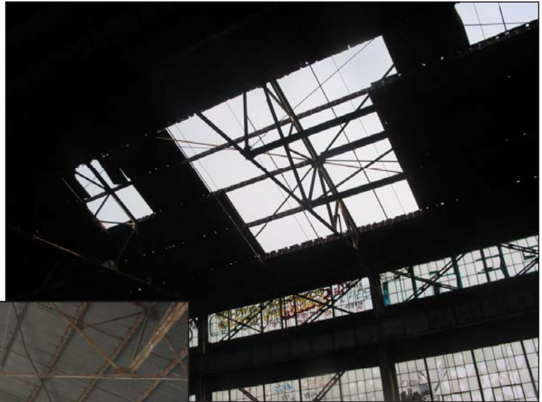
Photo 5 Above: Deteriorated Roof Framing
