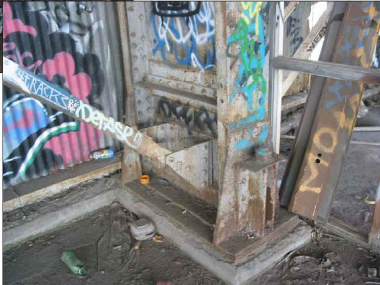
Photo 4 Below: Brace Connection at Column Base
