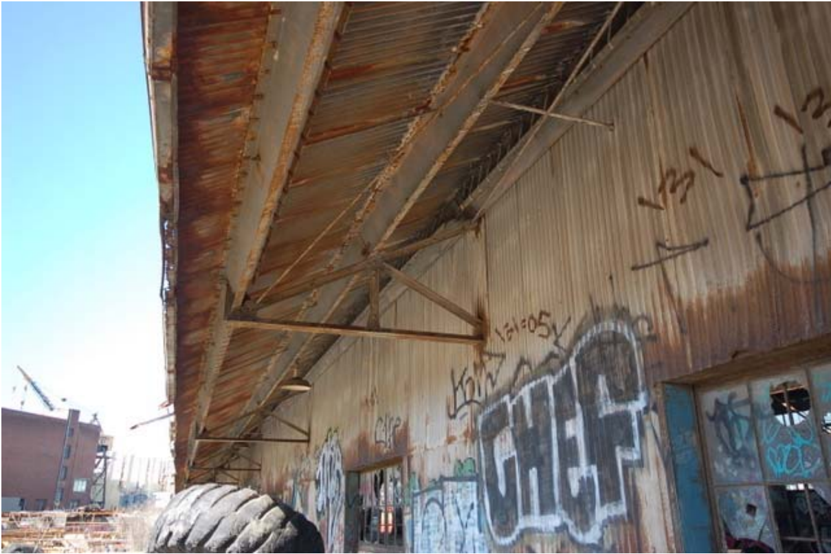
Figure 5: South wall, overhang
