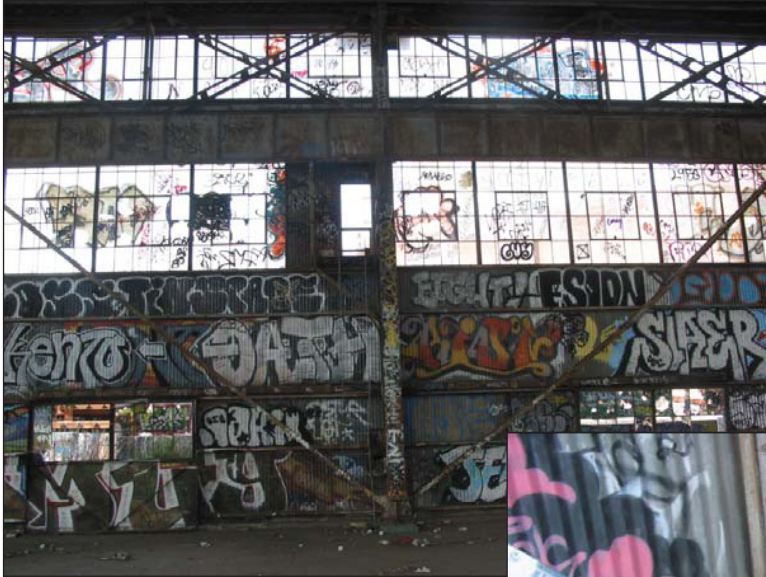
Photo 3 Above: Brace Frame at North Side
