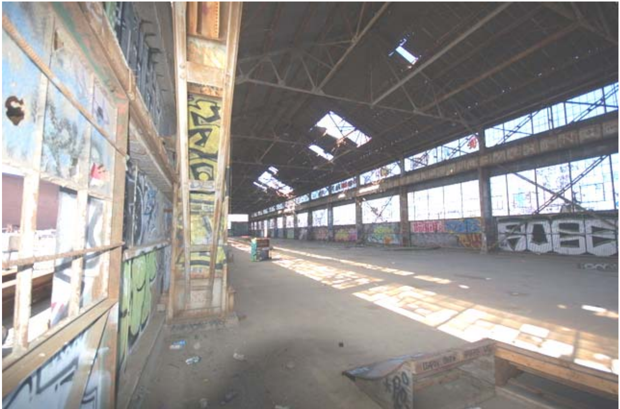
Figure 4: Interior, looking west
