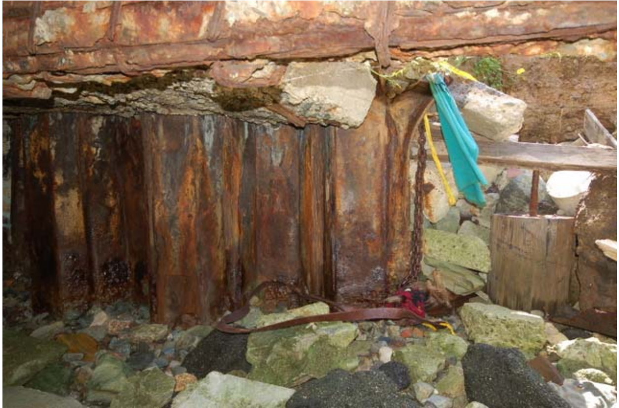
Figure 7: Damaged seawall
