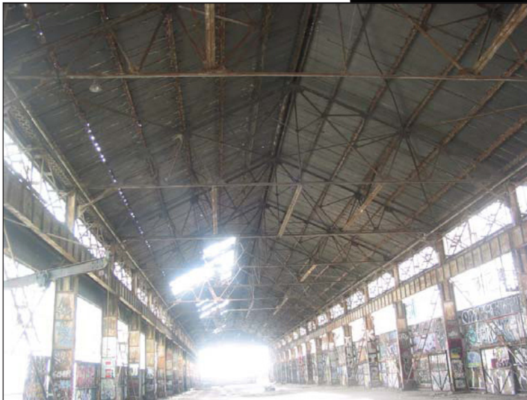
Photo 6 Below: Roof Truss and Metal Deck
