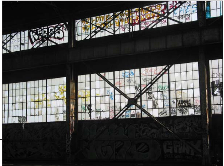
Photo 2 Above: Brace Frame at South Side
