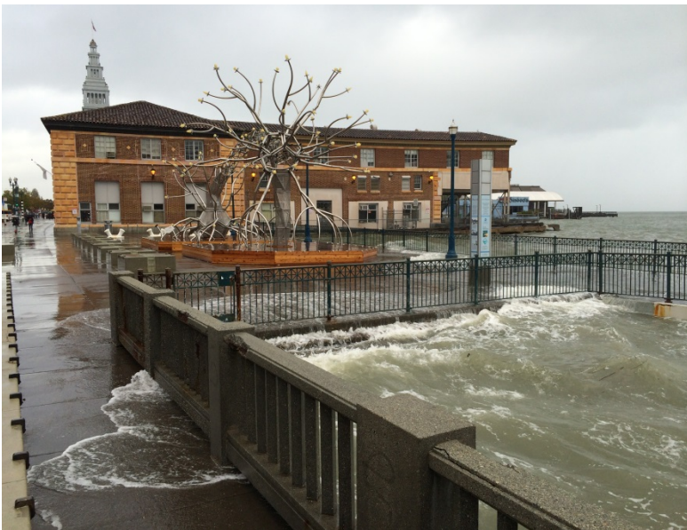
Figure 5: Flooding along Embarcadero during a king tide
