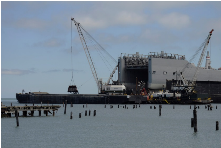
Figure 19: Prior dredging of Central Basin
