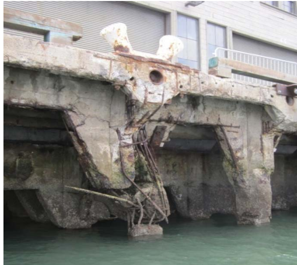
Figure 4: Pier 35 apron—scheduled for repair by the Port's new cement pile repair crew
