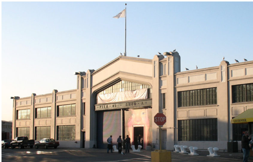
The Port made seismic repairs to Pier 45 to create a modern commercial fish processing center.
