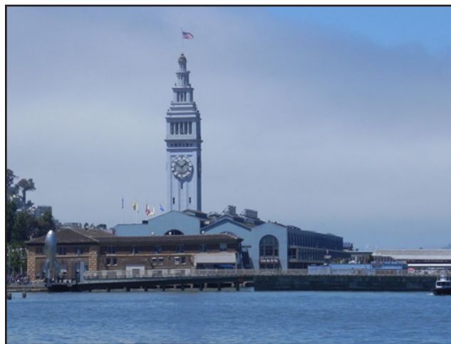
Ferry Building Restoration
