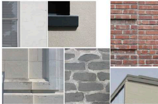
Materials - "... brick ... concrete ... stucco ... metal ..."
