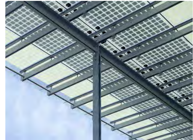
Photovoltaic Canopy Example
