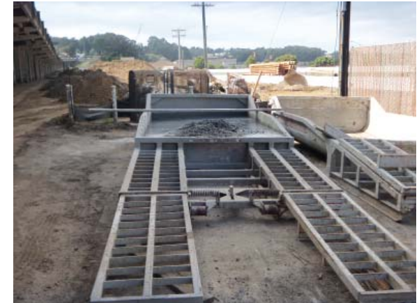
Runoff from the curing operation is captured in a concrete washout.
