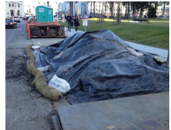
Asphalt debris is escaping from this poorly installed stockpile. Asphalt can release pollutants like hydrocarbons when not properly contained.
