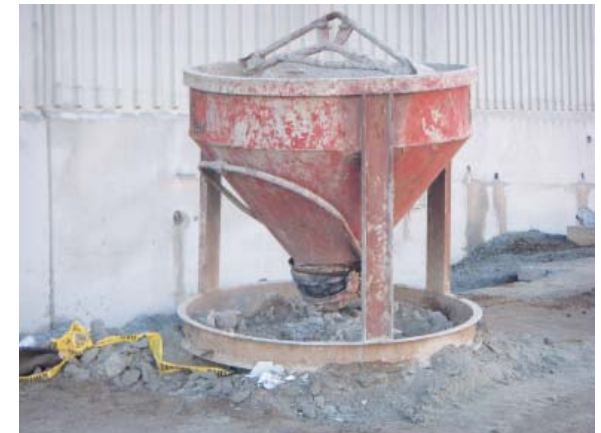
Wastes from concrete curing are not contained, and are open to contact with runoff.
