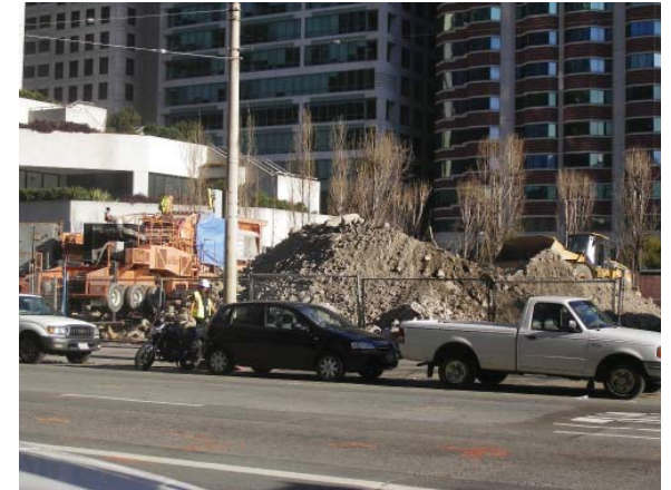
An exposed stockpile is susceptible to dust generation.
