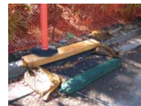
Properly protected inlets
