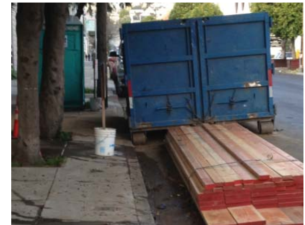
The waste runs into the street allowing pollutants to enter the City storm drain system.
