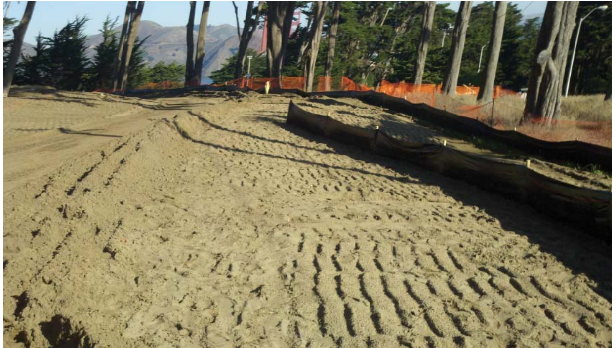
Soil roughening can be used as a complementary process for controlling erosion.
