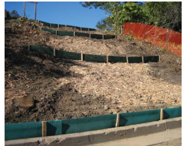
Plastic mesh fencing is installed parallel to the contours along the slope.
