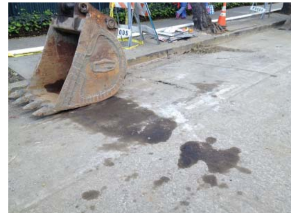
Minor oil spills need to be cleaned to prevent them from running into the storm drain system.
