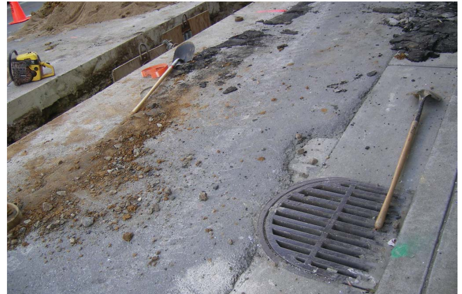
This drain inlet is completely unprotected while construction activities are conducted close by, allowing pollutants to enter the storm drain.
