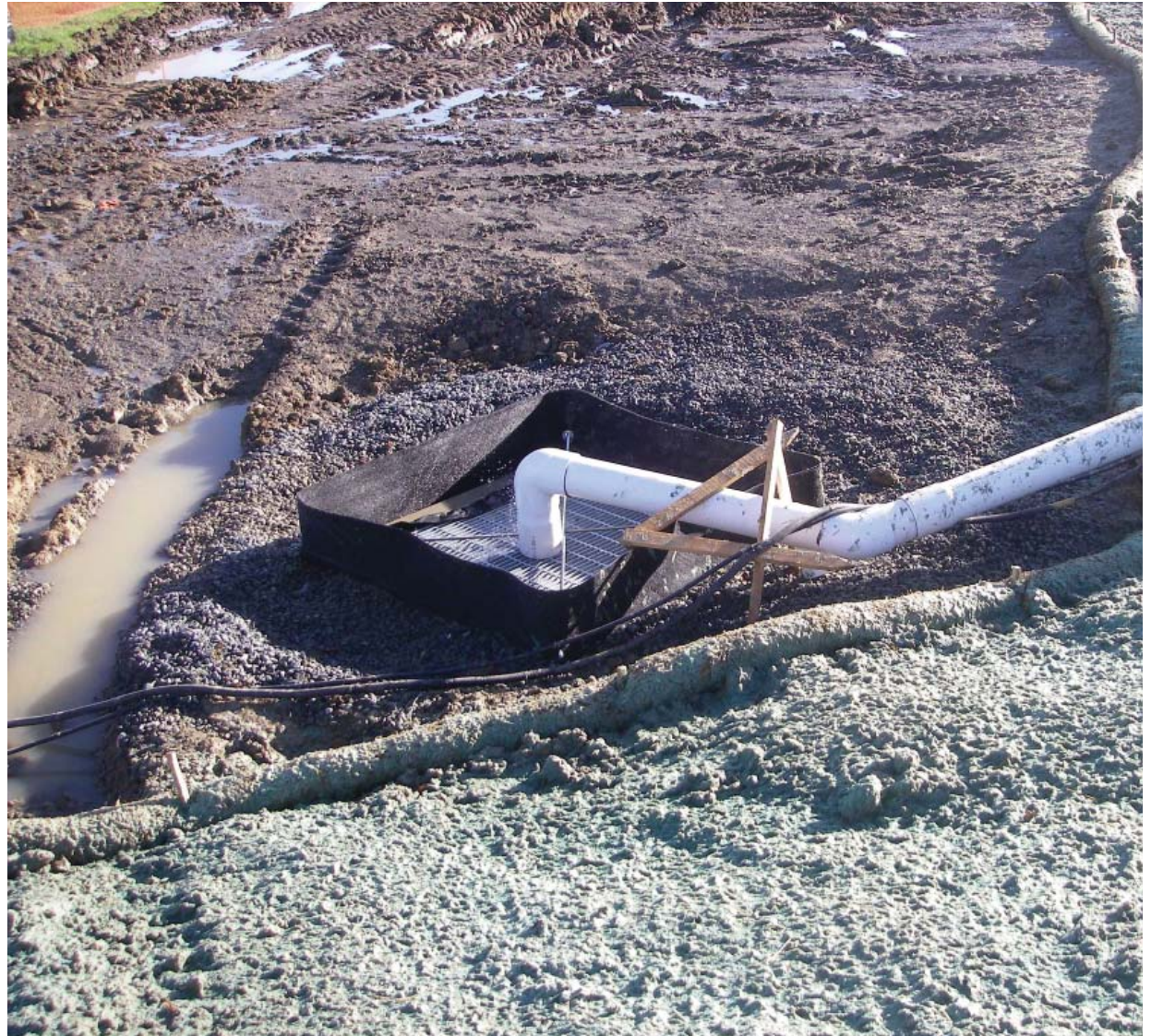
Clean runoff is directed to the storm system through a slope drain. This prevents the runoff from flowing down the steep slope.
