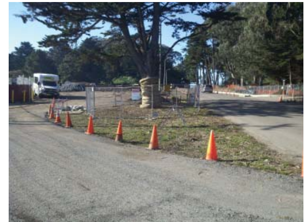
An existing tree is protected with fiber rolls and perimeter fencing.
