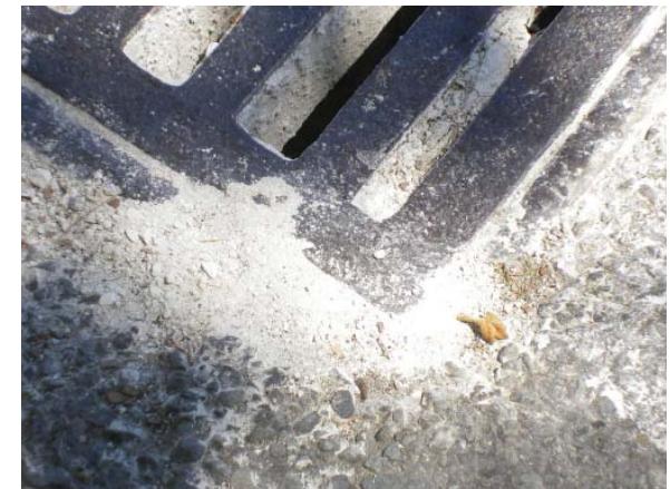
Runoff containing concrete admixtures from unprotected construction activities have made their way to a drainage inlet.
