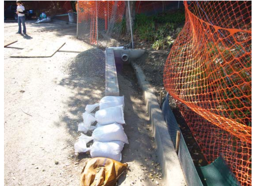
Sediment is allowed to settle out of the runoff. The overflow structure discharges the clean water to the storm system.
