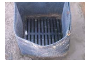
Properly protected inlets
