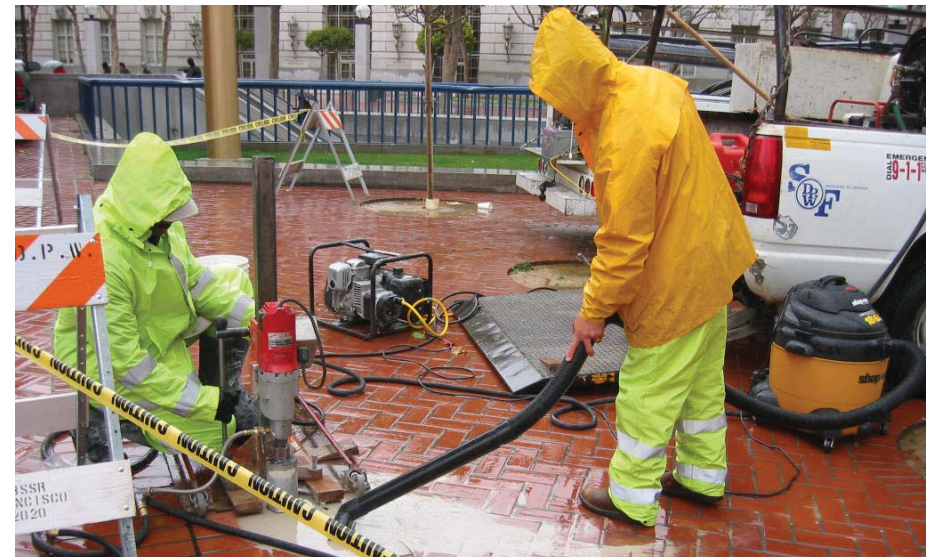
Workers vacuum liquid waste from drilling activities.
