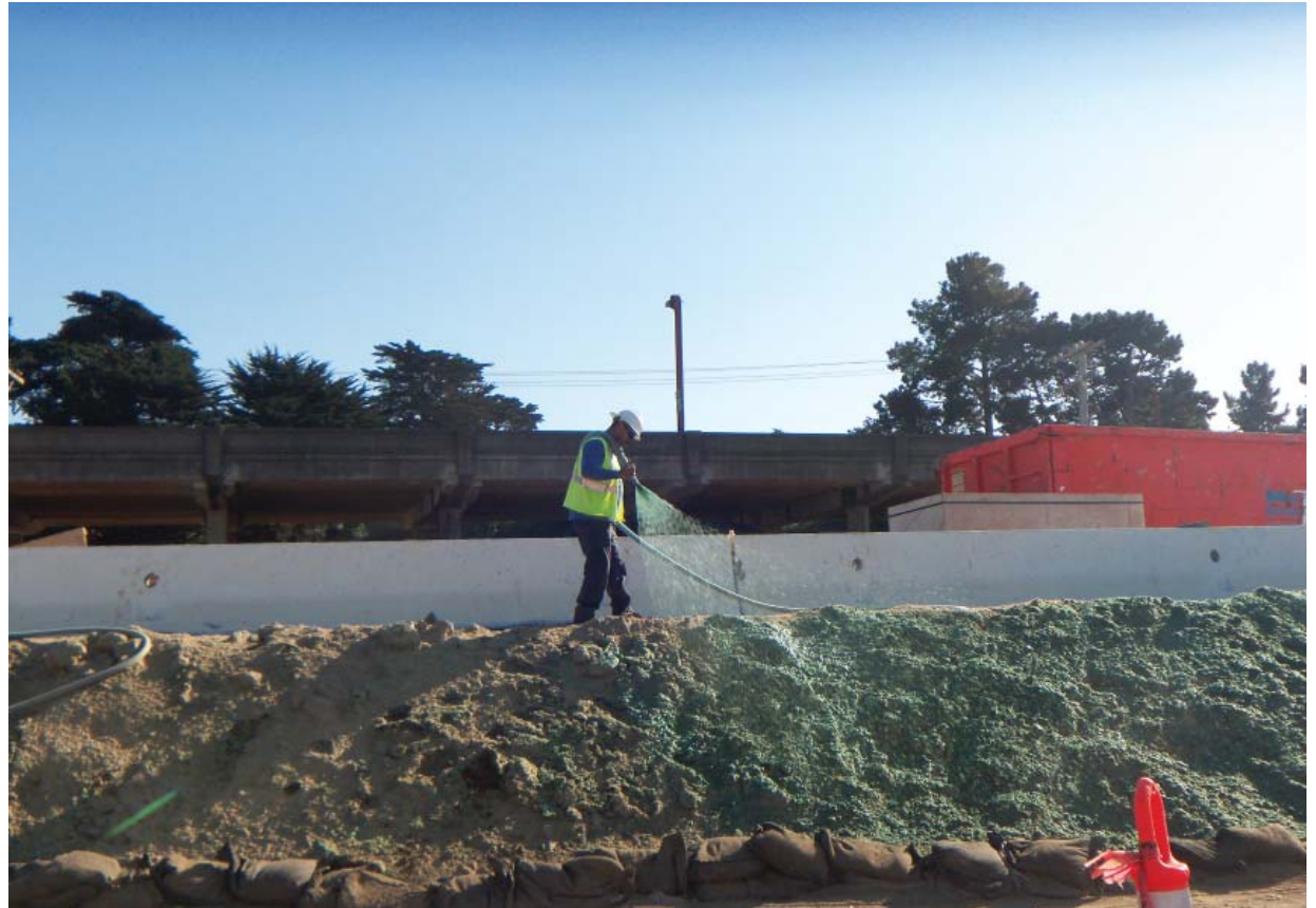
A construction worker is applying a bonded fiber matrix to disturbed soil area.
