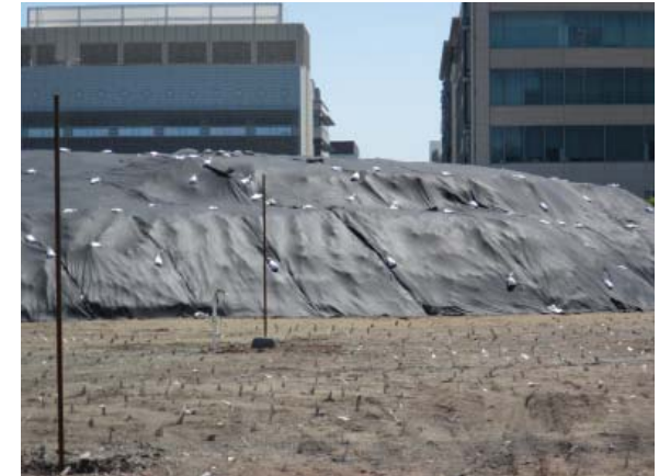
A properly protected stockpile with a plastic cover anchored down by gravel bags.
