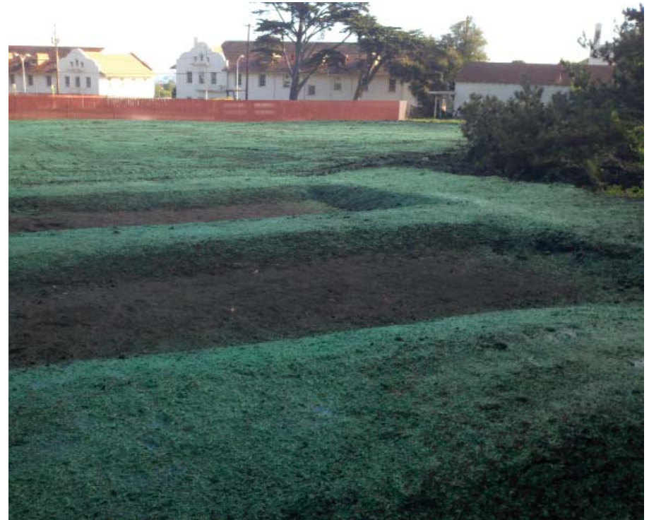
These disturbed soils were stabilized using a bonded fiber matrix.
