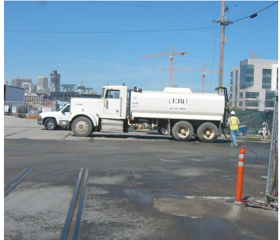
Mud is removed from a delivery truck prior to leaving the site.
