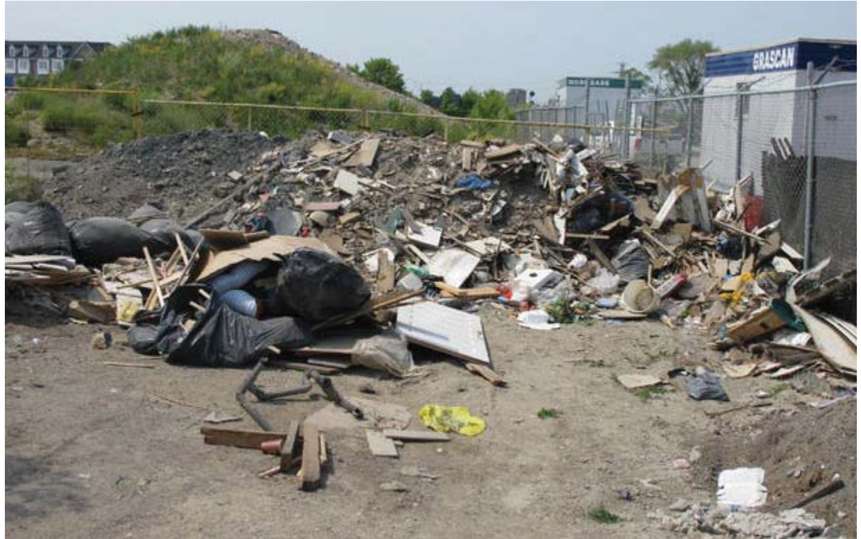
Illegal trash dumping on a construction site.
