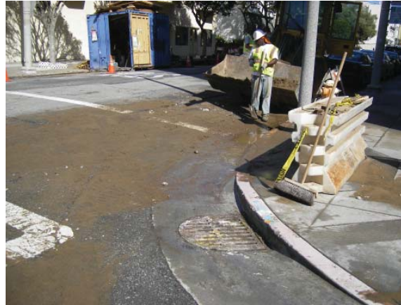
Site violations: unprotected inlet, tracking mud and concrete waste.
