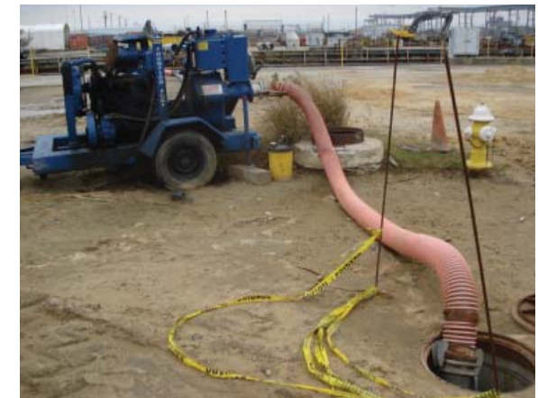
Contractors are illegally pumping unfiltered site runoff directly into the storm system.
