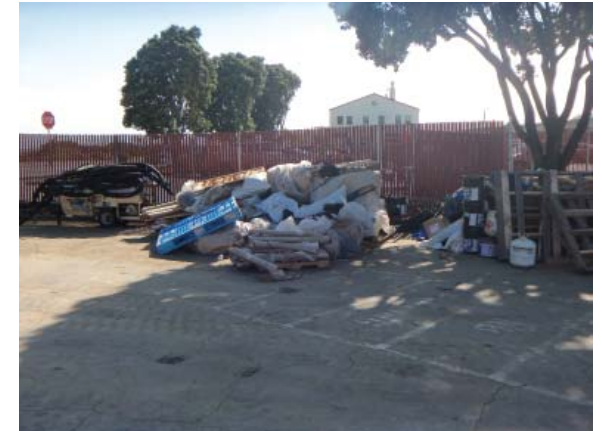
There are no dumpsters, containers or diversion structures to stop stormwater runoff from coming in contact with this construction litter and debris.
