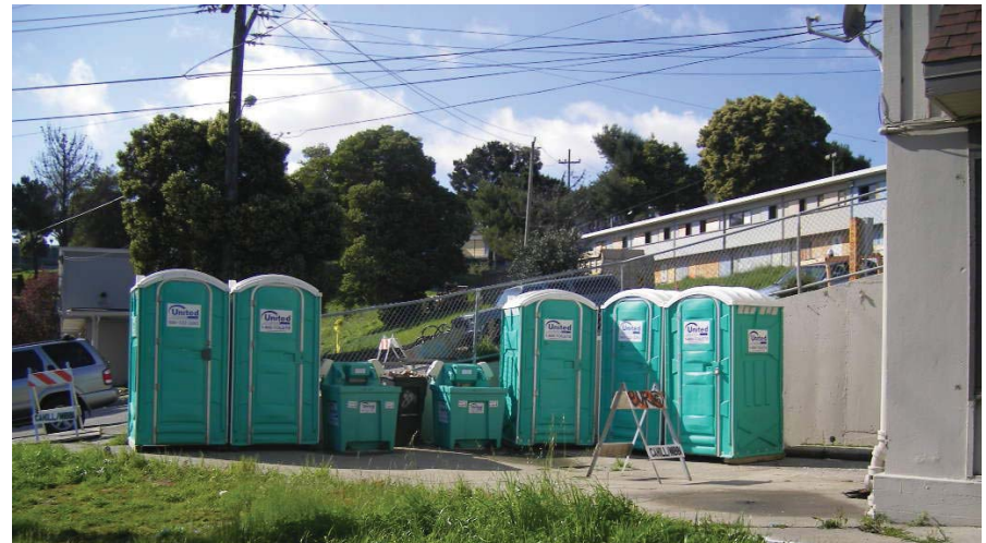
Properly installed portable sanitary facilities.
