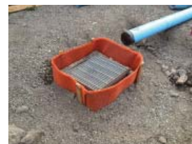
Properly protected inlets
