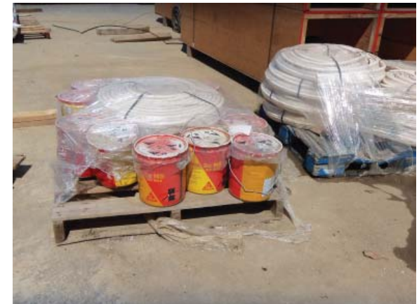
These materials are covered but require a secondary containment facility for storage.
