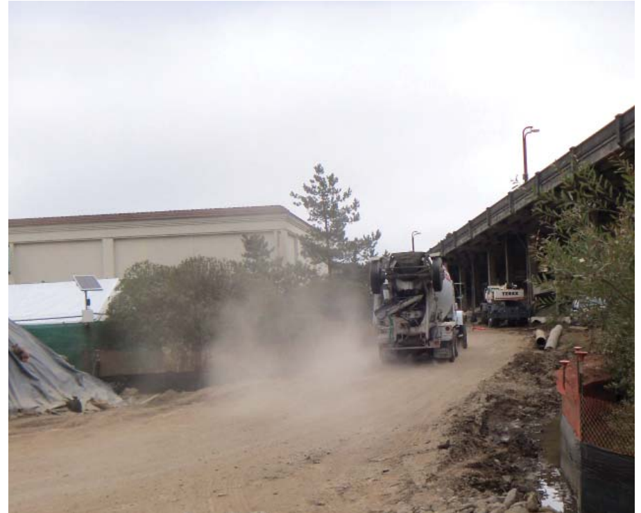
This site requires waterspraying or a soil stabilizer to minimize dust.
