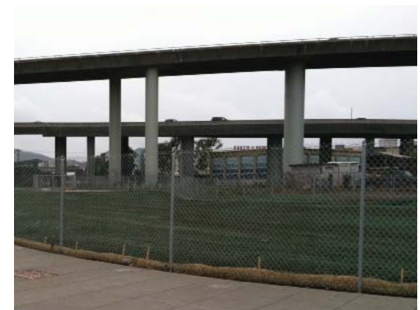
A hydraulic mulch with binder is applied to disturbed soil areas.
