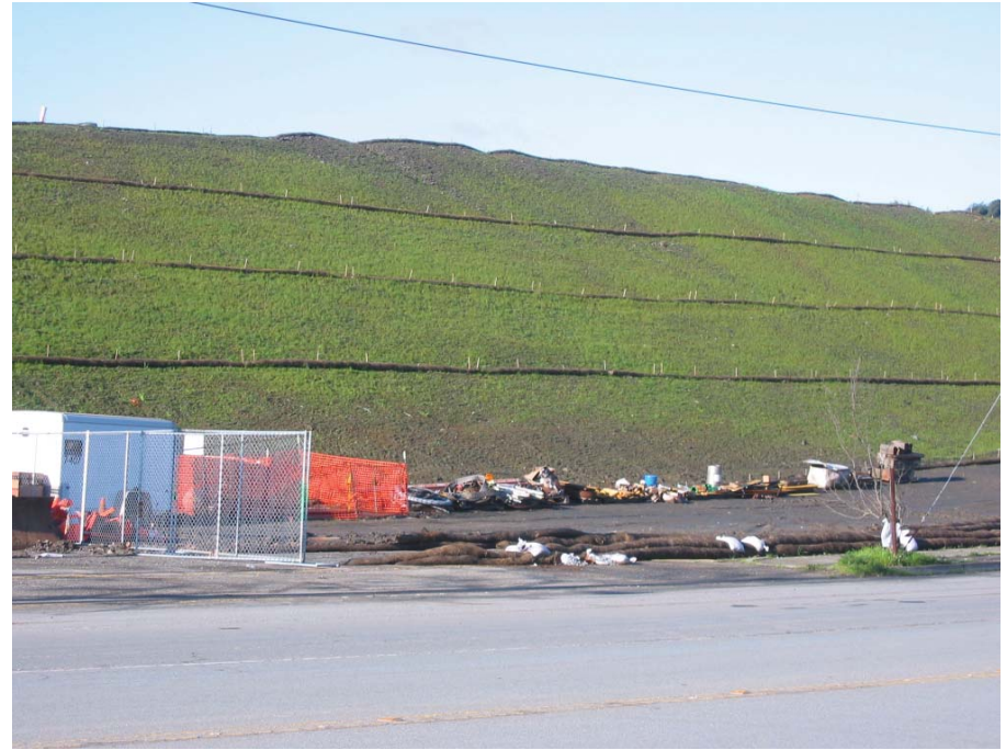
Disturbed soils on the hillside were stabilized with vegetative growth and fiber rolls.
