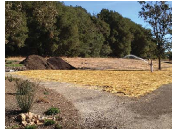
Water is applied to exposed soil and stockpiles to prevent dust generation.
