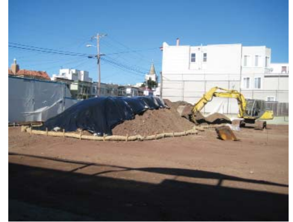
Fiber rolls are properly installed around a stockpile.
