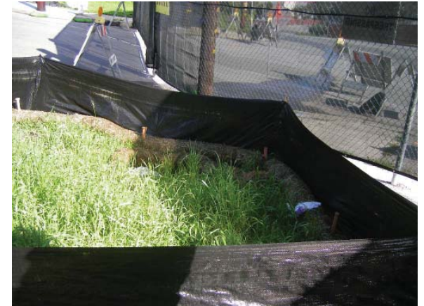
Existing vegetation is protected with fiber rolls and silt fence.
