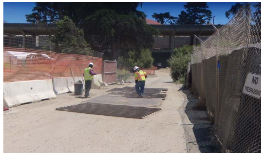
Workers are cleaning the access area to allow the BMP to function effectively.
