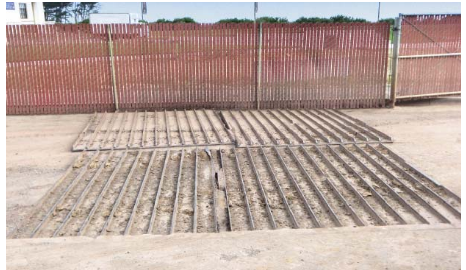
Maintenance is required on this dirt and debris filled construction access.
