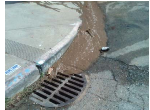
Untreated runoff from an upstream construction site is being discharged to the City storm system.
