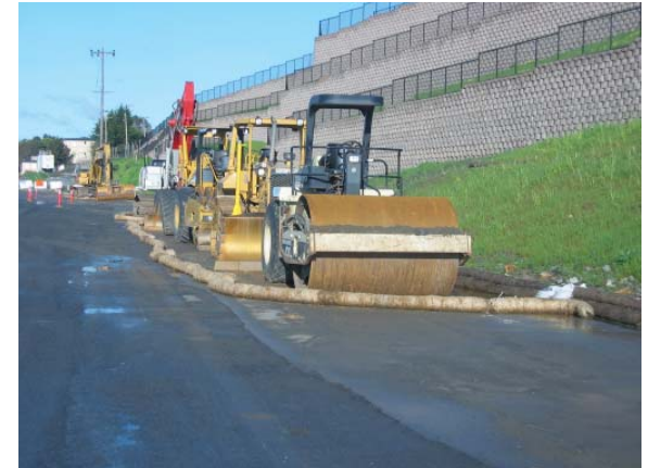
Inactive paving equipment is properly stored with perimeter protection.
