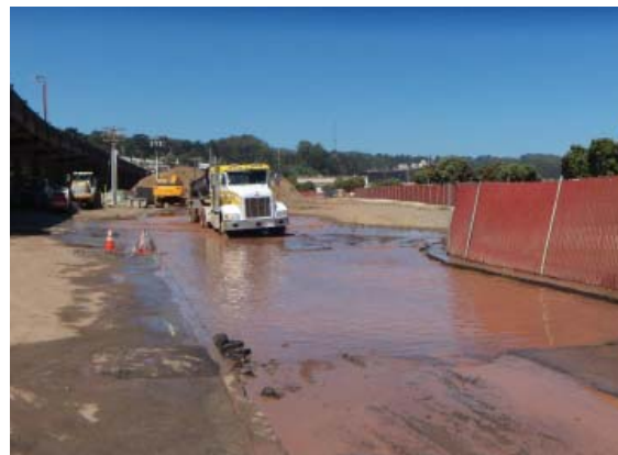
Construction area without a tire wash.
