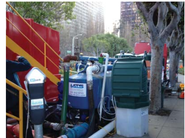
Active treatment system being used at a sewer replacement project in downtown San Francisco
