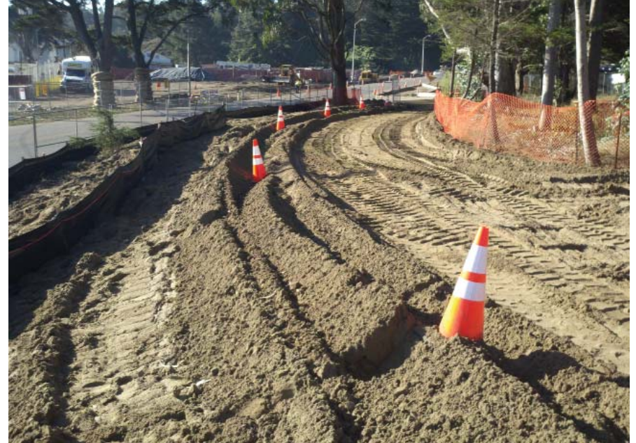
Soil roughening was used on this construction area to prepare for vegetative establishment.
