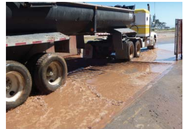
Effects of tire wash removal.
