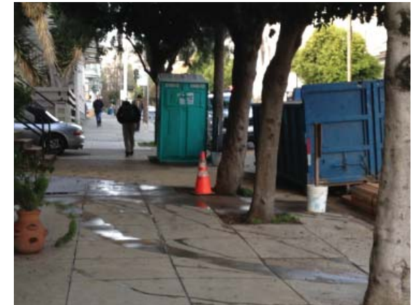
Drilling fluids from a small residence project are leaving the site untreated.
