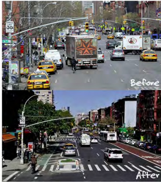
First Avenue Improvements, New York City
