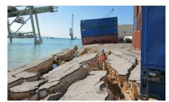
Liquefaction induced lateral spreading at Port de Port-au-Prince
