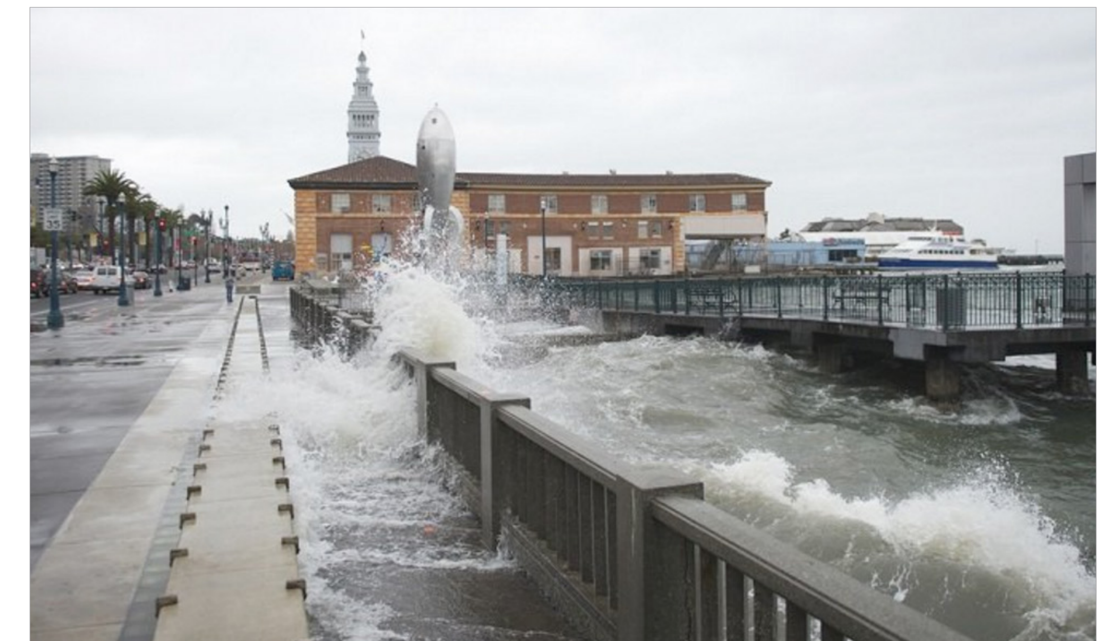
Today, San Francisco's Waterfront is subject to flooding.
