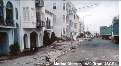
Liquefaction: ground shaking can cause the ground to lose strength and stiffness, causing severe damage to structures, pavements, and utilities.
