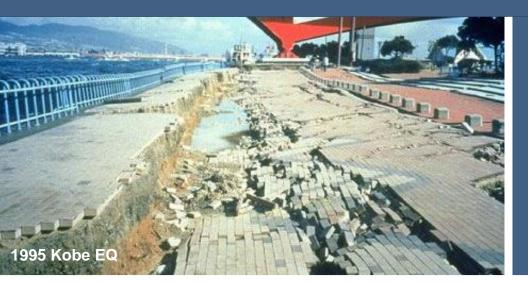
Lateral Spreading: when soils liquefy, they can permanently slide downslope, crack, and settle.
